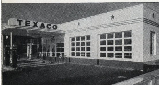
SUPER-Harbord panels applied with invisible joints on this series of stations.—Seattle.
