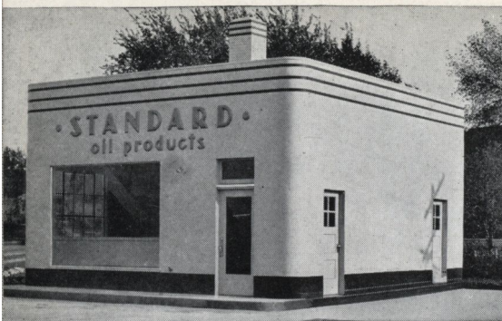
SUPER-Harbord panels applied flush on this oil station.—Des Moines.
