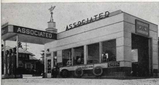
SUPER-Harbord panels with accented lines on this service station.—Bremerton, Wash.
