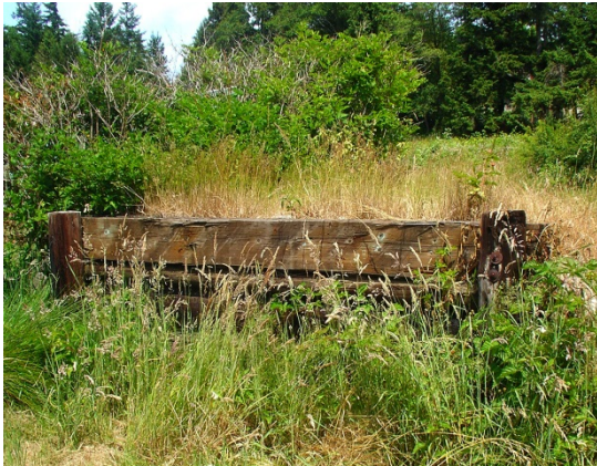
Fig. 16a. Suyematsu loading dock.
