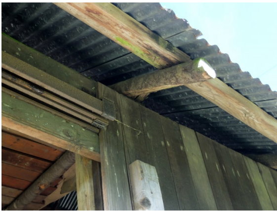
Fig.9d. Pole rafters and corrugated roof.
