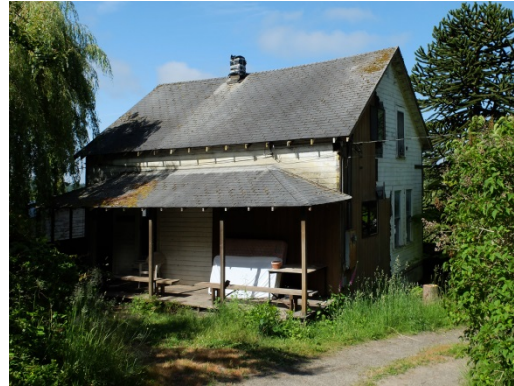
Fig. 8b. NW elevation with mixed siding.
