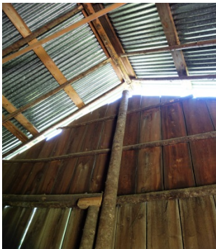
Fig.9a. Gap at ridge.
