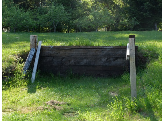
Fig. 16b. Manzanita loading dock.
