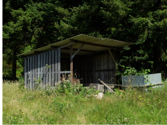
Fig. 26. SW elevation. No.26.
