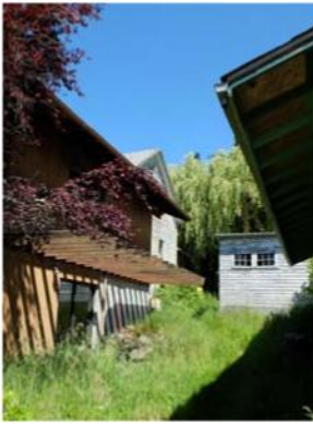
South elevation of house
