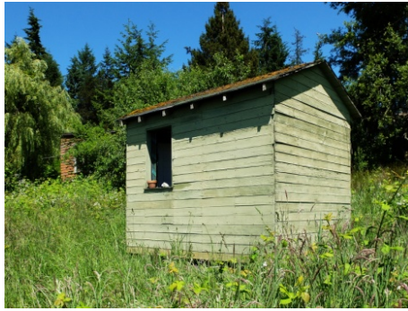
Southwest elevation of shower shed
