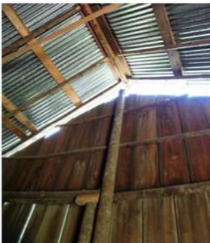
Wall & ceiling of barn
