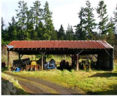
West elevation of Shed 2
