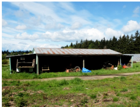
West elevation of Shed 1
