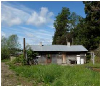
East elevation of bunkhouse
