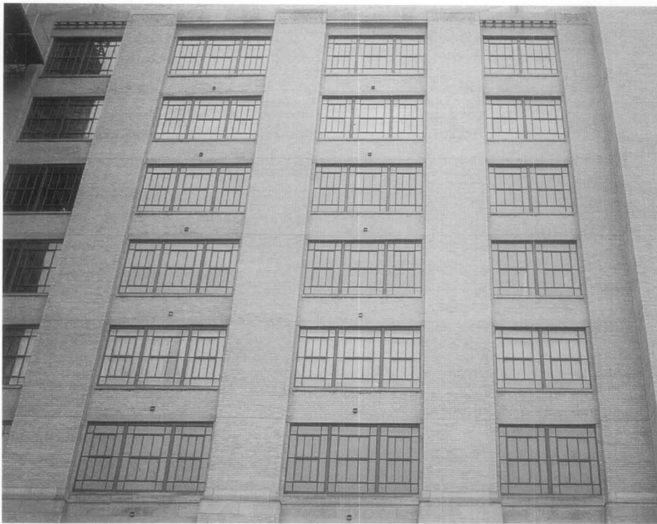
Figure 10. The replacement windows designed for the Sears building rehabilitation met energy efficiency and aesthetic goals while providing for the continued historic appearance of the structure. Photo: Bruner/Cott & Assoc., Inc.
