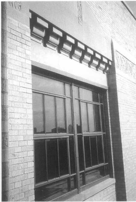
Figure 7. Installed replacement window. Photo: Bruner/Cott & Assoc., Inc.
