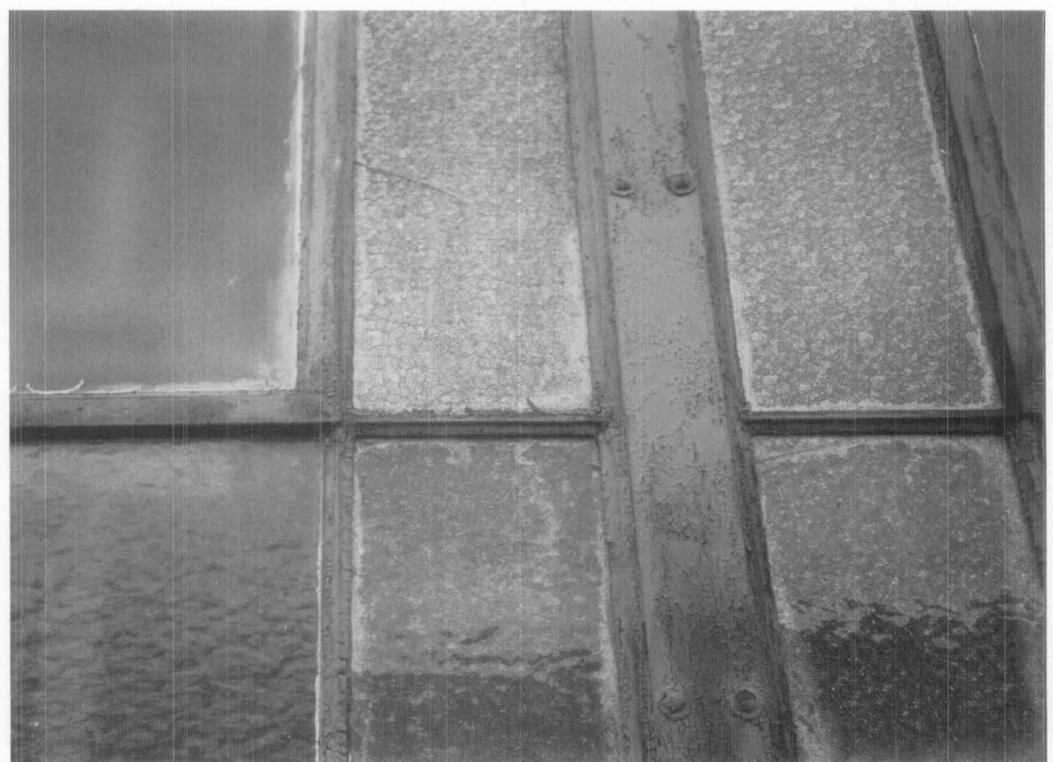
Figure 2. Narrow sightlines, ventilator weathering flanges and mullion boltheads were all distinguishing features of the original steel windows. Photo: Bruner/Cott & Assoc., Inc.
