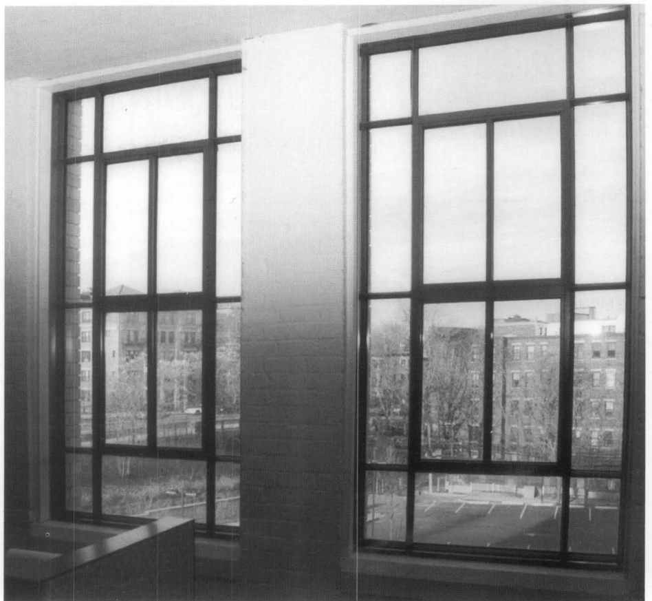
Figure 9. The interior profiles of the original windows were accurately reproduced in the aluminum replacement units. Photo: Bruner/Cott & Assoc., Inc.
