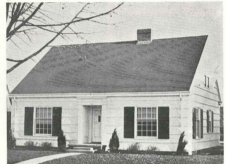
PLAN No. 6463 Size 34'-0" x 30'-0" — Area 1043 sq. ft. The Cape Cod Cottage takes advantage of all enclosed space so that it can be utilized to very best advantage.
