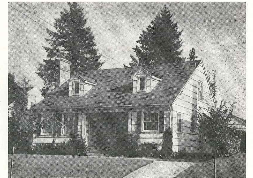
PLAN No. 5226 Size 34'-0" x 34'-6" — Area 1146 sq. ft. A very popular floor plan has been roofed in the economical Cape Cod style in this convenient home, with an attic and a full basement.
