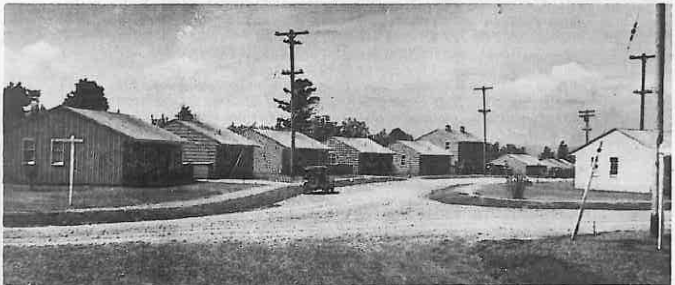
HARNEY HILL HOUSING PROJECT—500 permanent units.
