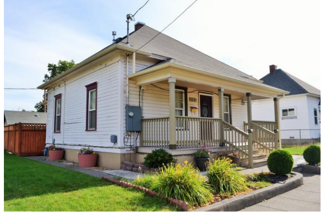
West and south (front) sides. 2015
