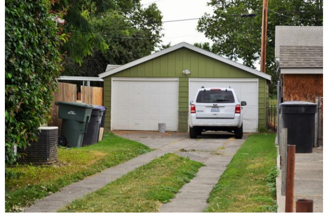
Detached garage, east (front) side. 2015
