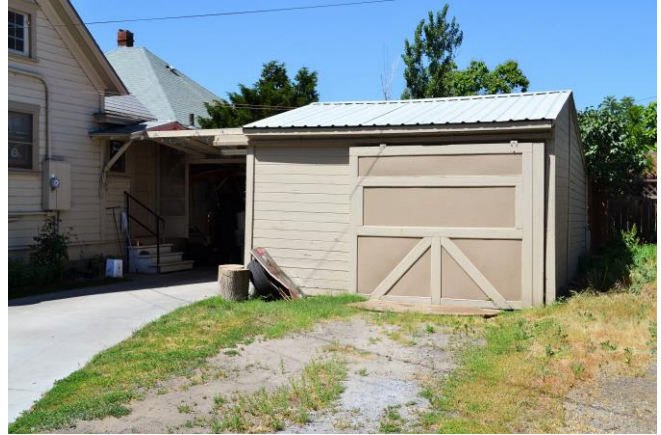
Detached Garage, east (front) and north sides. 2015
