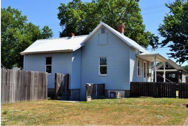
West and south (front) sides. 2015
