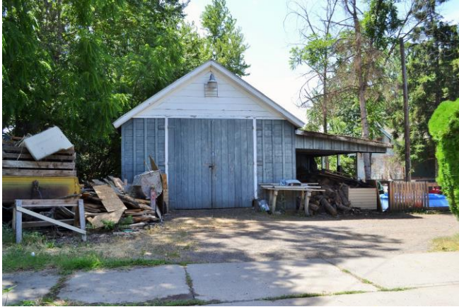
Detached garage, north (front) elevation. 2015
