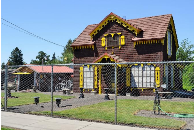
East (front) and north sides; detached garage to left. 2015
