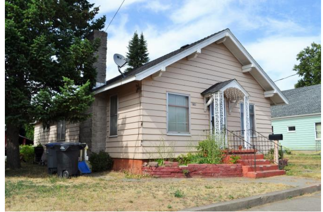
West and south (front) sides. 2015
