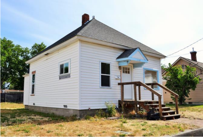
West and south (front) sides. 2015
