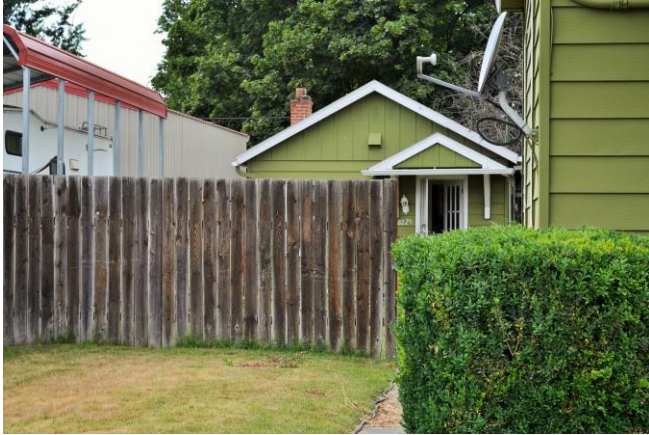
East (front) side; no public access. 2015
