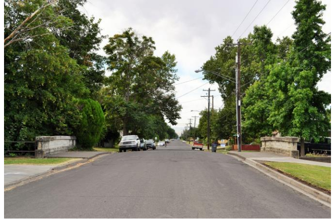
North approach; view to the south. 2015
