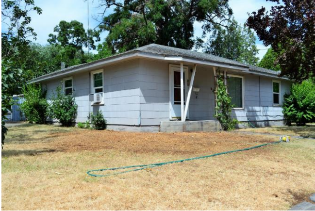
West and south (front) sides. 2015
