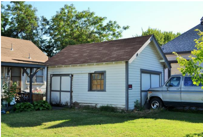
Detached garage, east and north (front) sides. 2015
