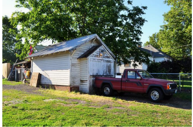
Detached garage, north and west (front) sides; house in background. 2015
