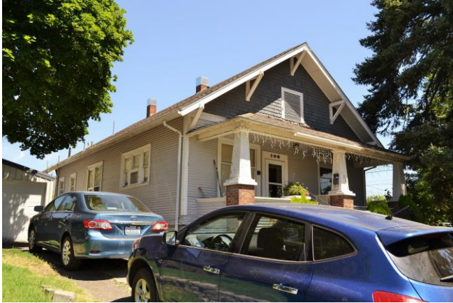
West and south (front) sides. 2015
