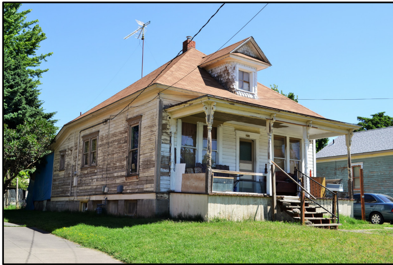
Figure 11. Queen Anne – Spindework style: House at 122 W. Maple St. (Project Number 41), west and south (front) sides.
