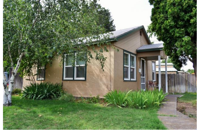
Southwest and southeast (front) sides. 2015
