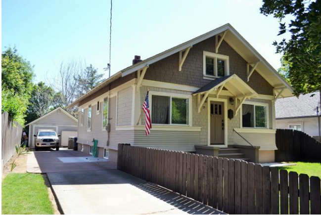
East and north (front) sides; detached garage to rear. 2015
