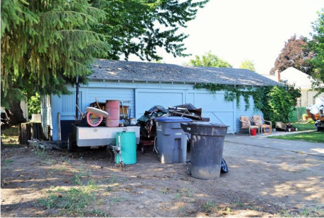
Detached garage, east and north (front) sides. 2015
