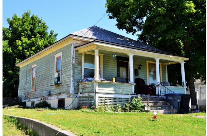
West and south (front) sides. 2015
