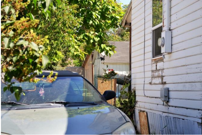
West and south (front) sides, photo center. 2015
