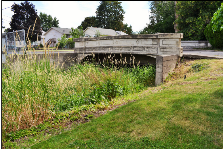
Figure 9. S. 3rd Avenue Bridge (Project Number 120). View to the northeast.
