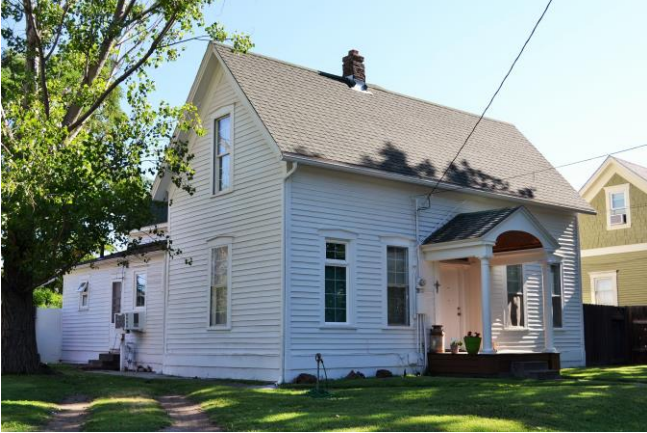
West and south (front) sides. 2015
