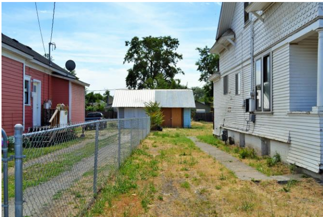
Detached garage, north side, divided between two properties. 2015
