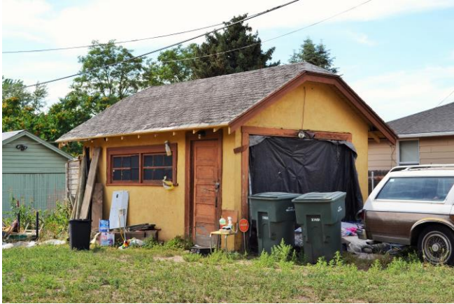
Detached garage, south and east (front) sides. 2015
