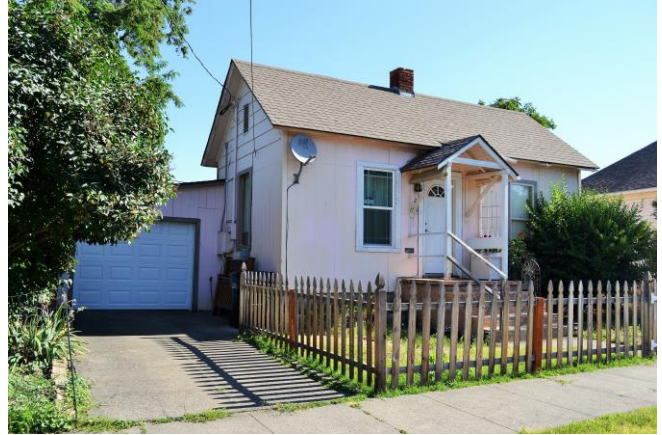
West and south (front) sides. 2015
