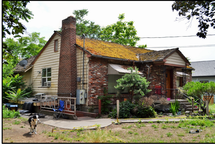
Figure 16. Minimal Traditional style: House at 211 W. Chestnut St. (Project Number 10), east and north (front) sides.
