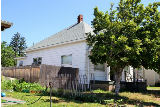
West and south (front) sides. 2015
