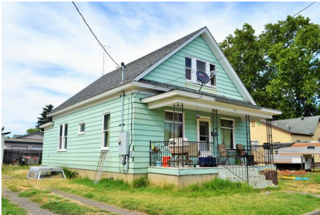
West and south (front) sides. 2015
