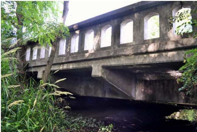
East side of bridge; view to the southwest. 2015
