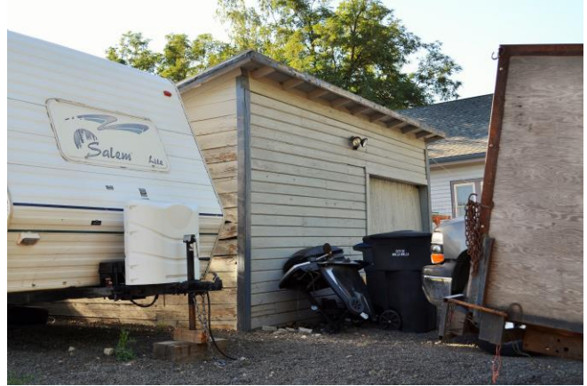
Detached garage, south and east (front) sides. 2015
