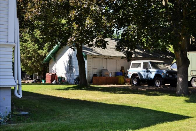
Detached garage, east and north (front) sides. 2015
