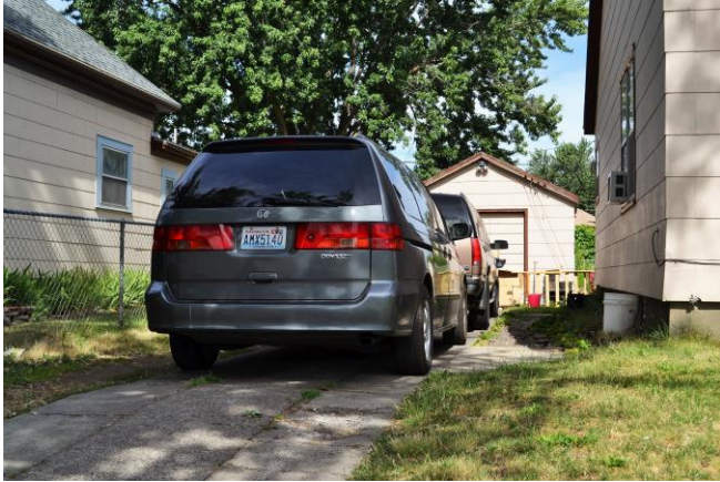
Detached garage, photo center, west (front) side. 2015
