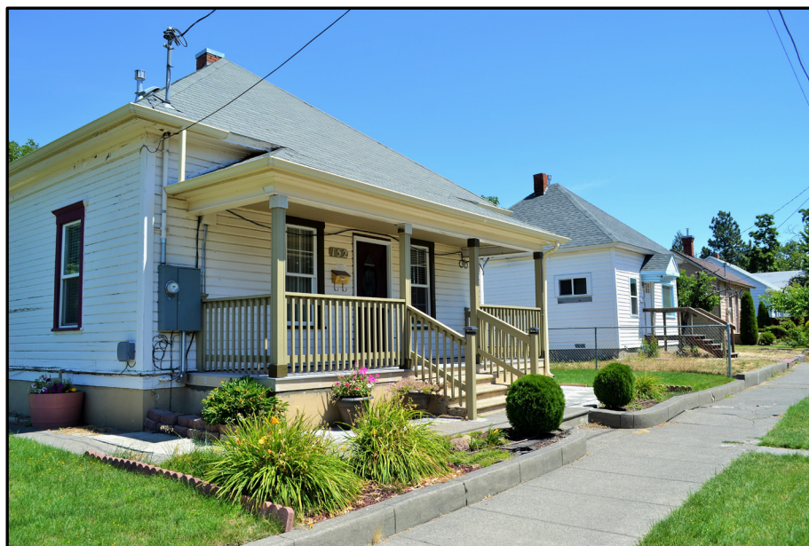
Figure 6. Overview of homes on Malcolm Street just east of S. 4 th Avenue; the building at the left is Project Number 97. View to the northeast.
