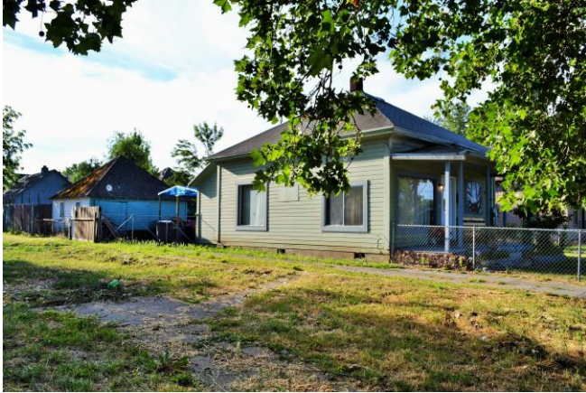
North and west (front) sides; detached garage to rear. 2015
