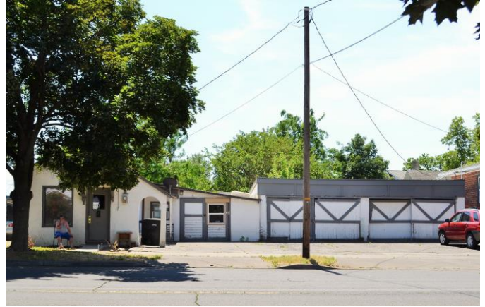
North (front) elevation; garages at right. 2015
