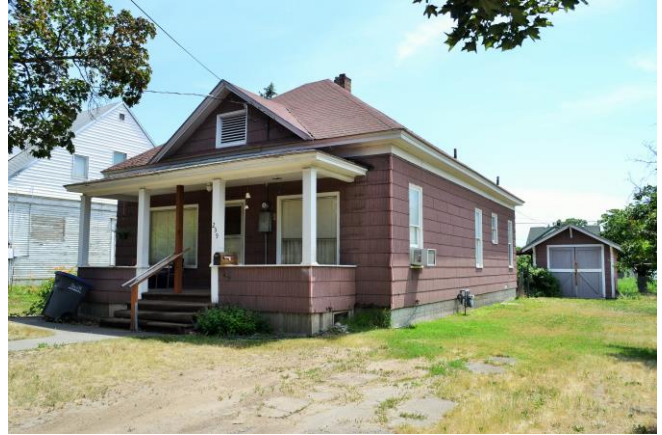
North (front) and west sides; detached garage to rear. 2015
