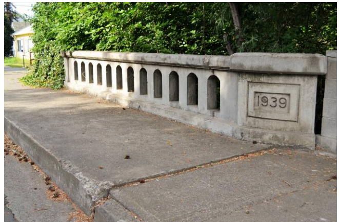
West balustrade; view to the southwest. 2015
