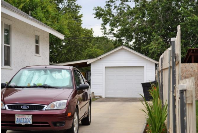
Detached garage, east (front) side. 2015
