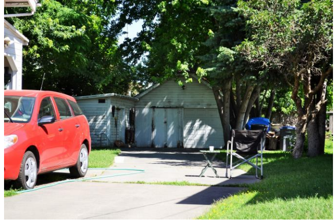
Detached garage at right, south (front) side; shed at left. 2015
