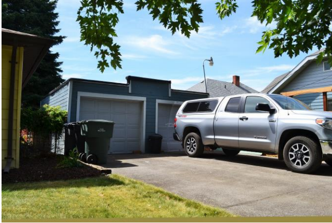
Detached garage, south and east (front) sides; house at right. 2015
