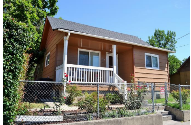
West and south (front) sides. 2015
