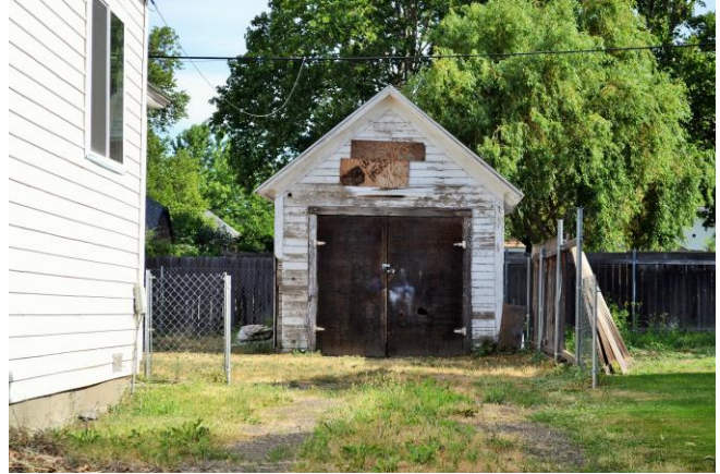
Detached garage, south (front) side. 2015
