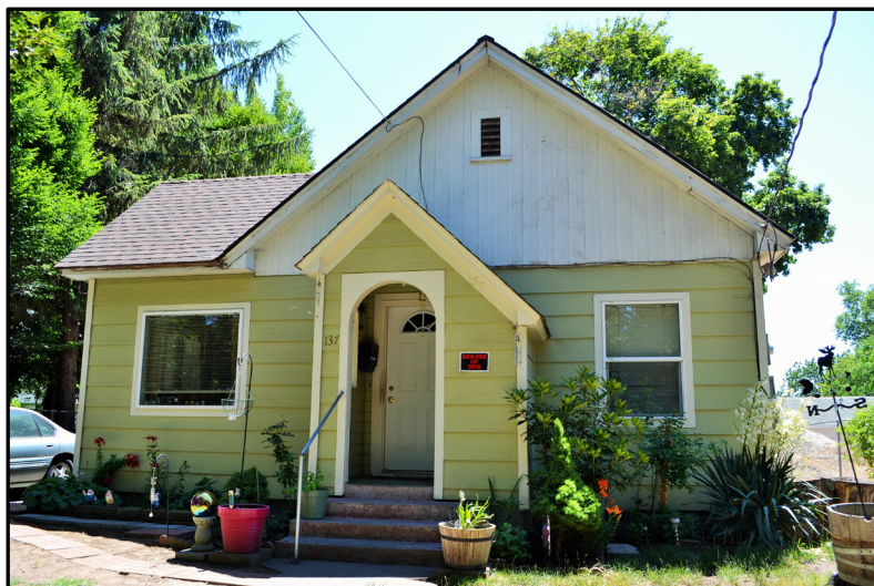
Figure 15. Tudor style: House at 137 W. Chestnut St. (Project Number 27), north side.
