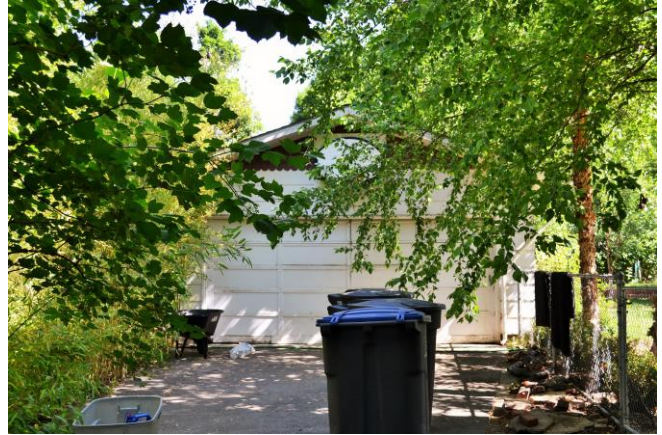
Detached garage, south (front) side. 2015
