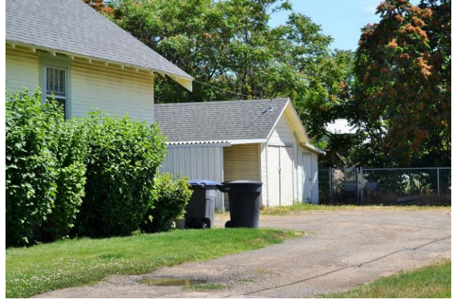
Detached garage, west and south (front) sides; house at left. 2015
