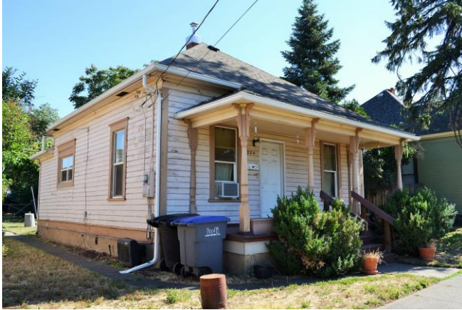
West and south (front) sides. 2015
