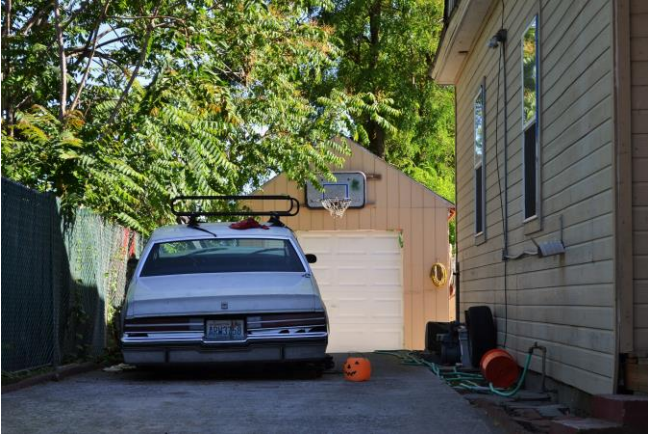
Detached garage, north (front) elevation. 2015
