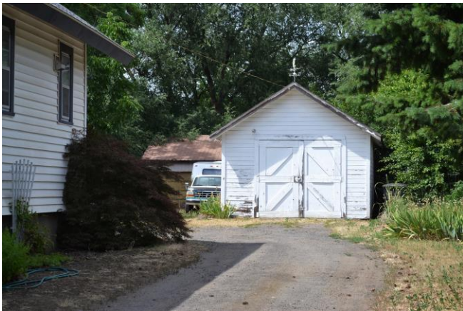
Detached garage, south (front) side. 2015
