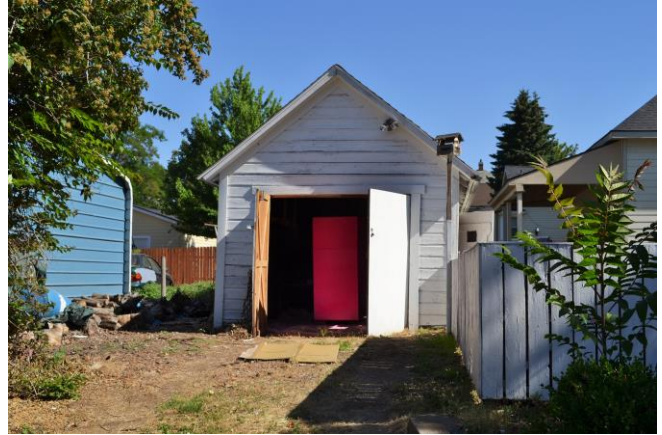
Detached garage, south (front) side. 2015
