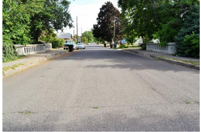
South approach; view to the north. 2015
