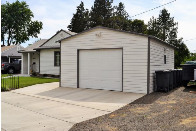
Detached garage, east (front) and north sides; house to rear. 2015
