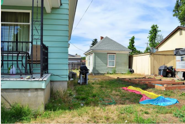
Outbuilding, west (front) and south sides; house left foreground. 2015
