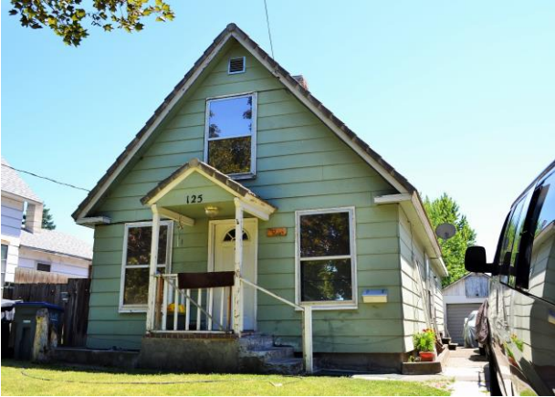
North (front) and west sides; detached garage to rear. 2015
