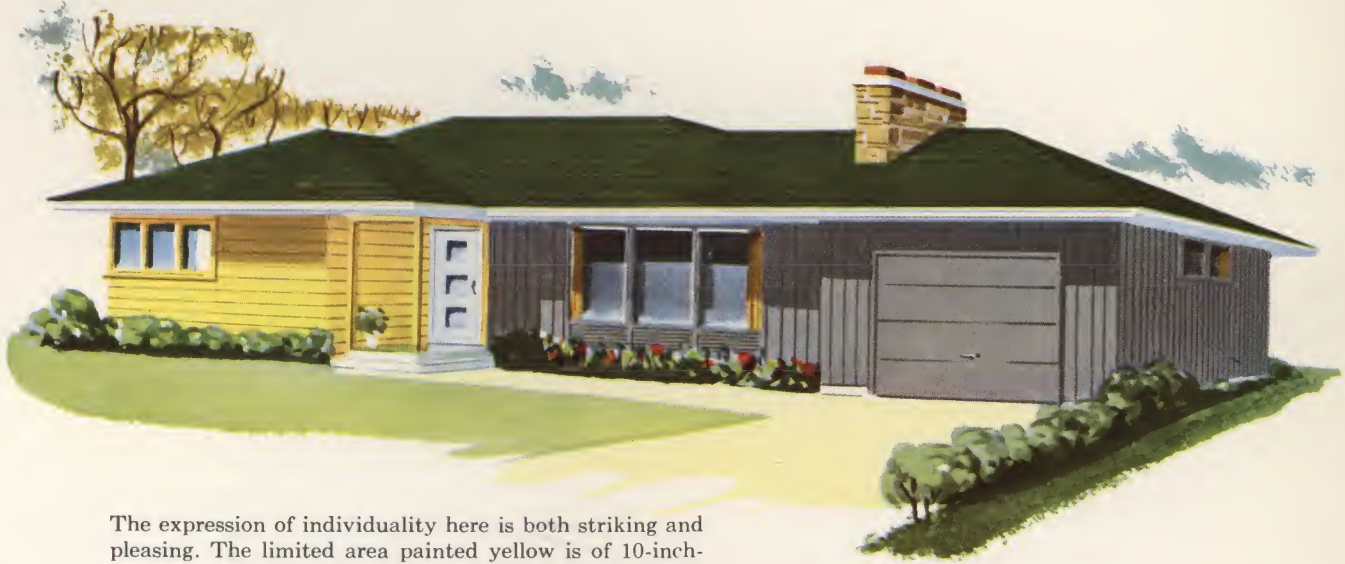
This handsome exterior variation embodies a feature section of deep color and shadow lines derived from wide vertical siding. The remaining walls of the home have 8-inch siding installed horizontally and painted soft green.
