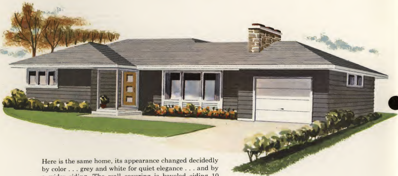
This attractive modern home . . . a rambler or ranch house . . . typifies the design preference of many throughout the nation. Walls of horizontal beveled wood siding 8 inches wide contribute to the pleasing low-and-long appearance.
