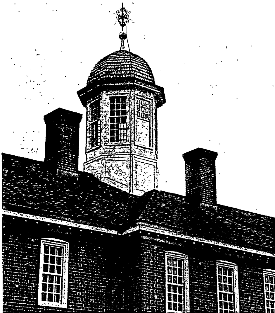
Pressure-impregnated fire-retardant cypress shingles were installed on the reconstructed mental hospital at Colonial Williamsburg. Photo by Rudd M. Long.
