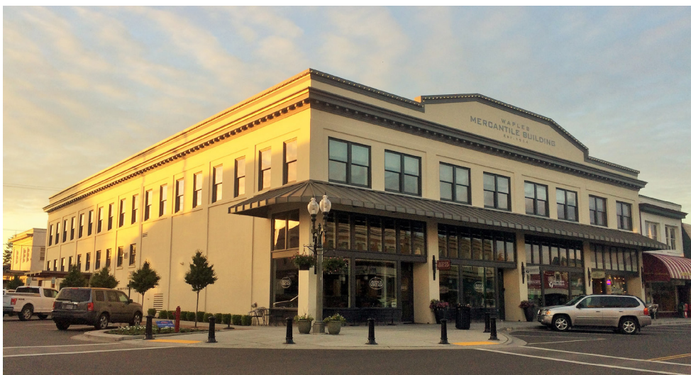
The Waples Building is listed in both the National Register of Historic Places and the Lynden Register of Historic Places. The extensive renovation of the building to convert it into a 35-room inn and a number of retail spaces utilized the Federal Historic Tax Credit and Special Tax Valuation. Courtesy City of Lynden.
