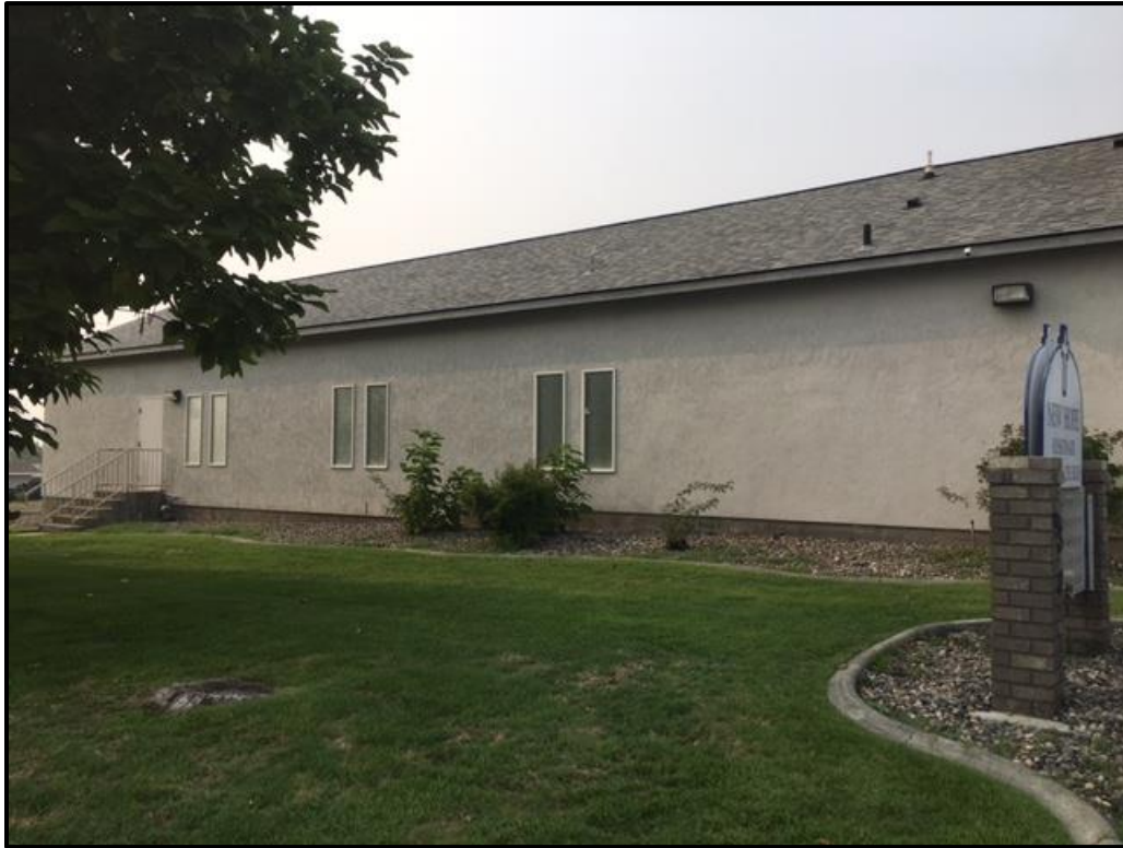
Figure 63. Southern elevation of the New Hope church building, looking west.
