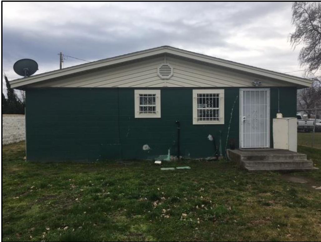
Figure 11. Northern (rear) elevation of the residence at 107 W Sylvester Avenue.
