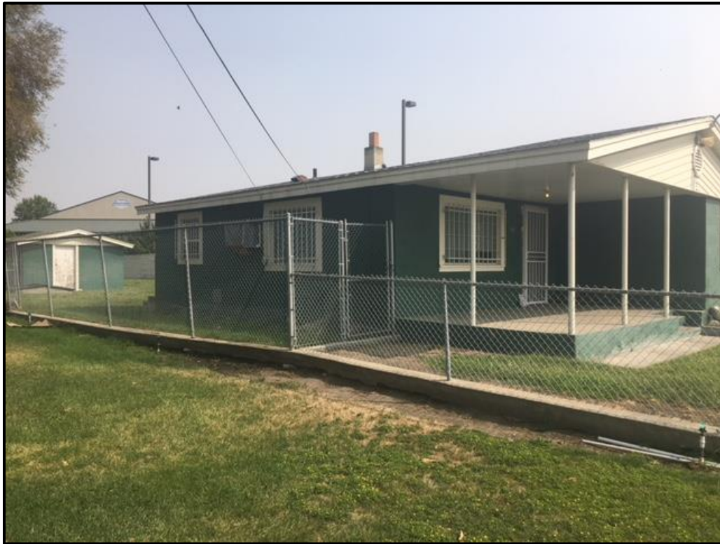
Figure 10. Western elevation and southwestern corner of the residence at 107 W Sylvester Avenue.
