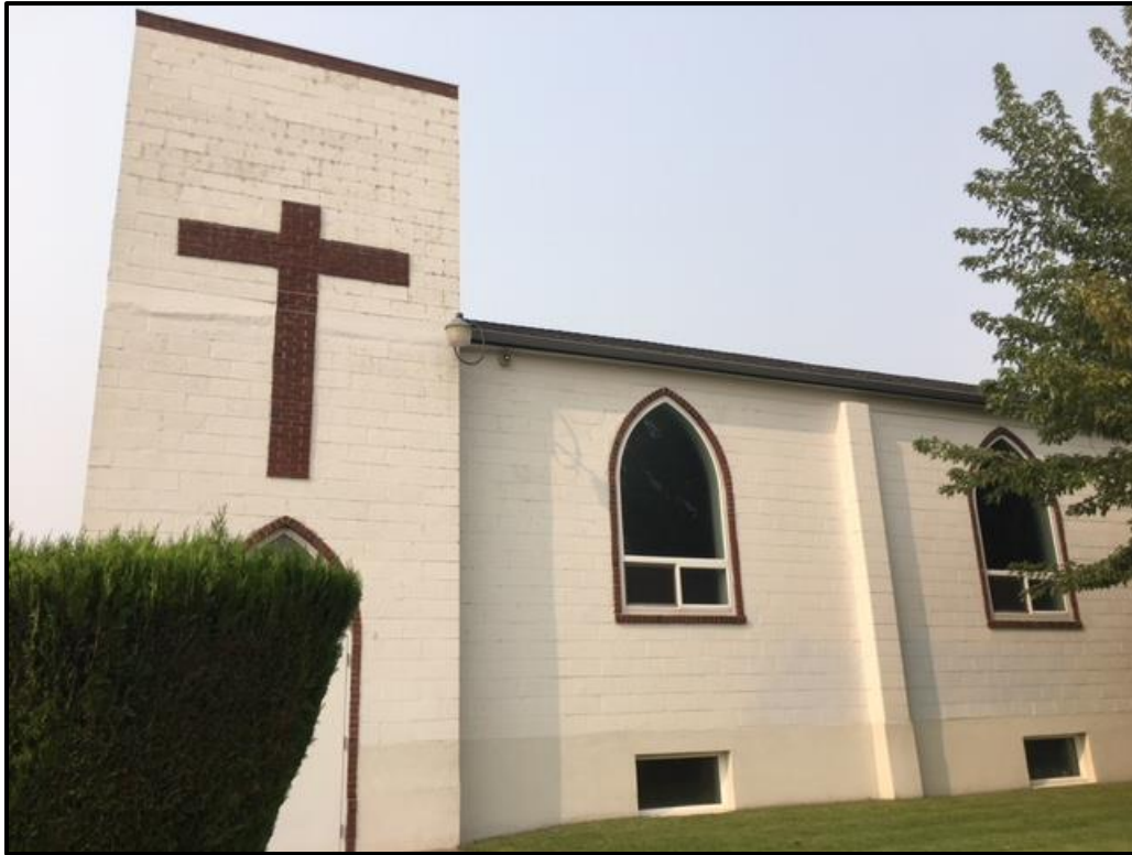
Figure 50. Southern elevation of the church, entryway on left.
