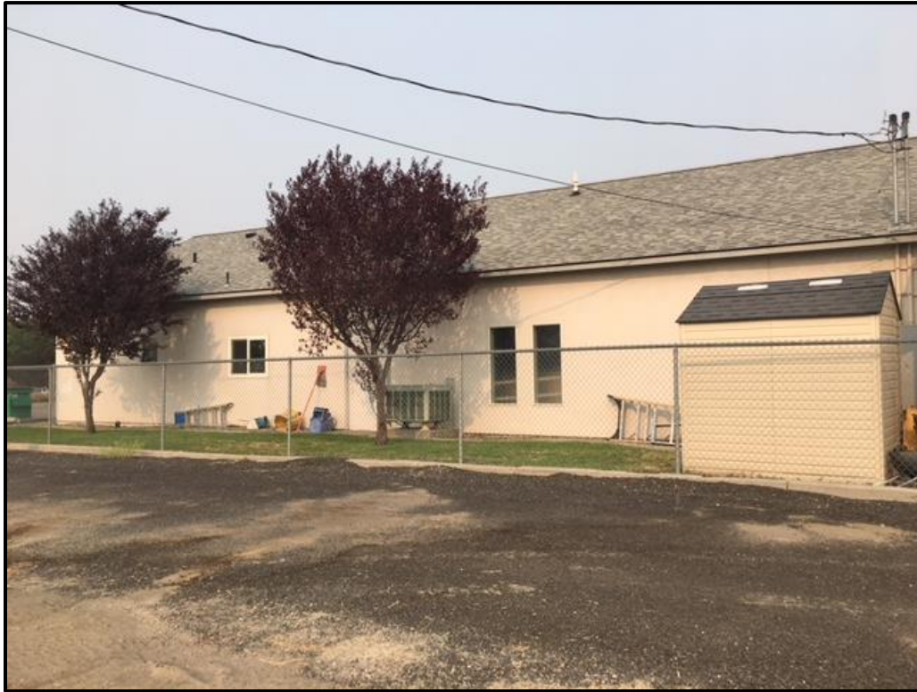
Figure 66. Western elevation of the New Hope church building.
