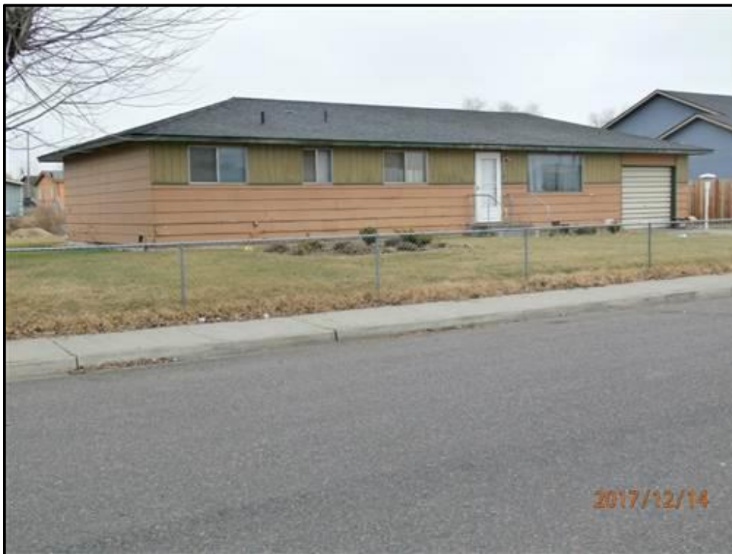
Figure 22. Western (front) elevation of 705 S Douglas Avenue.
