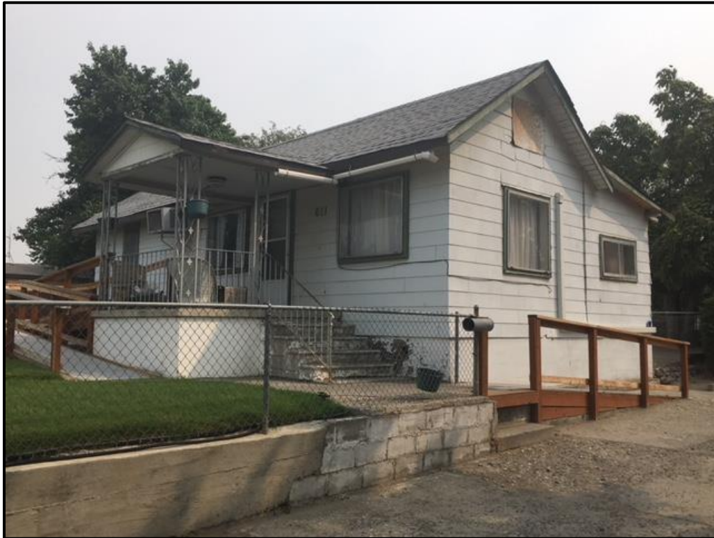
Figure 16. Southwestern corner of residence at 611 S Beech Avenue.
