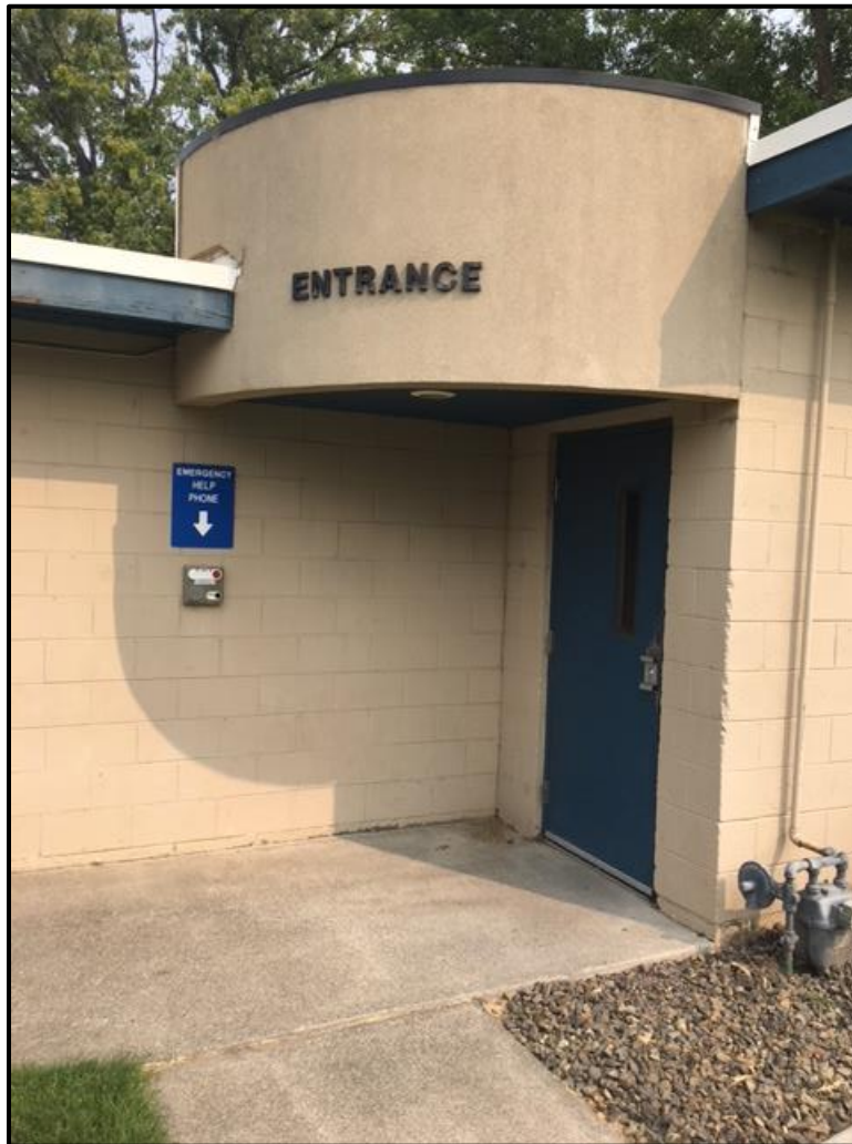
Figure 82. Main entry on the western elevation of the Kurtzman Park Mini Station.
