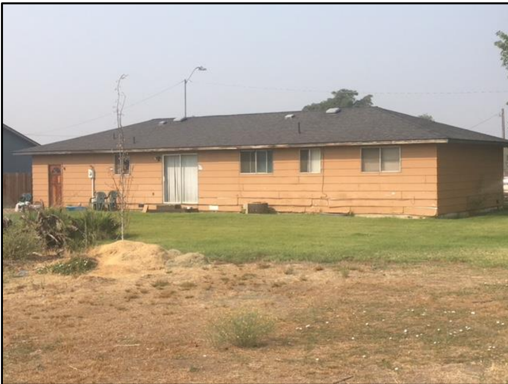
Figure 25. Eastern (rear) elevation of the residence.
