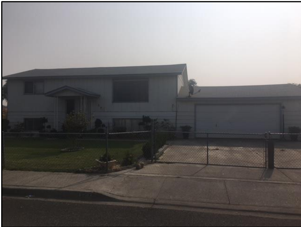
Figure 28. Eastern (front) elevation of residence at 727 S Douglas Avenue.
