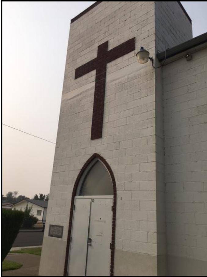
Figure 52. Entrance on southern elevation of the church.
