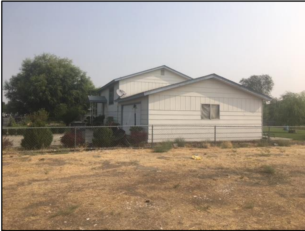
Figure 30. Southern elevation of 727 S Douglas Avenue.
