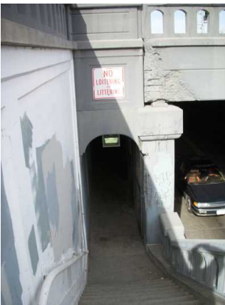
one of the pedestrian underpass stairwells, facing east.
