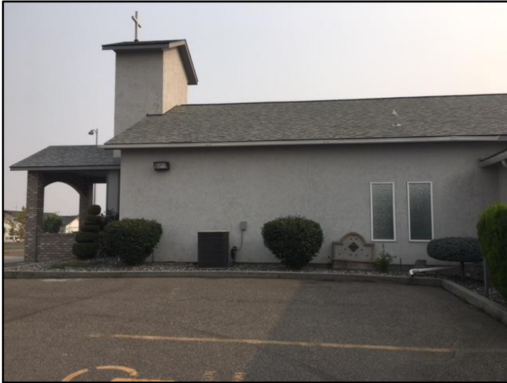
Figure 69. Northern elevation of the main entryway vestibule.
