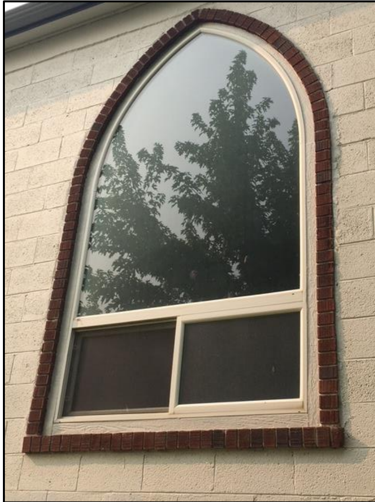
Figure 49. Detail of the windows on the southern elevation of the church.
