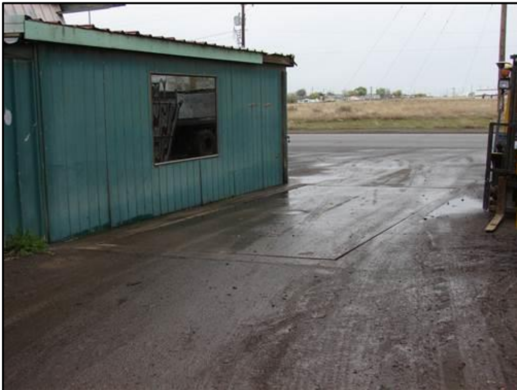
Figure 74. Southern elevation of the utility building at the Tommy's Steel and Salvage complex, looking east.
