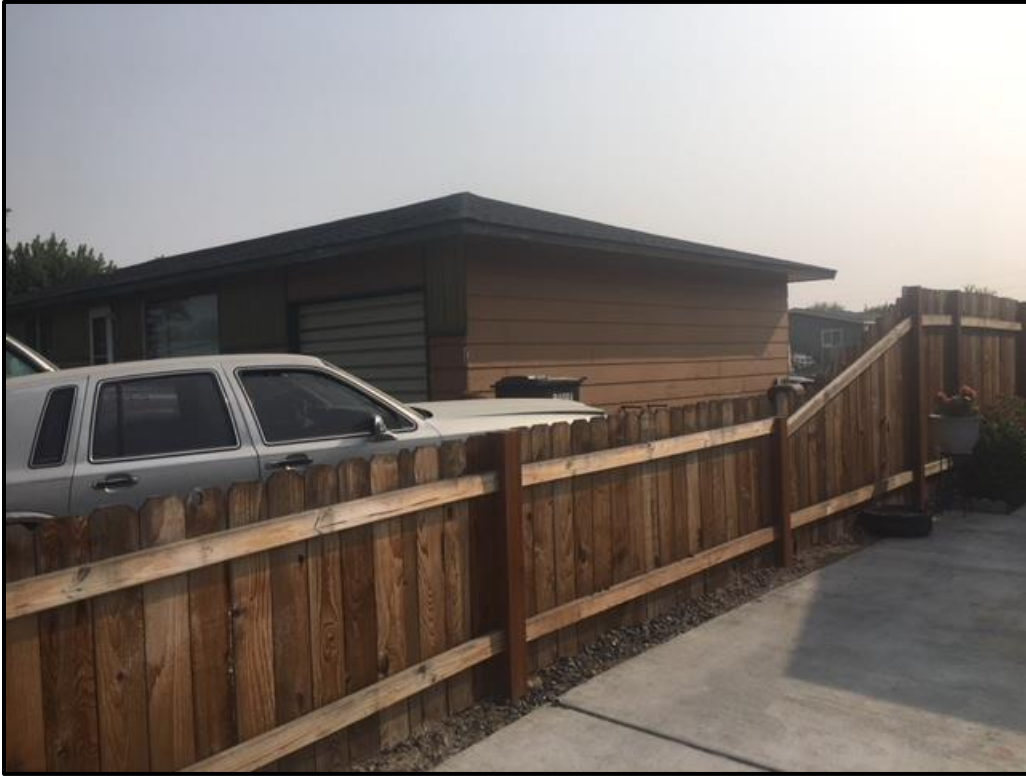
Figure 24. Southern elevation of the residence.
