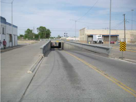
the Lewis Street Railroad Underpass from its west end, facing east.
