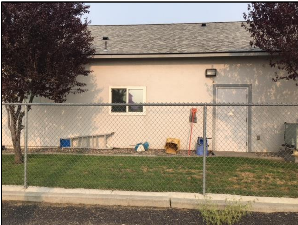
Figure 67. Western elevation of the New Hope church building.
