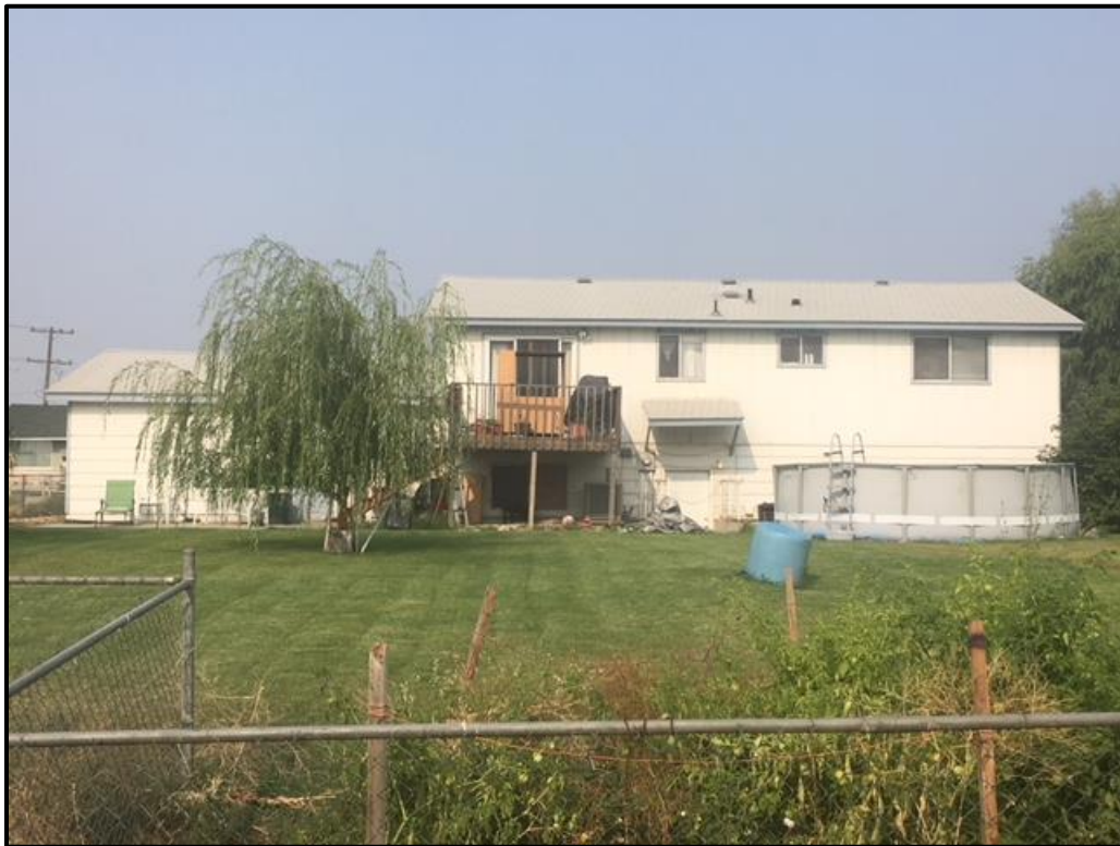
Figure 31. Eastern (rear) elevation of 727 S Douglas Avenue.
