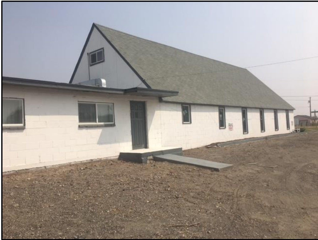
Figure 39. Overview of the southern elevation of the church building.
