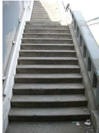
a pedestrian stairwell in the underpass, facing east.
