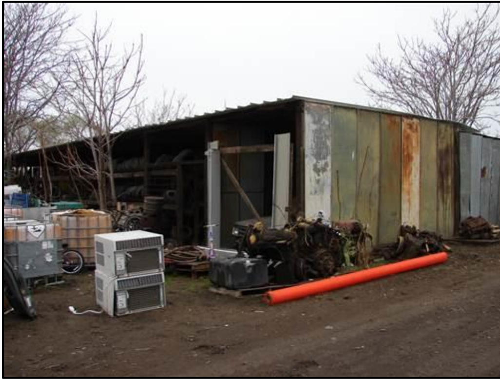
Figure 78. Eastern and southern elevations of implement shed.
