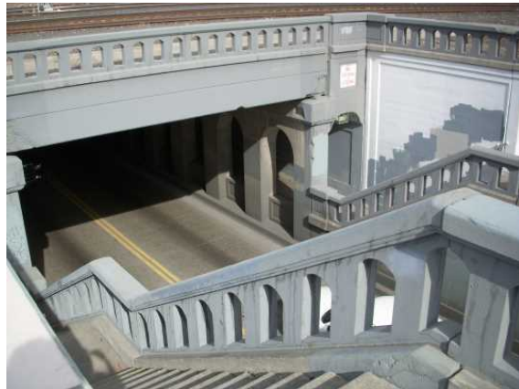
the pedestrian underpass stairwell facing southeast.
