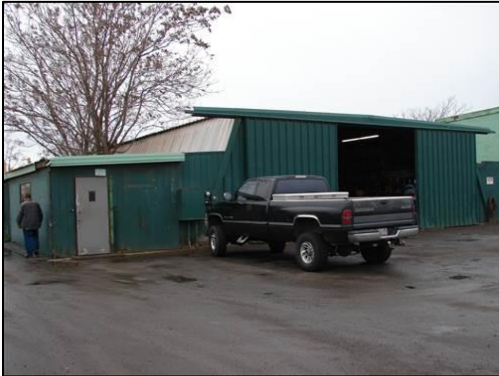
Figure 73. Eastern elevation of the utility building at the Tommy's Steel and Salvage complex.
