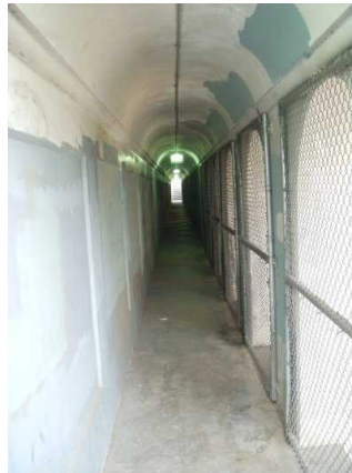
the arched pedestrian underpass facing east.
