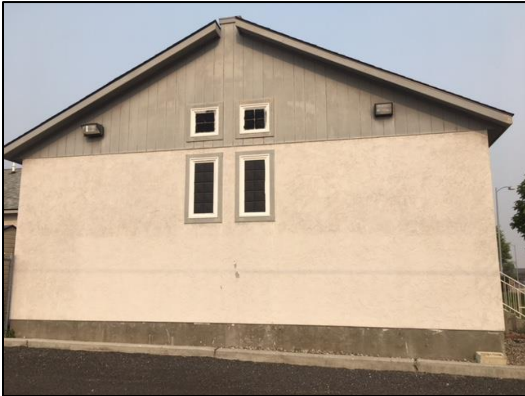
Figure 65. Southern facet of the western elevation.
