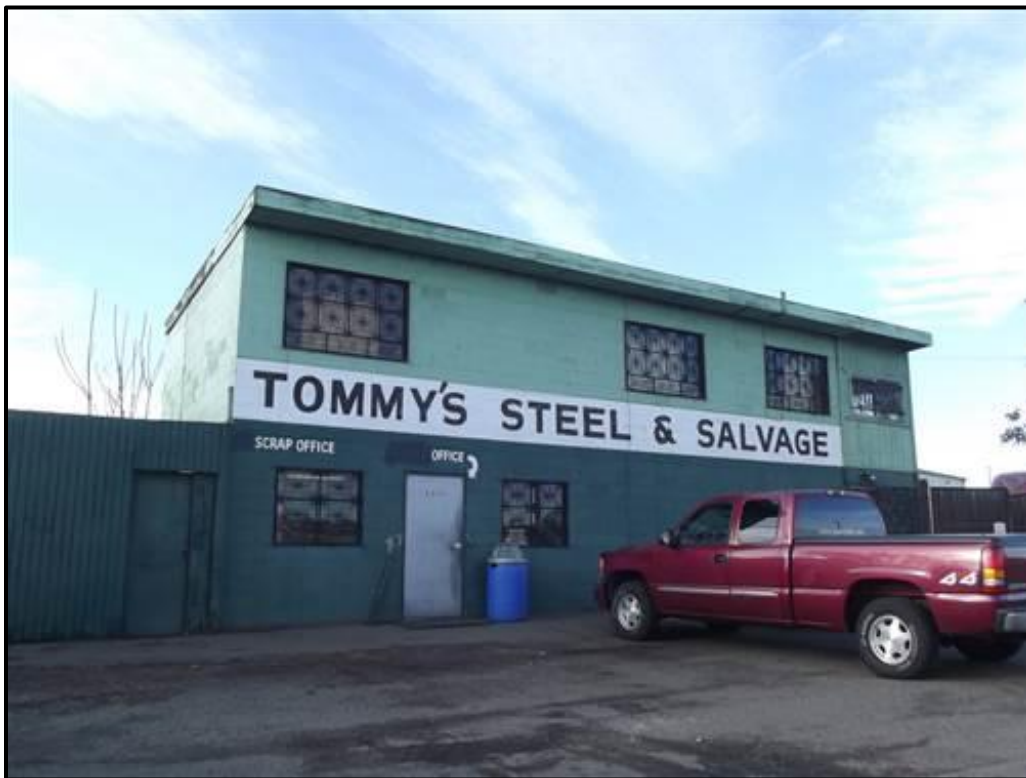
Figure 75. Eastern elevation of the mixed commercial and residential building, looking west.
