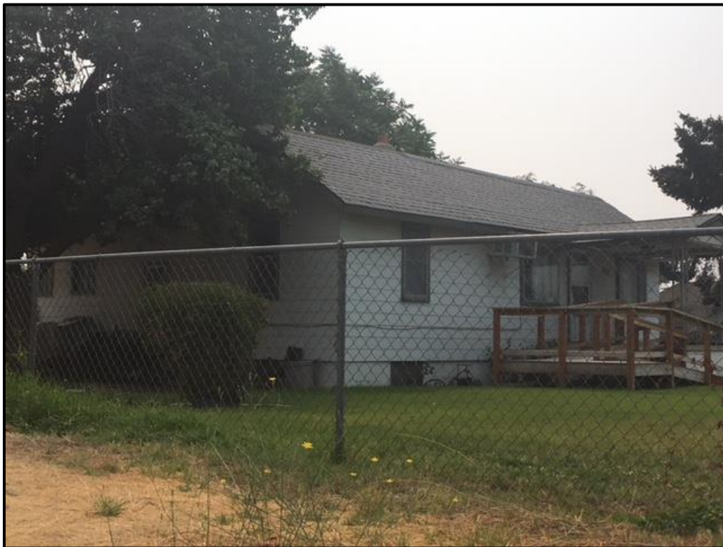
Figure 17. Northwest corner of the residence.
