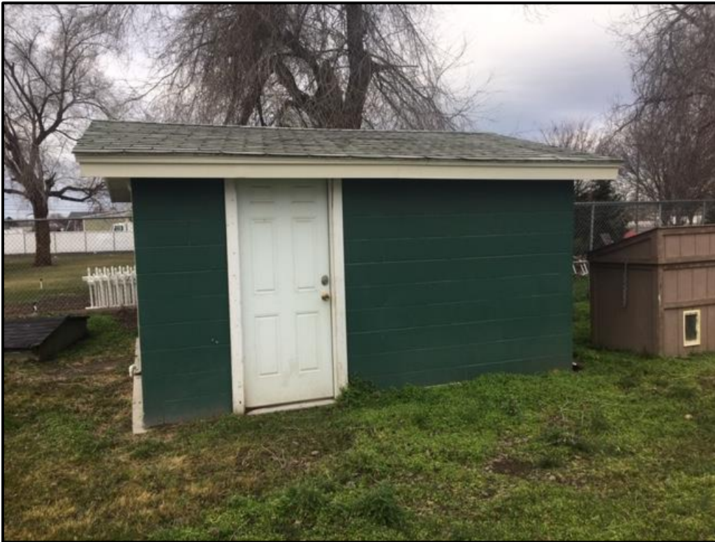
Figure 13. Outbuilding in the backyard of the residence at 107 W Sylvester Avenue.
