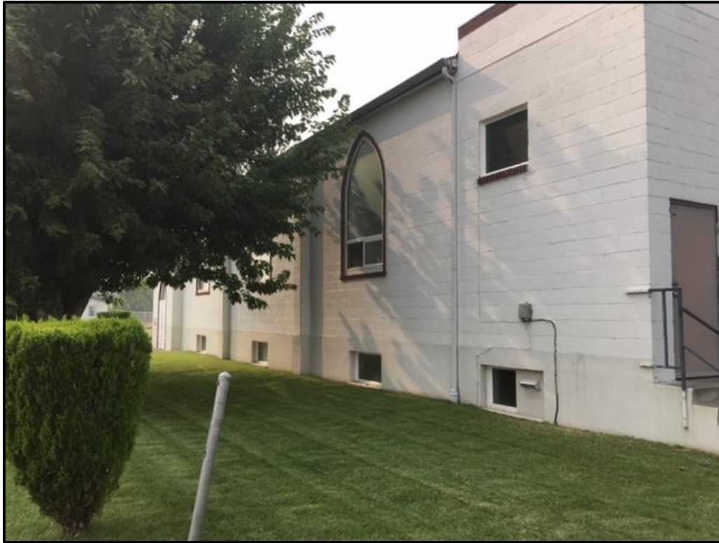
Figure 55. Southern elevation and southeastern corner of the church.
