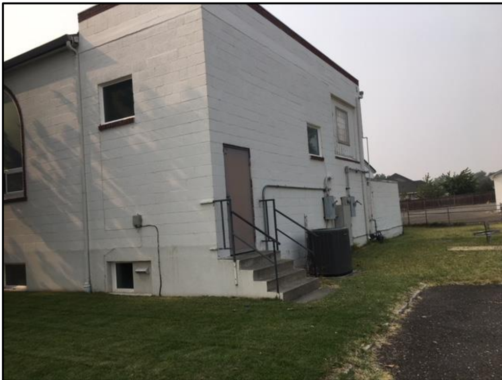
Figure 56. Southeastern corner, southern and eastern elevations of the church.
