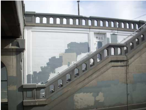
a pedestrian stairwell and utilities access door facing north.
