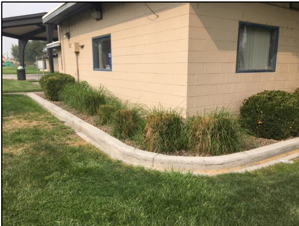
Figure 84. Southwest corner of the Kurtzman Park Mini Station.
