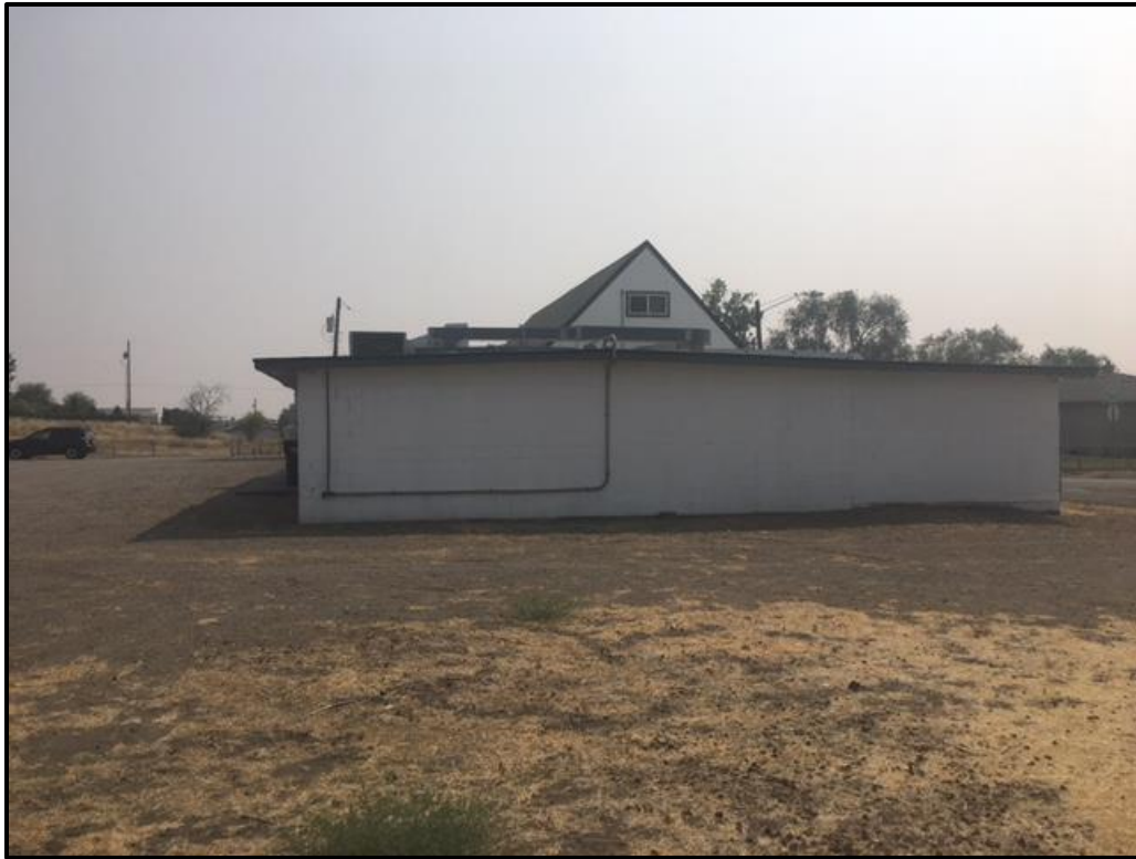
Figure 42. Western elevation of the church building.
