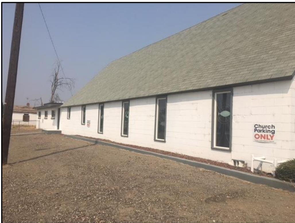
Figure 40. Detail of the southern elevation, showing the stained-glass windows.
