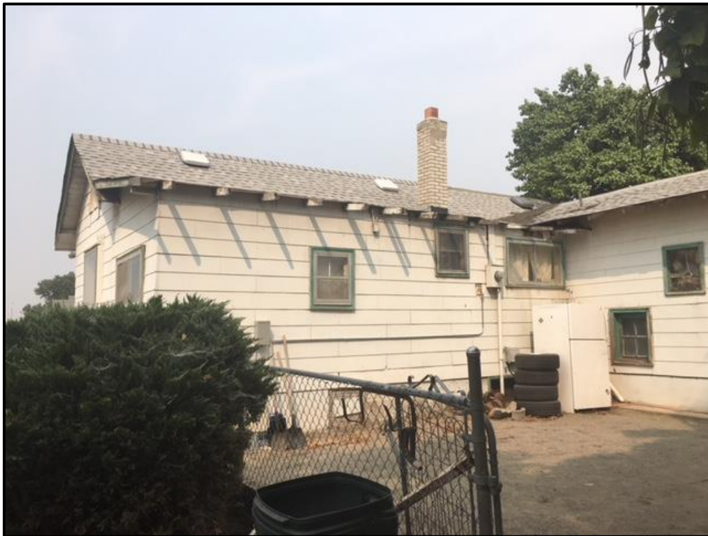
Figure 19. Eastern elevation (rear) of residence at 611 S Beech Avenue.
