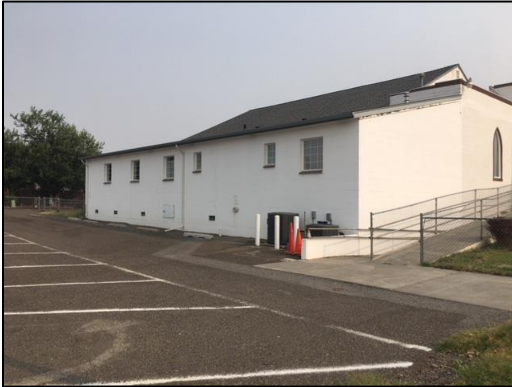
Figure 58. Northern elevation of church building.
