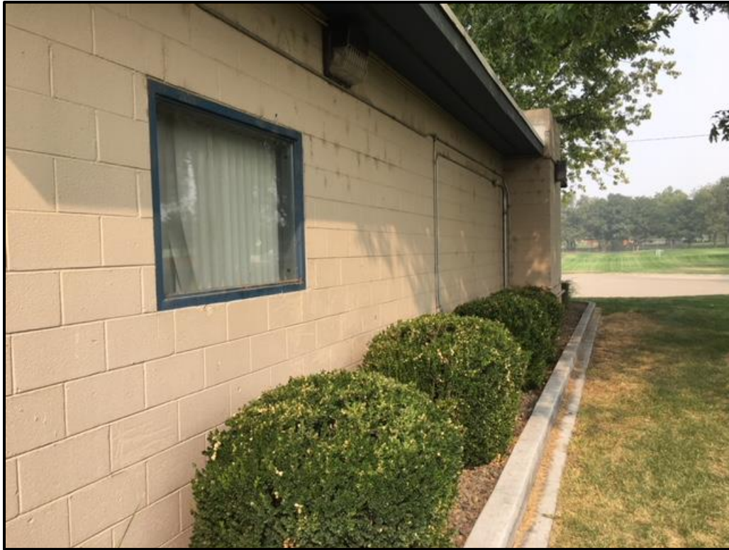
Figure 83. Western elevation of the Kurtzman Park Mini Station.
