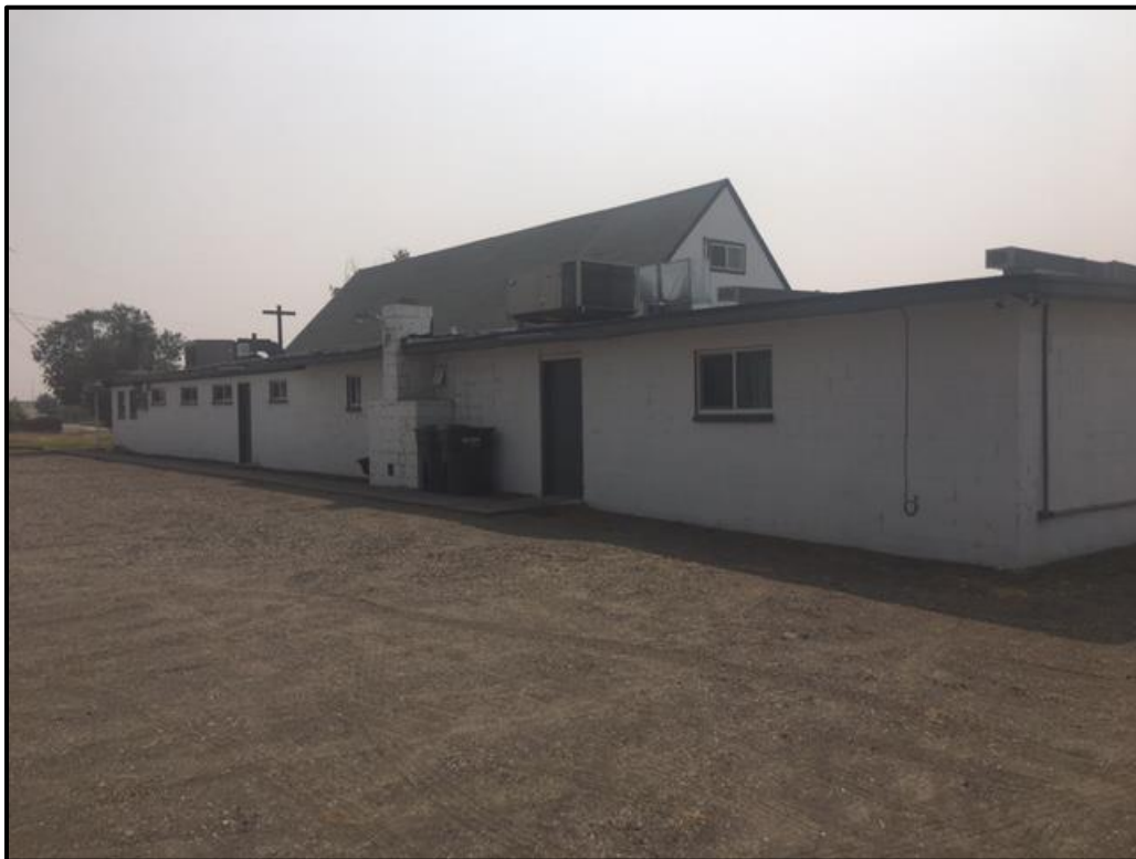
Figure 43. Northern elevation of the church building.
