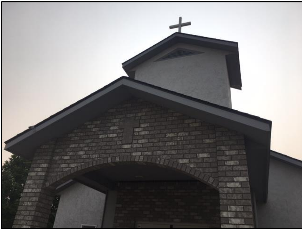
Figure 62. Detail of the covered entryway at the southeastern corner of the building.
