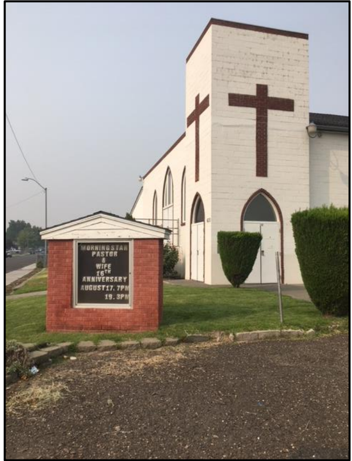
Figure 53. Southwestern corner, and entryway of church, with announcement board, looking north along S. Douglas Avenue.
