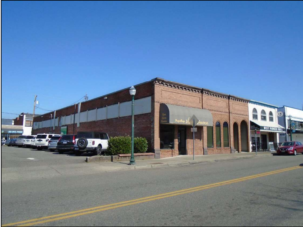
Photograph 3. Setting of the building, facing northeast (Stantec 2023).
