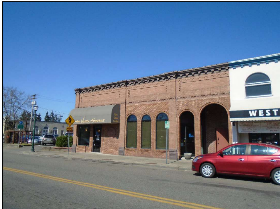
Photograph 2. Primary façade of the building, facing northwest (Stantec 2023).
