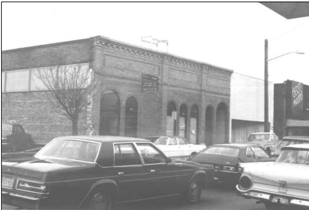
Photograph 6. The primary façade of the building in 1982, facing northeast (Gallacci 1982).
