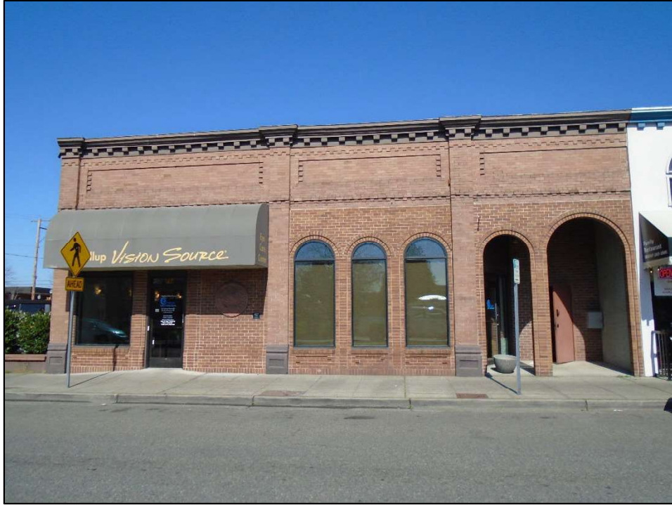
Photograph 1. South-facing primary façade of the building, facing north (Stantec 2023).
