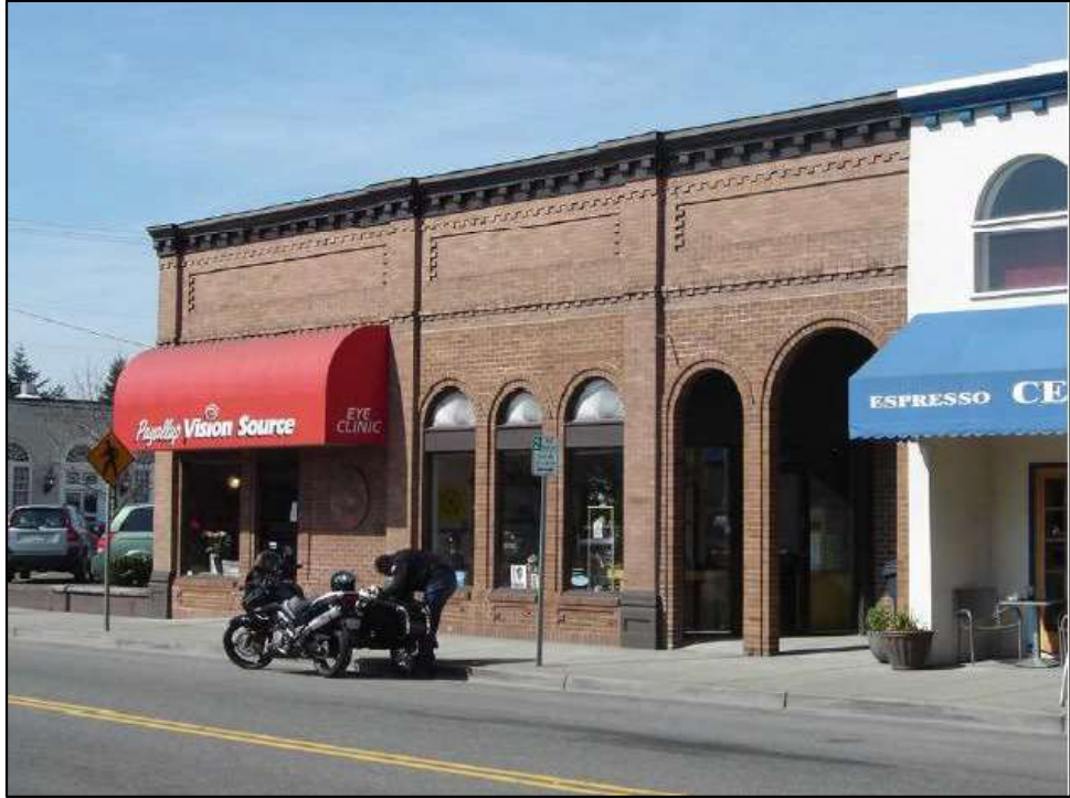
Photograph 7. The primary façade of the building in 2007, facing northwest (Fűrész 2007).
