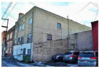
East (rear) of building, right center of photograph, 2017. Note scar on adjacent building, suggesting an addition has been removed.
