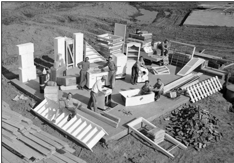
Left, a view of the materials used by the Levitt Brothers Company in constructing a typical Levittown house (Levittown Historical Society).
