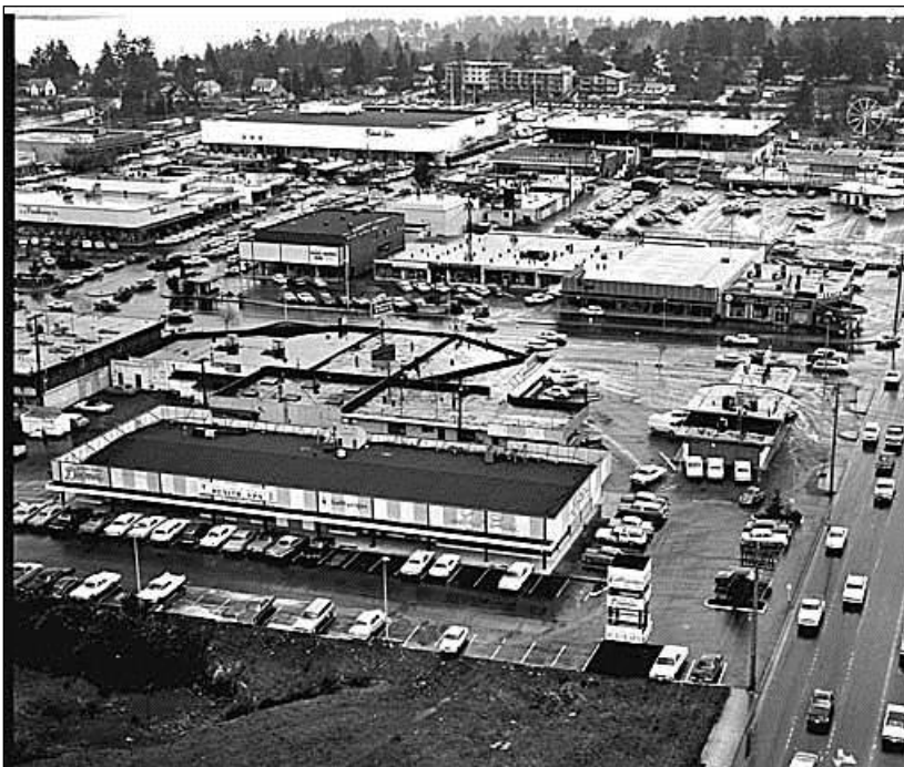
As the suburbs grew, so did the auto-oriented retail development that served the residents. Below, a view of NE 8 th Street and 104 th Avenue NE in downtown Bellevue in 1967 (MOHAI, Image 1986.5.1000.1).
