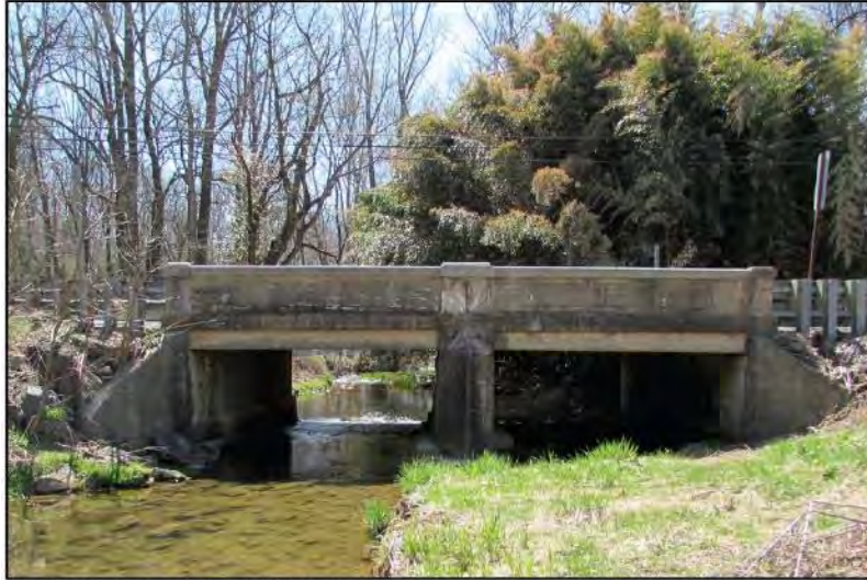
FIGURE I-15: Kirks Mill Bridge, 2015 (Courtesy of PWKP 2018c)
