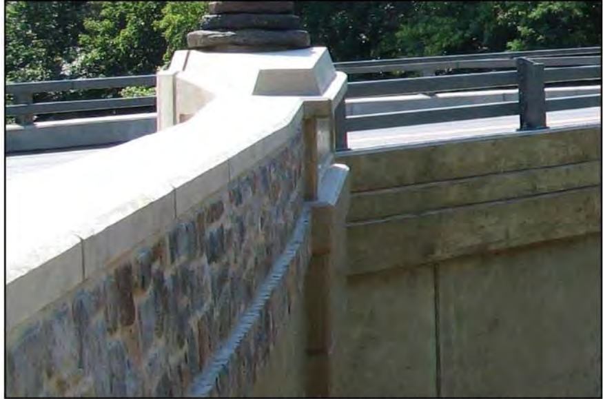
FIGURE I-49: Successful Application of Texture onto Bridge Face and Real Stone Masonry Abutments, River Road Bridge, PA (Photographer: Monica Harrower, Pennsylvania DOT; Courtesy of Harrower 2019)
