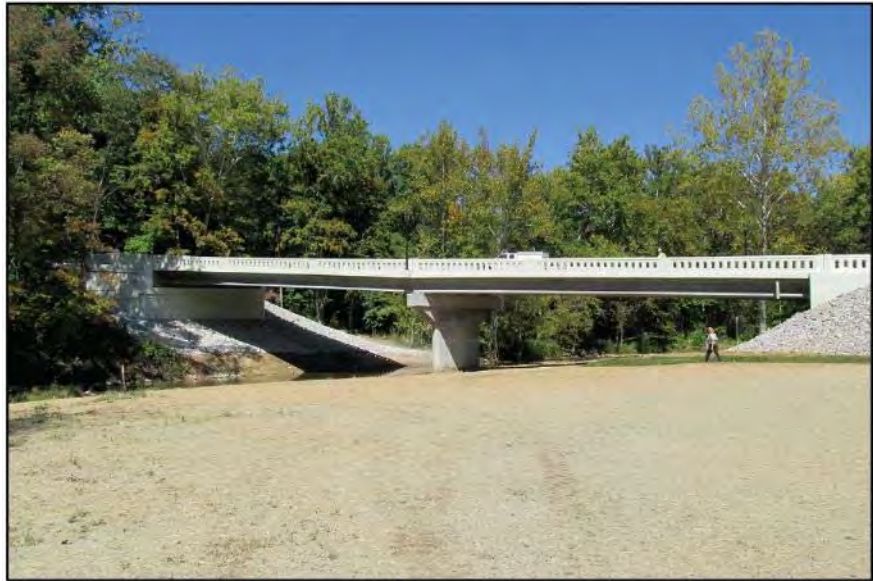
FIGURE I-28: Stinesville Road Bridge, 2014 (Courtesy of BLN 2019b)
