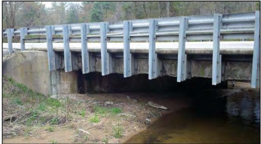
FIGURE I-17: Carlisle Road Bridge, 2018 (Courtesy of PWKP 2018b)
