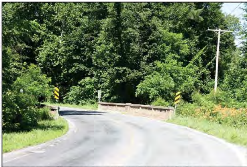
FIGURE I-1: Gardners Bridge over Bermudian Creek before Replacement, 2015 (Courtesy of Amisson 2016)
