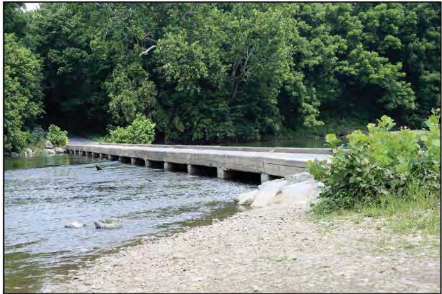
FIGURE I-42: Morgan's Ford Bridge, 2015 (Photographer: Trevor Wrayton, Virginia DOT)
