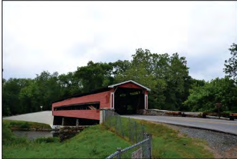
FIGURE I-24: Smith's Bridge, June 2011 (Photographer: Jodi Christman; Courtesy of Bridgehunter.com)
