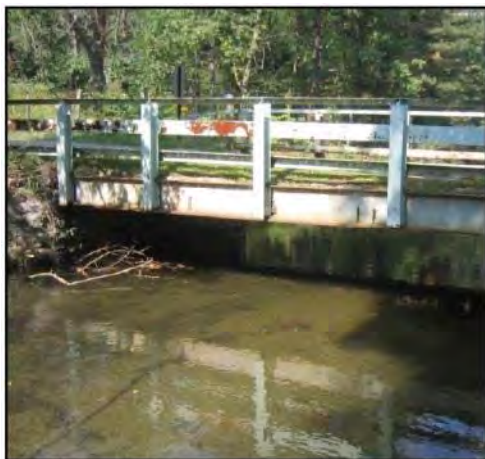
FIGURE I-3: Ross Mountain Park Bridge before Replacement (Gargan 2010)
