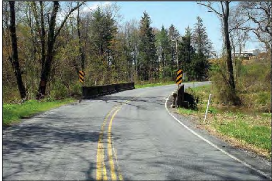
FIGURE I-13: Gardners Bridge, 2015 (Courtesy of PWKP 2018a)
