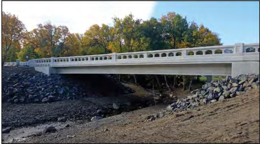
FIGURE I-8: Chenoweth Creek Bridge, August 2017 (Courtesy of Oregon DOT 2019b)
