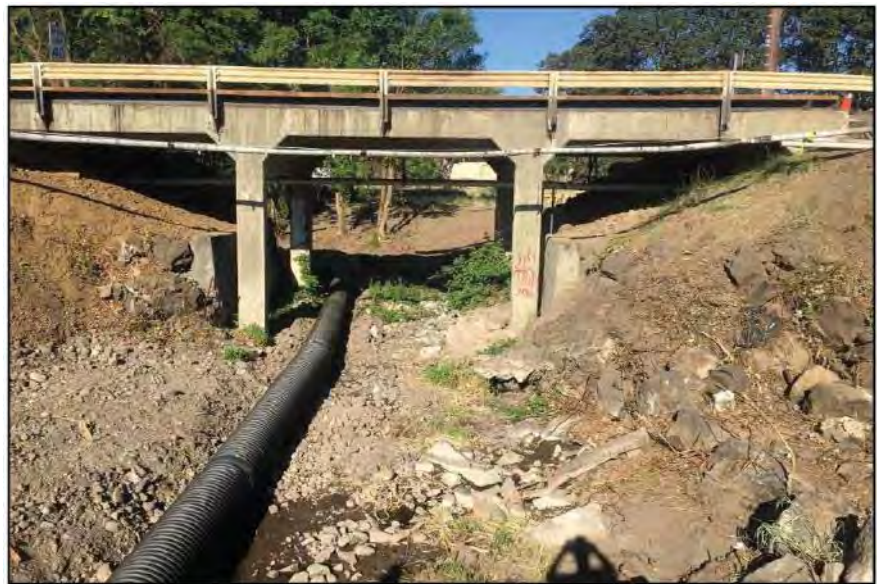
FIGURE I-5: Chenoweth Creek Bridge, May 2017 (Courtesy of Oregon DOT 2018)
