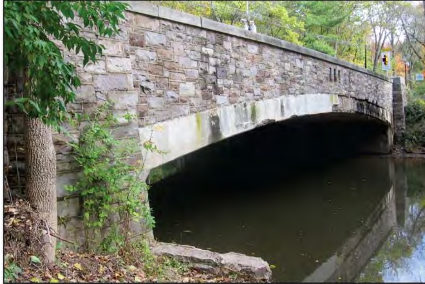
FIGURE I-20: Rosedale Road Bridge, April 2005 (Courtesy of IHE 2019b)
