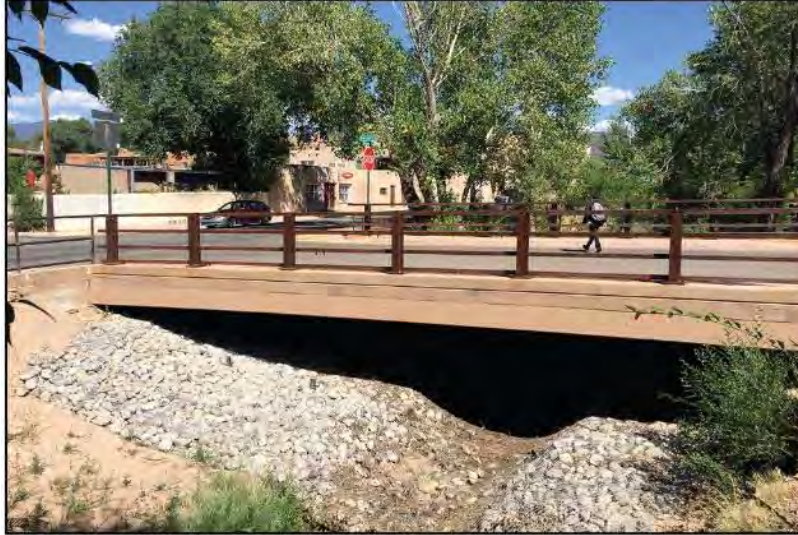
FIGURE I-30: Defouri Street Bridge, August 2017 (Courtesy of WSP 2019)
