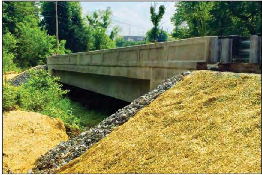
FIGURE I-2: Bridge over Bermudian Creek after Replacement, June 2018 (Courtesy of PWKP 2018d)
