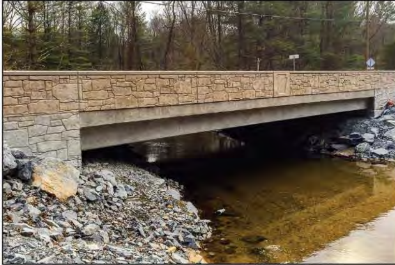
FIGURE I-18: Carlisle Road Bridge, January 2019 (Courtesy of PWKP 2019b)
