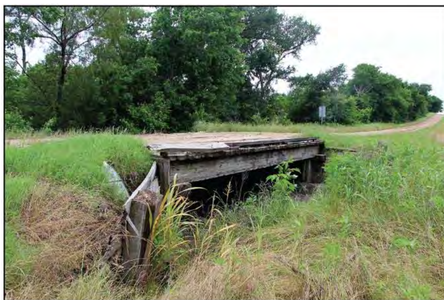
FIGURE I-39: Falls County Road Bridge, Ca. 2015 (Courtesy of Texas DOT/Mead & Hunt 2019)
