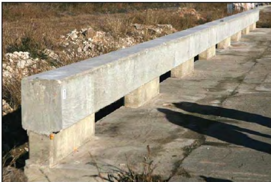
FIGURE I-40: T223 Railing (Courtesy of Texas DOT 2019)
