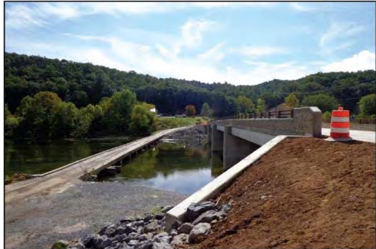
FIGURE I-43: Indian Hollow Road Low Water Bridge and New Adjacent Bridge (ACEC 2019)
