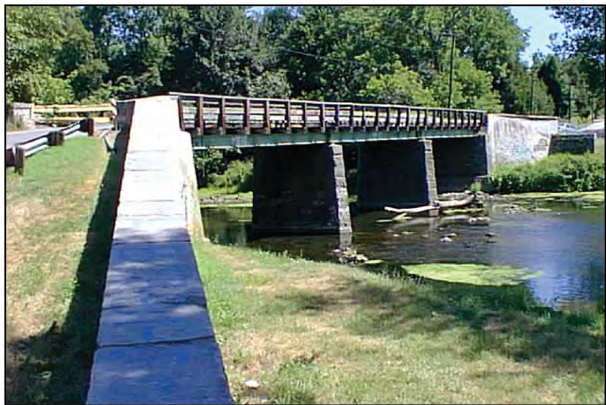
FIGURE I-22: Smith's Bridge , Ca. 2000 (Courtesy of Delaware DOT 2000b)
