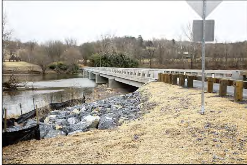
FIGURE I-52: Morgan's Ford Bridge Replacement Exhibits Compatible Abutment Design with the Natural Landscape (Courtesy of Trevor Wrayton 2019)
