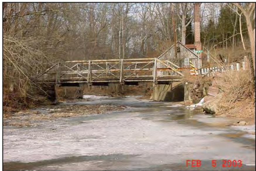
FIGURE I-31: Geigel Hill Road Bridge, 2003 (Courtesy of Benesch Engineering 2019)
