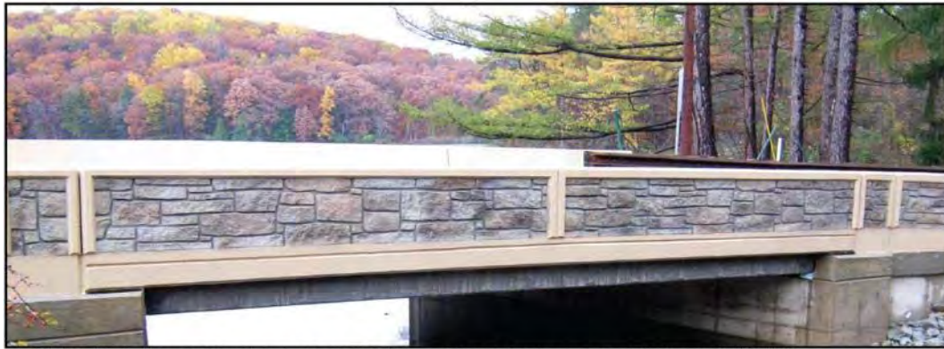
FIGURE I-4: Ross Mountain Park Bridge after Replacement (Gargan 2010)
