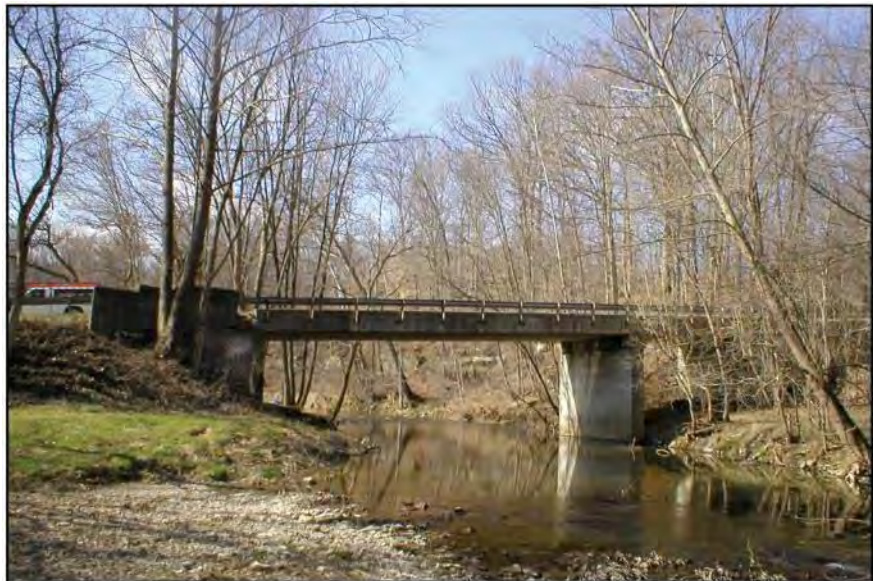
FIGURE I-25: Stinesville Road Bridge, Ca. 2010 (Courtesy of BLN 2019b)
