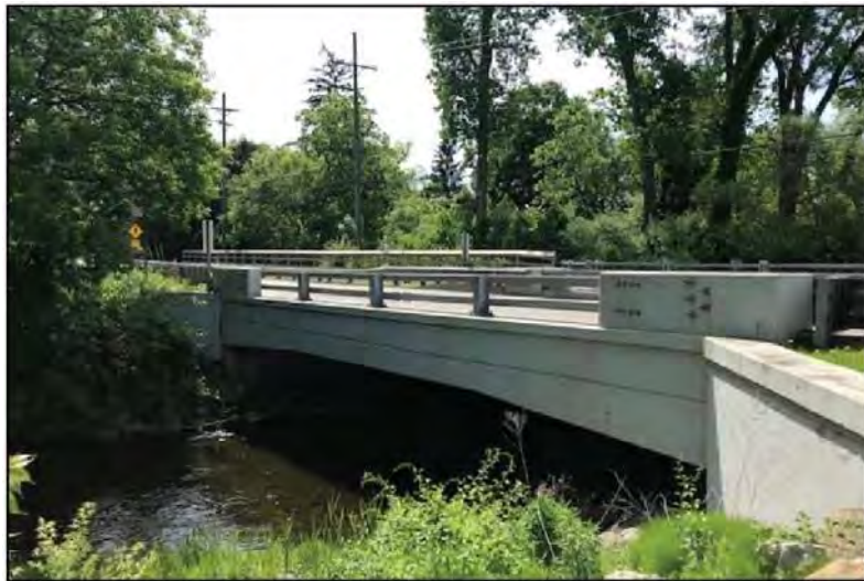
FIGURE I-45: Stoney Creek Mill Bridge Replacement, Rochester Hills, MI (Paul Graham, WSP)
