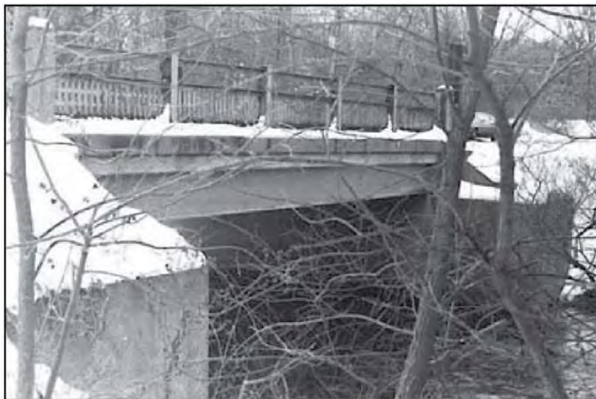
FIGURE I-33: Stoney Creek Mill Bridge, 1978 (Courtesy of RHM 2019)
