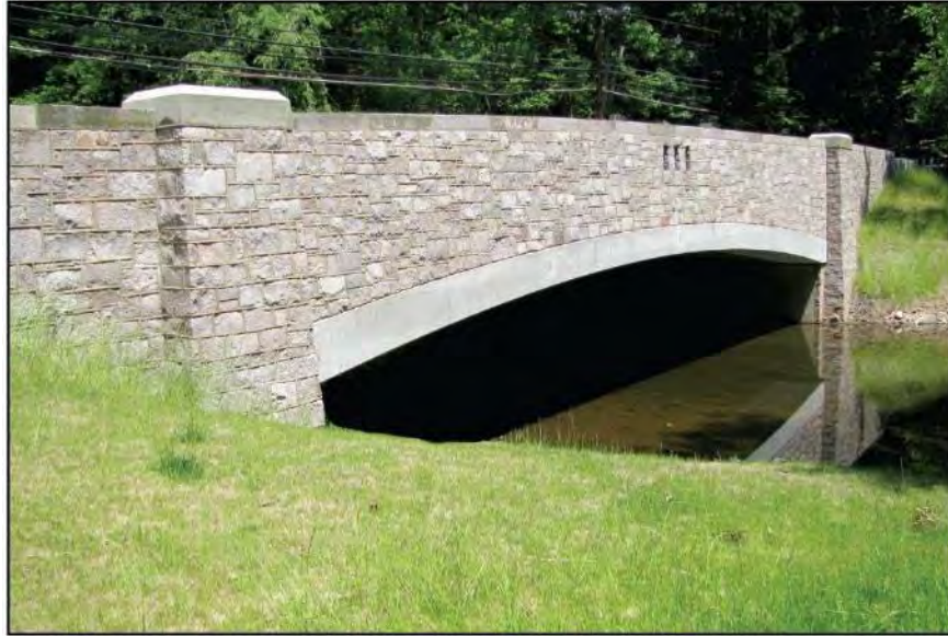
FIGURE I-21: Rosedale Road Bridge, September 2010 (Courtesy IHE 2019b)
