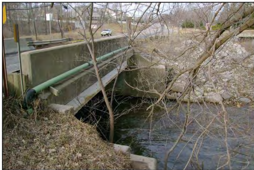
FIGURE I-34: Stoney Creek Mill Bridge with Concrete Barriers, Ca. 2008 (Courtesy of RCOC 2019)
