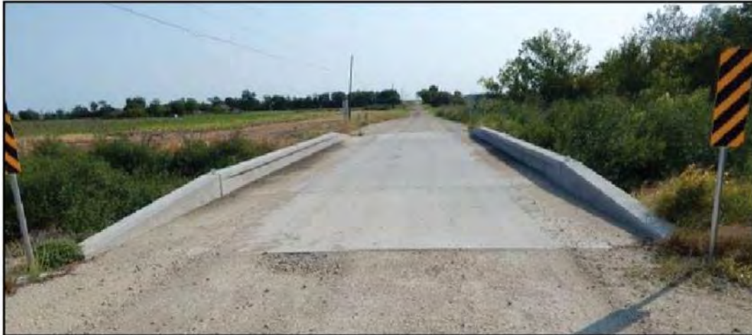
FIGURE I-41: Falls County Road Bridge, 2017 (Courtesy of Texas DOT 2017)
