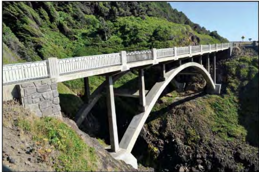
FIGURE I-9: Cooks Chasm Bridge, July 2011 (Photographer: Michael Goff, Courtesy of Bridgehunter.com)
