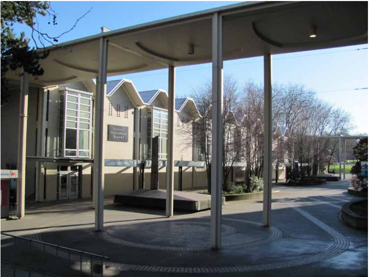
2013 view of former north entrance; Founders Court visible beyond the colonnade. Source: Artifacts Consulting, Inc.
