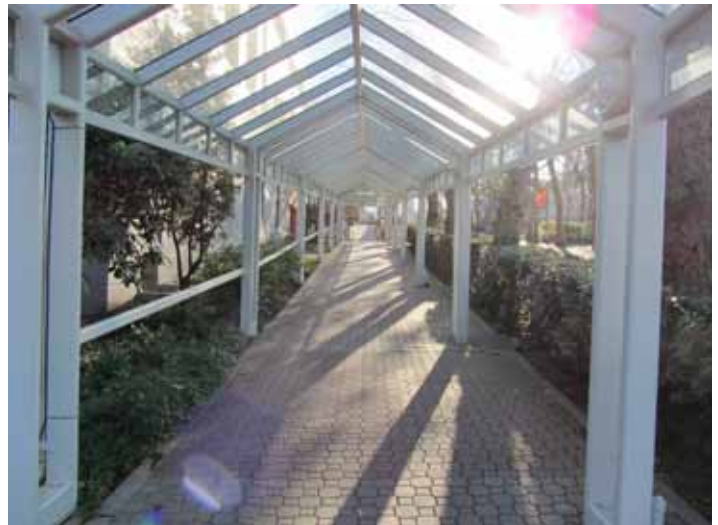
Above and right: 2013 images of covered breezeways. Source Artifacts Consulting, Inc.
