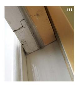
III: Nylon brushes being inserted into the sash as draught-proofing.
