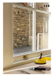
125–139: This sequence shows the addition of precision cut acrylic glazing to small paned windows. This allows the existing glazing to remain in place.
