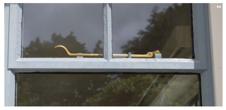
94: The new putty to this steel casement hasn't been allowed sufficient time to cure before being painted. Consequently the paint has blistered.
