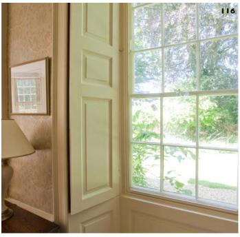
**115:** Failing plastic coated aluminium double glazed windows to this listed terrace house were replaced with single glazed timber casements to the correct historic pattern with secondary glazing incorporating Low E glazing giving a centre pane U-value of I.6w/m²K.
