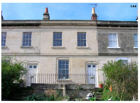
**140:** Windows of the original size and pattern have been reinstated in this south London conservation area which has involved reinstating the original masonry openings.
