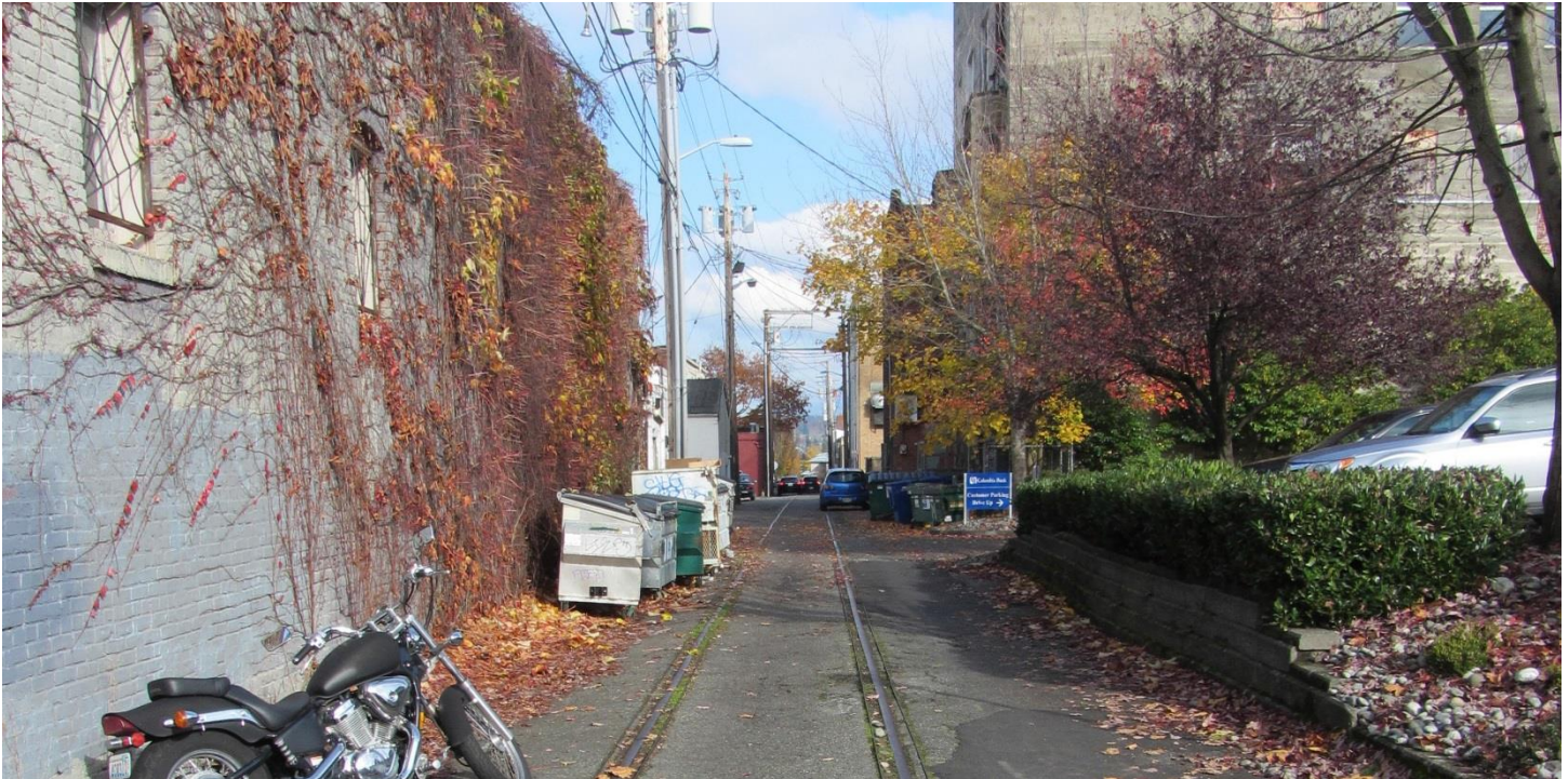
3 of 18. View looking northeast down the alley off East Holly Street showing the spur line.
