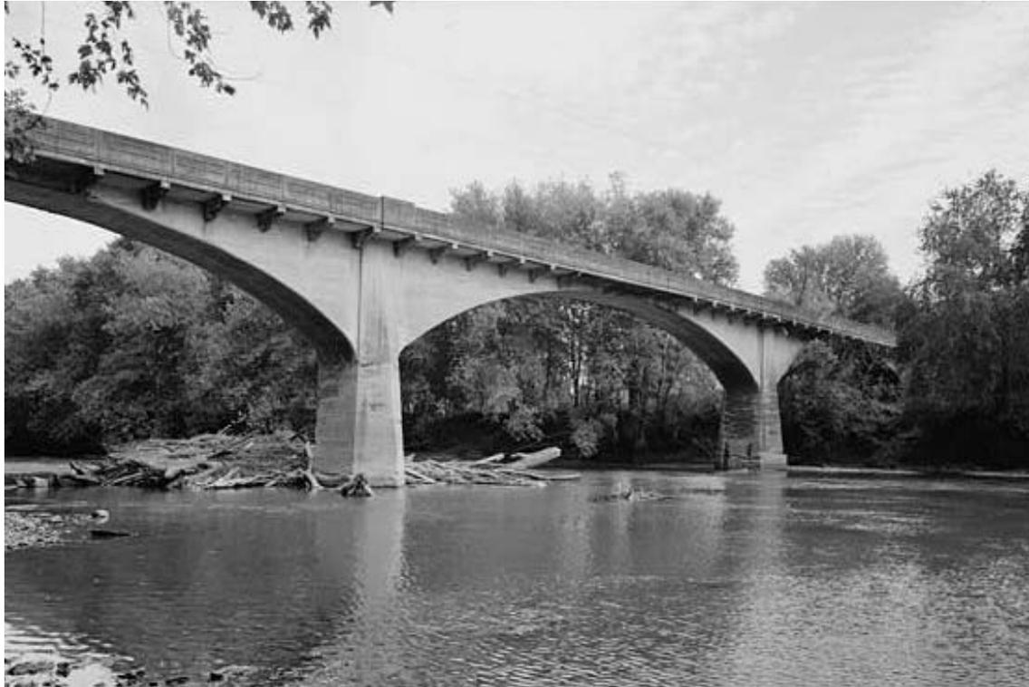
Figure 3-51. Milwaukee Street Bridge (1930), spanning Rock River, Watertown, Wisconsin. The photographs below show an example of the Luten open-spandrel arch.
