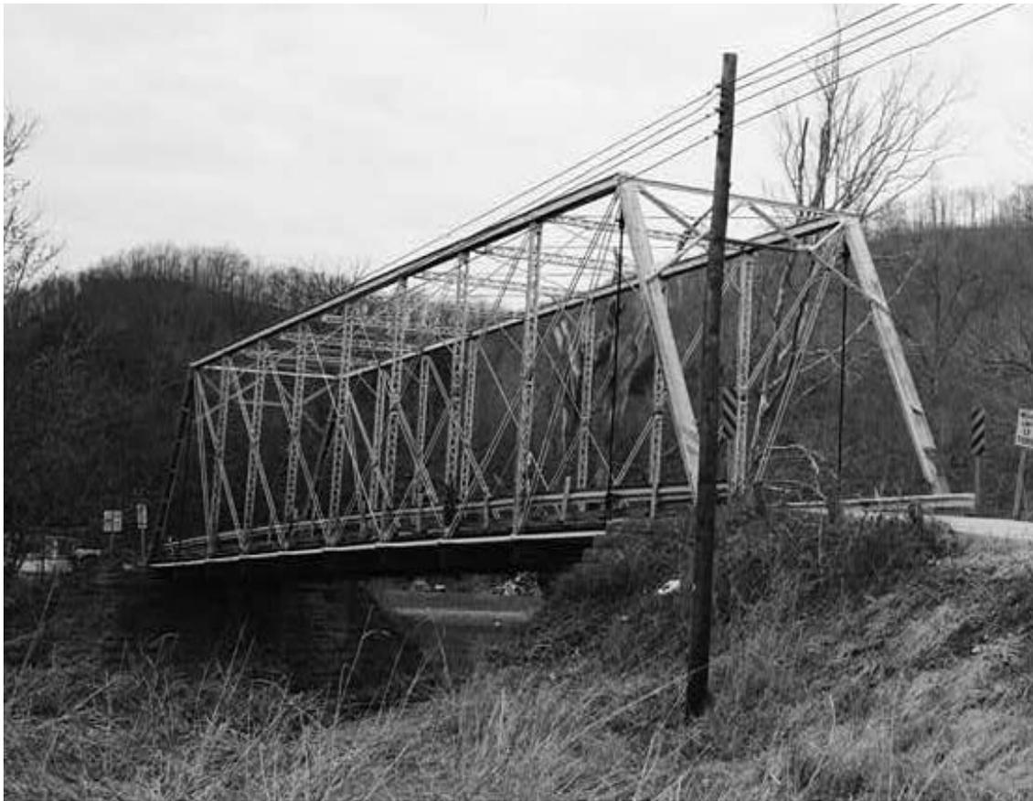
Figure 3-24. Laughery Creek Bridge (1878); Dearborn County, Indiana. This bridge is the only known example of the triple-intersection Whipple truss.
