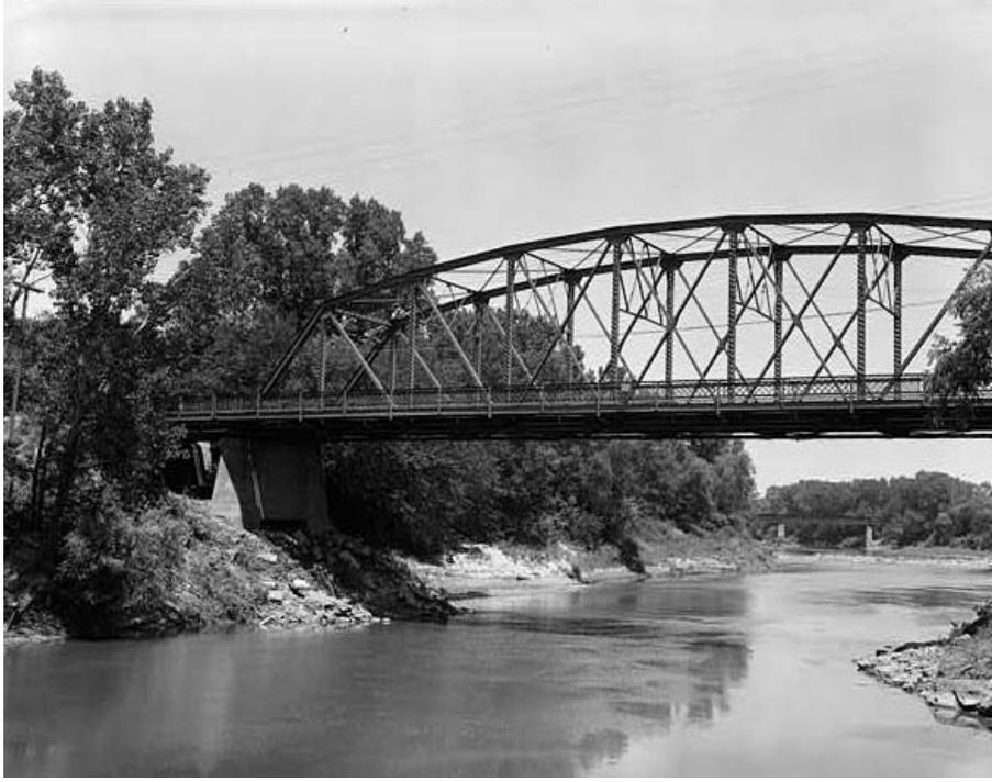
Figure 3-29. Sparkman (Shelby) Street Bridge (1907-09), spanning the Cumberland River, Nashville, Davidson County, Tennessee. This span is an example of the camelback variation of the Parker truss. Note the characteristic five slopes in the upper chord and end posts.
