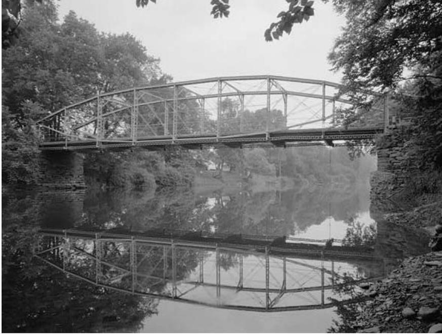
Figure 3-41. Nicholson Bridge (1888), Cemetery Road spanning Black Creek, two miles Southwest of Salem, Washington County, New York. This bridge is an example of the pony lenticular truss.
