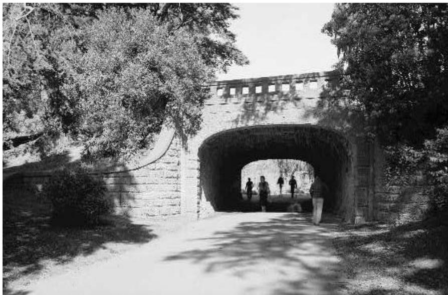
Figure 3-48. Melan Arch Bridge (1893), Emma Slater Park (Moved from Dry Run Creek), Rock Rapids vicinity, Lyon County, Iowa. The photograph illustrates an example of a von Emperger bridge.
