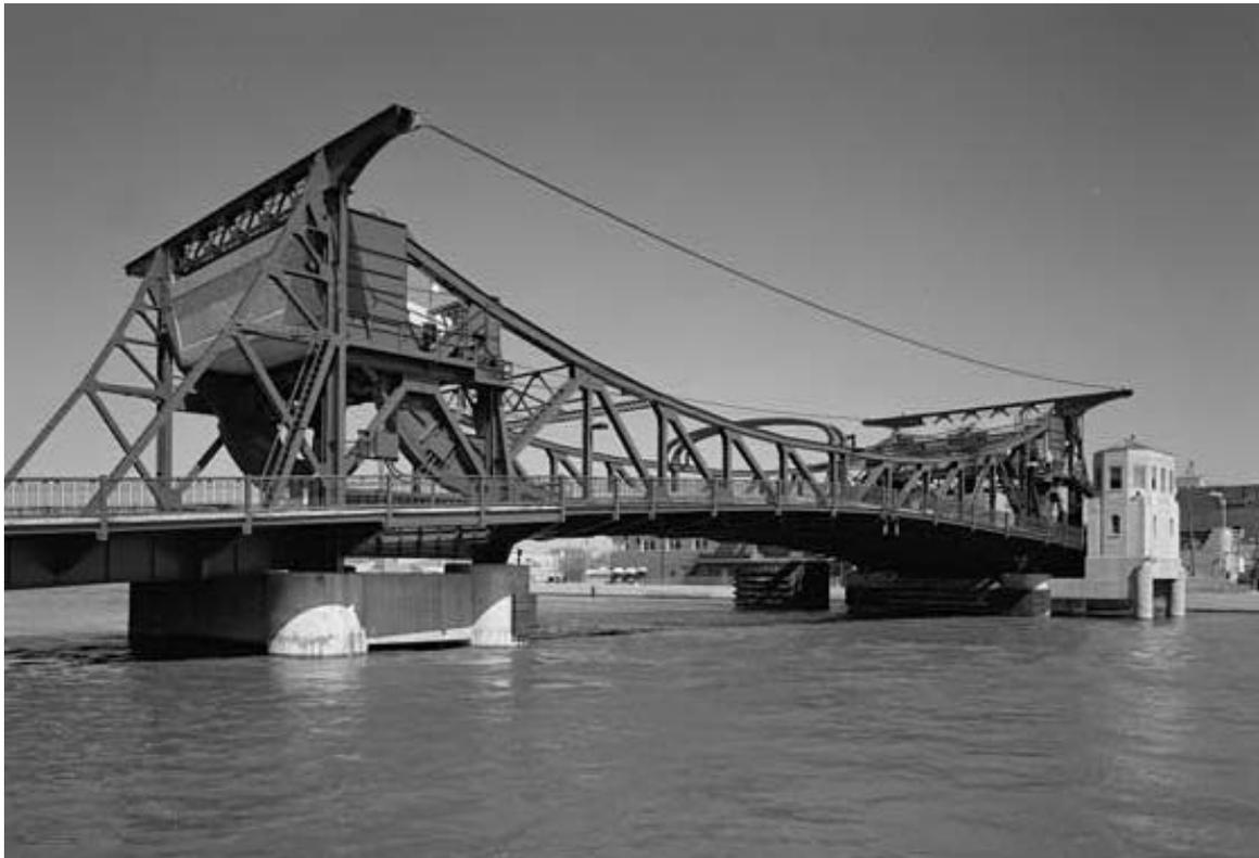
Figure 3-97. New York, New Haven & Hartford Railroad Bridge (1907), spanning Niantic River, East Lyme, Connecticut. This Scherzer rolling lift bridge is a through girder built for railroad use.
