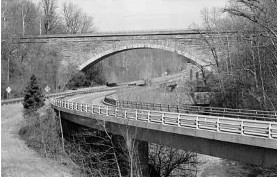
Figure 3-46. Possum Kingdom Stone Arch Bridge (1940-42), spanning Brazos River at State Route 16, Graford, Texas. This structure is an example of a Works Progress Administration-built stone arch bridge.
