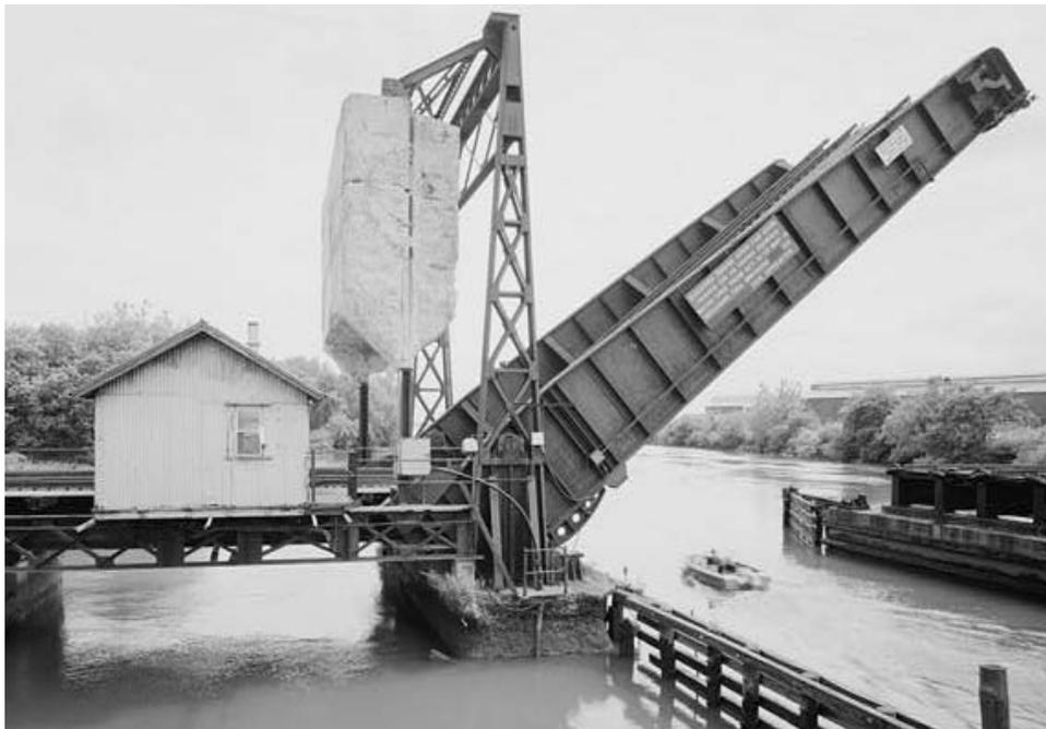
Figure 3-95. NJ-127 Route 7 Bridge (1925), Route 7 (1AG) over Passaic River, Belleville, New Jersey. This Strauss Bascule Company structure is a heel trunnion bascule.
