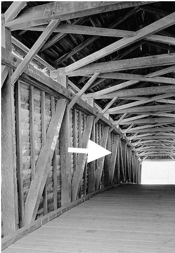
3-5b. *Interior view shows king post truss in the center (shown by arrow) with multiple panels to either side formed by vertical posts with diagonal counters matching the angle of the diagonals in the center truss, and a horizontal upper chord that is parallel with the lower chord.*
