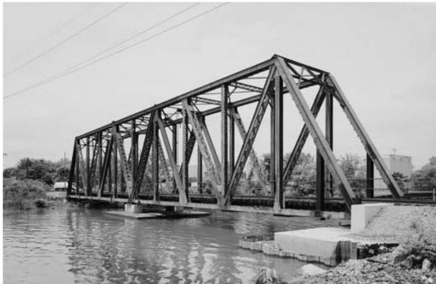
Figure 3-87. Chester & Delaware River Railroad (1907), spanning Chester Creek, Chester, Pennsylvania. When built, this swing bridge was hand operated.
