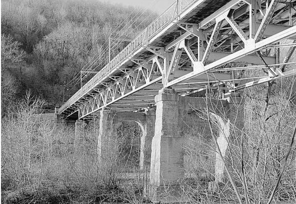
Figure 3-36. Spavinaw Creek Bridge (1909), Benton County Road 29 spanning Spavinaw Creek, Gravette vicinity, Benton County, Arizona. This structure is an example of the Warren bedstead truss.
