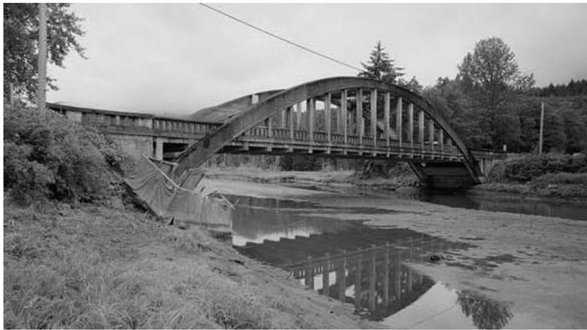
Figure 3-63. North Hamma Hamma River Bridge (1923); Mason County, Washington. This structure is a three-hinged concrete arch bridge built by Washington State Highway Department.
