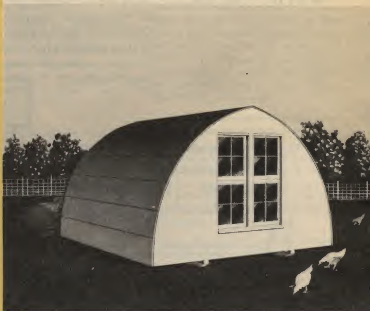
Chicken Brooder — No. 406 ● A new modern type. This design makes use of \frac{1}{4} " plywood. Building is planned in 4' sections for easy shipment—sections being assembled at site. Exterior of plywood with roll roofing on roof; insulating board lining optional; double floor; capacity 400 chicks. Ground Size 12 x 12.
