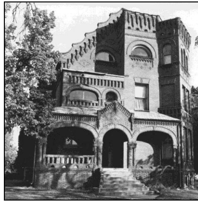
Figure 5: Hallett House in Medical Lake.
