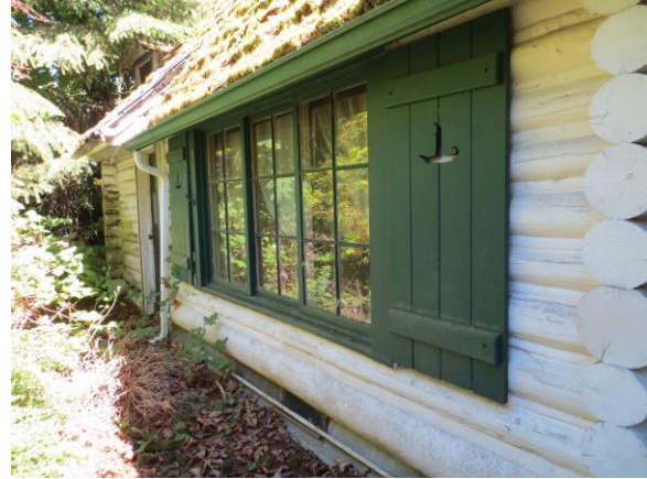
oblique view of north facade 2015
