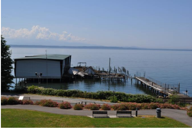
Demolished Meadowdale Marina Building with intact boathouse. Haines Wharf Park visible in image foreground. demolished Meadowdale Marina Building 2015
