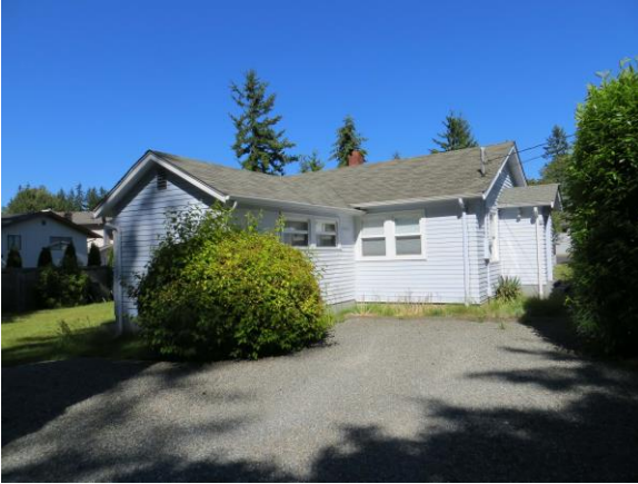
oblique view of east and north facades 2015
