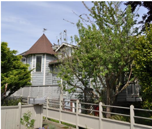
west facade and turret detail 2015
