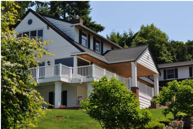
oblique view of north and west facades 2015
