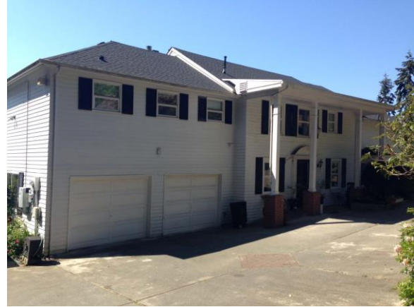
oblique view of north facade 2015
