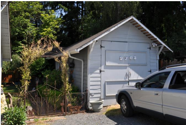
west facade of 9705 2015
