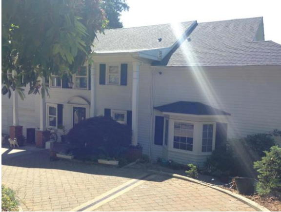
oblique view of north facade 2015
