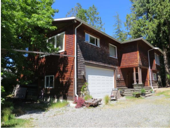
oblique view of SW facade 2015
