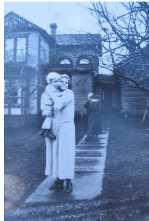
Historic Photograph from homeowner's collection. Date unknown. Bigelows in front of south facade, historic entrance 2015
