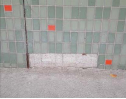
Substitute materials to replicate authentic materials found their way to mid-century storefronts just as terra cotta imitated stone on turn-of-the-century facades. This panel replicates tile pieces, yet there were other panels of materials copying stone, stucco or concrete.
