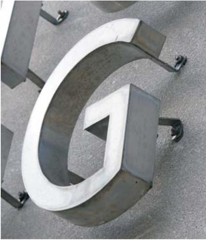
Individual letters were available in a variety of mid-century clean-lined scripts. Made out of stainless steel, painted sheet metal, aluminum or bronze, they were usually pinned to the wall or mounted to a canopy or
