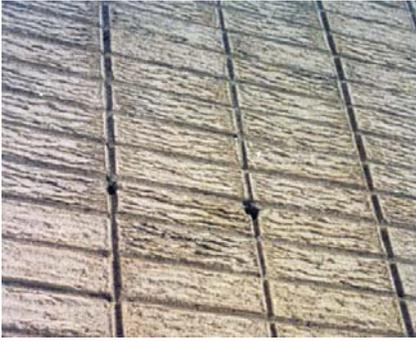
Unusual and textured masonry surfaces were utilized. Often as a contrast to smooth metals and sheets of plate glass. Brick was often stacked in a vertical bond. This provided clean vertical lines for the modern aesthetic.
