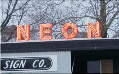
Channel-set neon tubing was set within metal letters with the neon tubes left uncovered and visible. Since the 1970’s most new channel-set letters had their neon hidden by a cover of translucent plastic.
