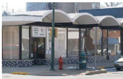
Some designers experimented with new developments in roofing technologies. This barrel vaulted roof protected the sidewalk as a canopy.
