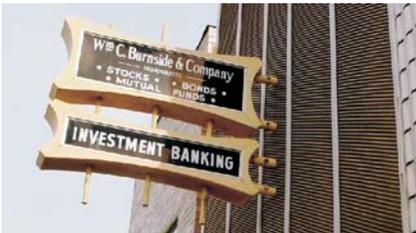
Internally illuminated back-lit use a metal box to hold a light source (either fluorescent or white neon) that is covered by a translucent plastic or glass face onto which graphics were printed. New internally illuminated plastic signs are generally not recommended for historic districts; however, some internally illuminated plastic signs may be old enough or integral enough to the building design or business to consider their preservation.
