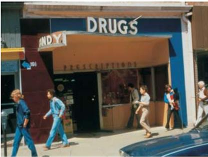
Jutting canopies replaced traditional fabric awnings. Some were supported by rods, and columns, while other steel and concrete canopies were cantilevered without visible support. They were made of steel, aluminum, concrete or wood. These canopies provided sun screening and also a location for individual letter signs, attached either above, or suspended below the canopy. Although most canopies were rectilinear, some incorporated sweeping curves.
