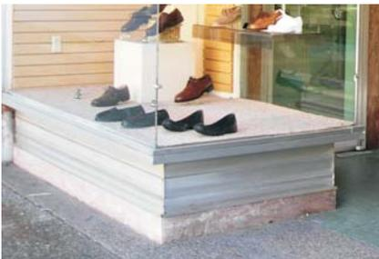
Cantilevered display windows projected beyond their base to further deconstruct the storefront plane. By recessing the base, the display seemed to float, and the exterior lobby felt more spacious.
