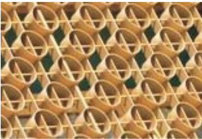
Not all striking modern facades of the mid-century were slipcovers over earlier buildings. Many stores were built in the 1950's. New construction and slipcovers alike could be covered with opaque materials of glass, steel, aluminum or porcelain enamel, or with perforated metal screens that let in sunlight to upper floors. The screens were usually anodized aluminum and were made in a variety of colors.
