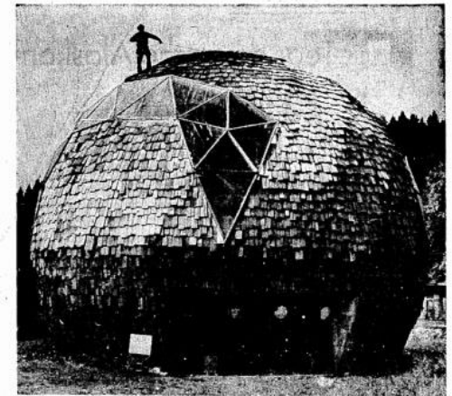
Steve Bondelid checked for loose shingles.
