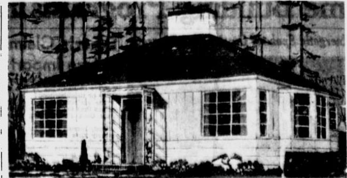
Preliminary work is under way for construction of this attractive conservative-modern style home for J. Orville Westberg of the Exchange Lumber company on Twenty-ninth, east of Bernard. The design is by Edwin J. Peterson, Spokane architect. The $4000 class home is being built by William Bengel, contractor. It contains four rooms and a dining bay. A hot-air heating plant is planned for the half-basement. The exterior will be white, with stained roof. Both wide siding and vertical boarding will be used.
