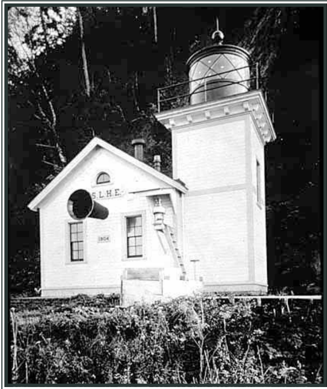
Slip Point Light House Station. Courtesy U.S. Coast Guard
