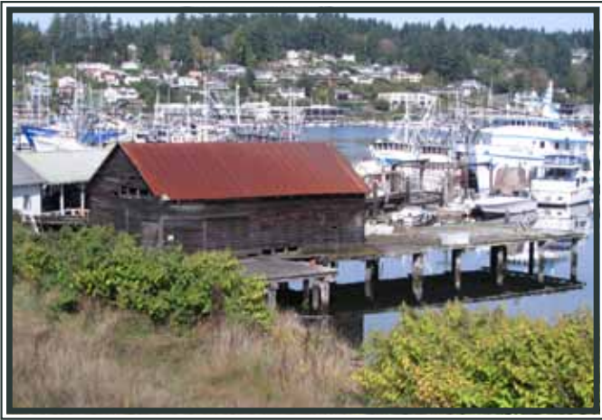
View of the Gig Harbor waterfront with the Ancich-Rainier Netshed in the foreground. Image courtesy of Artifacts Consulting, Inc., 2011.
