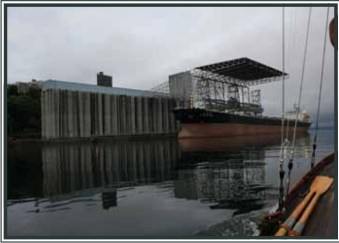
2010 view of the grain silos along Commencement Bay. The grain silos along Tacoma's waterfront continue to load oceangoing vessels. Located along the railway, they receive grain by rail car bound for international markets. Image courtesy of Artifacts Consulting, Inc.
