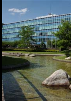
WWP Building Spokane, 1959
