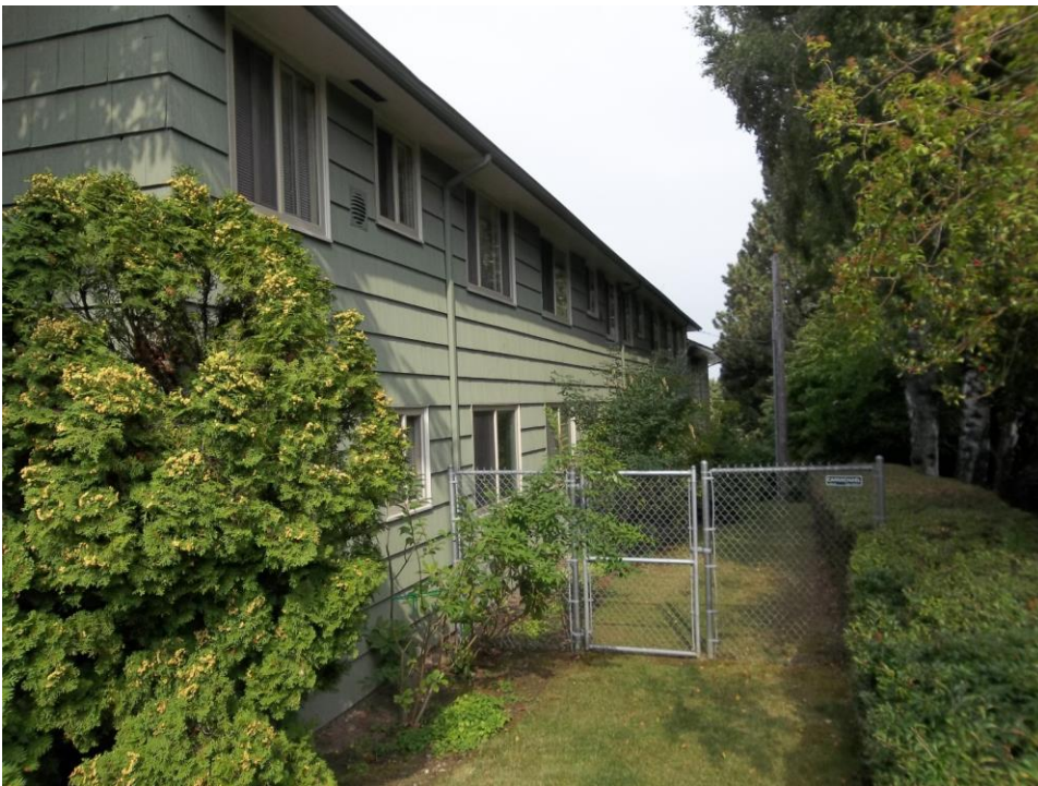
5 of 19 Northwest boundary line from North Forest Street at Building No. 2.
