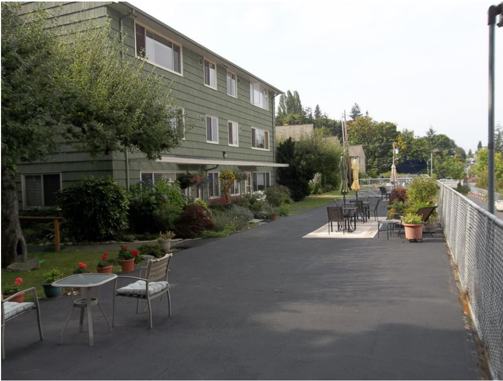
10 of 19 Roof of carport and Building No. 1 in background.
