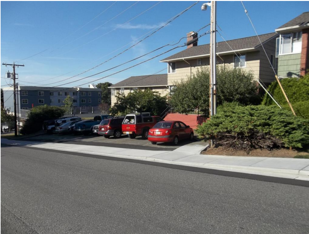
8 of 19 Southeast boundary on Berry street, showing Building No. 5 and parking area.
