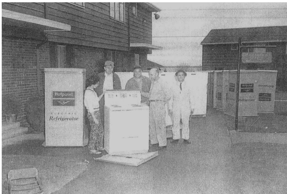
Orchard Terrace – Image from Advertisement for General Plumbing Co. July 17, 1971 – Photo courtesy of Whatcom Co. Museum, #1995.0001.023098
