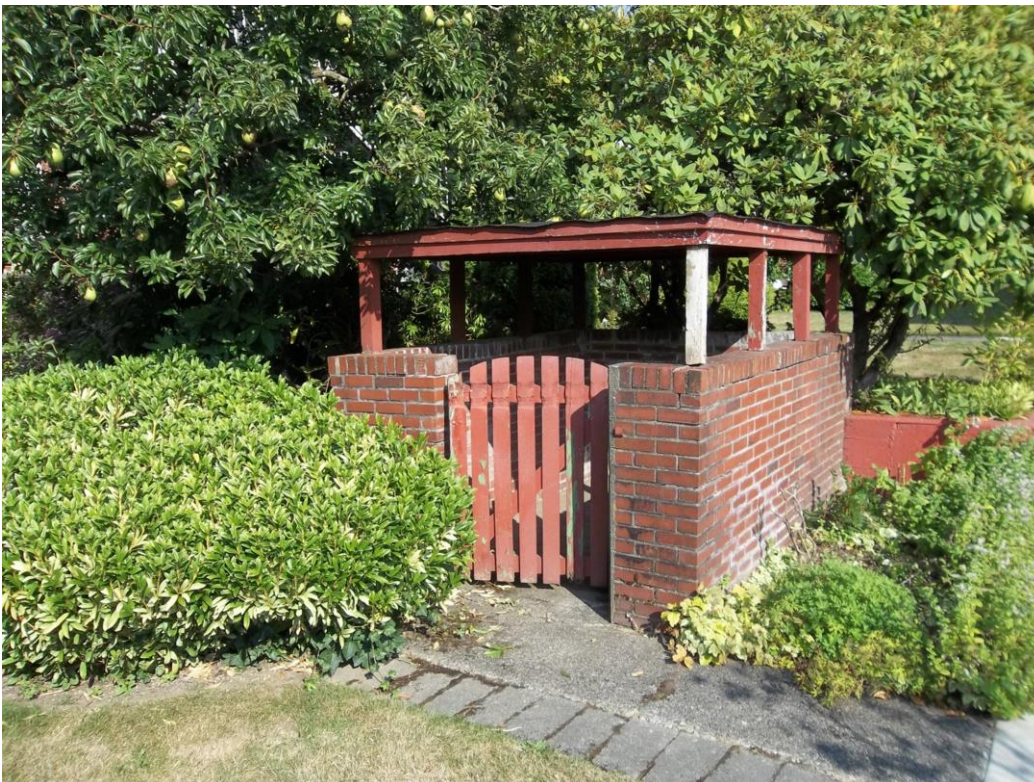
18 of 19 Waste storage pavilion within the landscaping.
