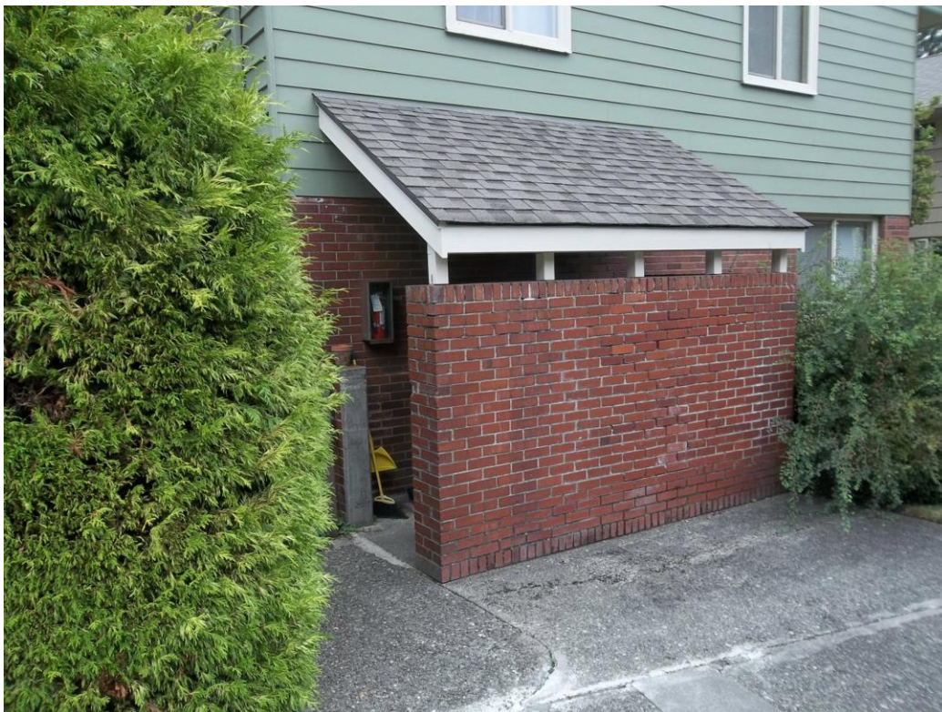
19 of 19 Waste storage pavilion attached to unit.
