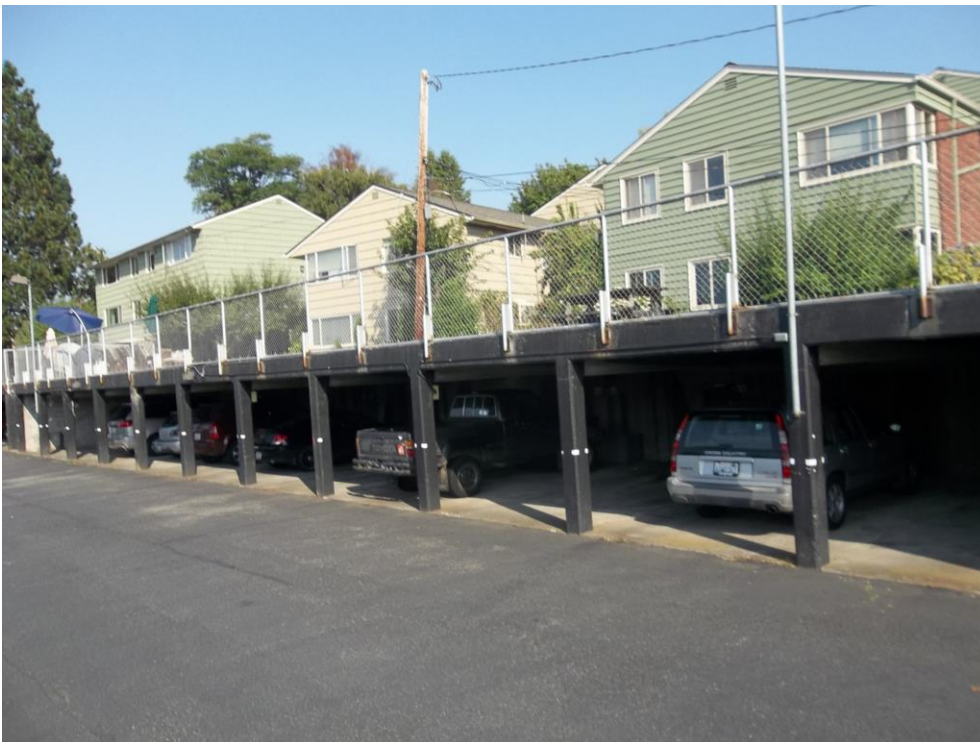
9 of 19 Northeast boundary, showing Carport and Building No. 2, 3 and 4.
