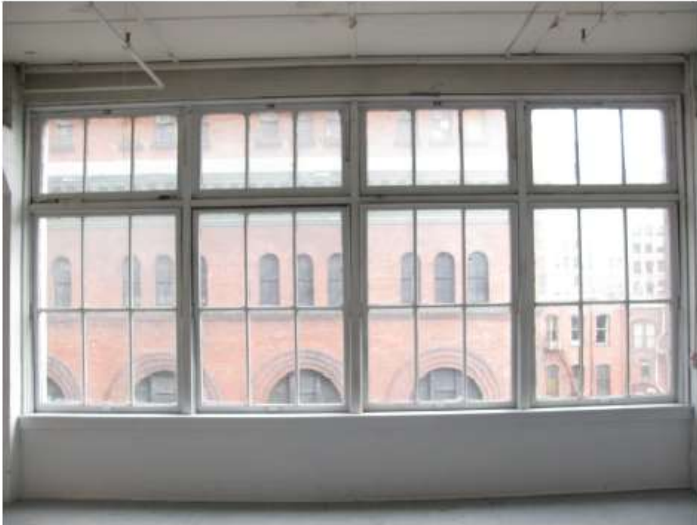
No. 33. 2012. Original wood windows--center pivot lower unit with transom hopper. Typical for stories two through five. Source: Historic Seattle
