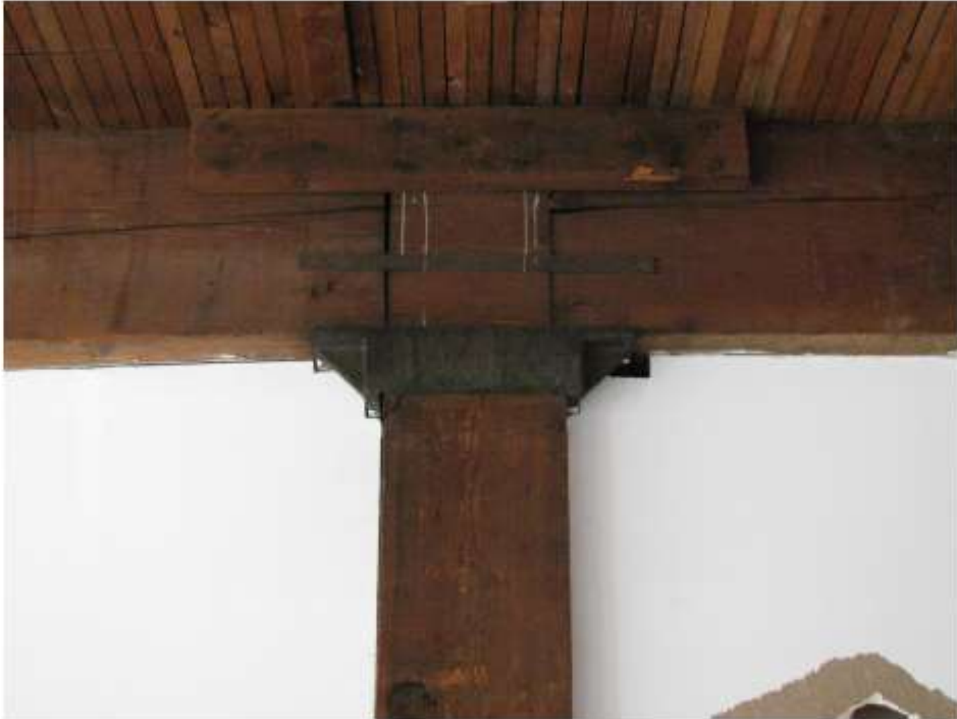
No. 34. 2012. Detail of heavy timber beam, column and connection. Car deck ceiling visible. Sheetrock wall is non-historic. Source: Historic Seattle
