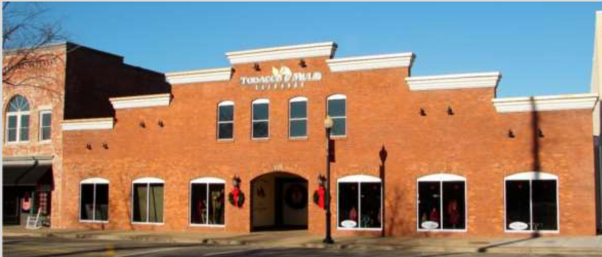
Project denied for incompatible work completed prior to Part 2 review.
