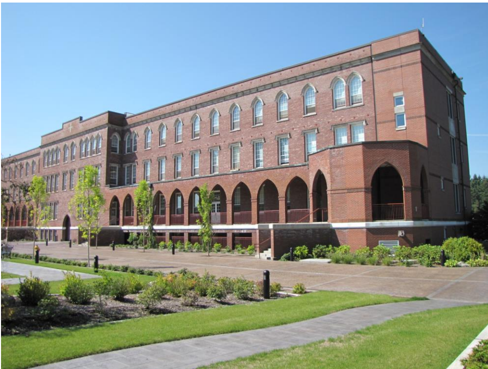
5 of 14 Rear courtyard area – showing 1989 stairwell addition, Michael Houser, August 25, 2014
