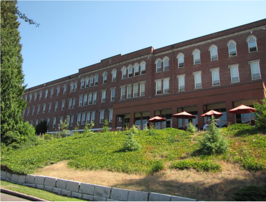
6 of 14 West Façade – 1923 rear wing, Michael Houser, August 25, 2014
