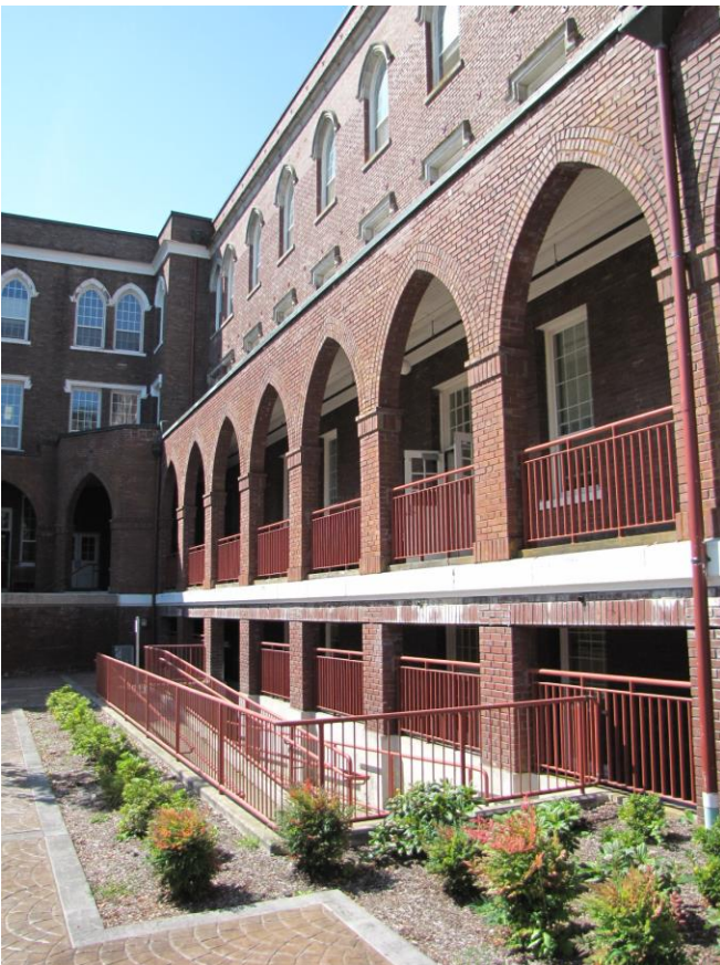
7 of 14 Courtyard Façade – Showing exterior arcade, Michael Houser, August 25, 2014
