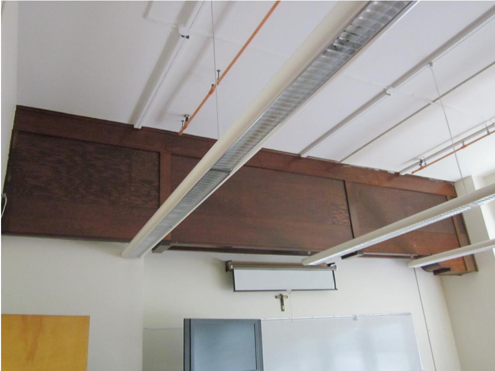
14 of 14 Structural Beam in Classroom – 1923 wing, Rebecca Sill, August 1, 2014
