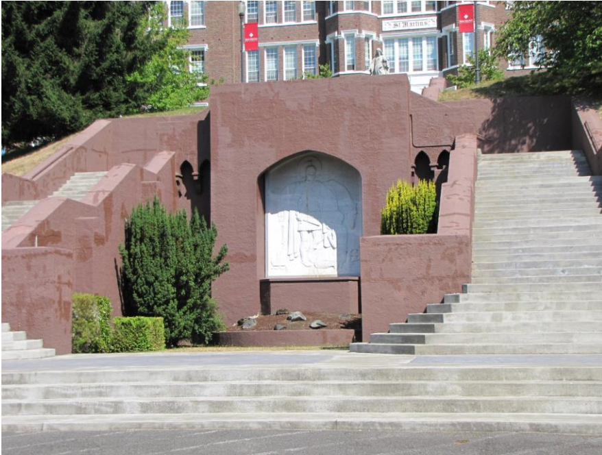
8 of 14 Main Entry Stair Detail, Michael Houser, August 25, 2014
