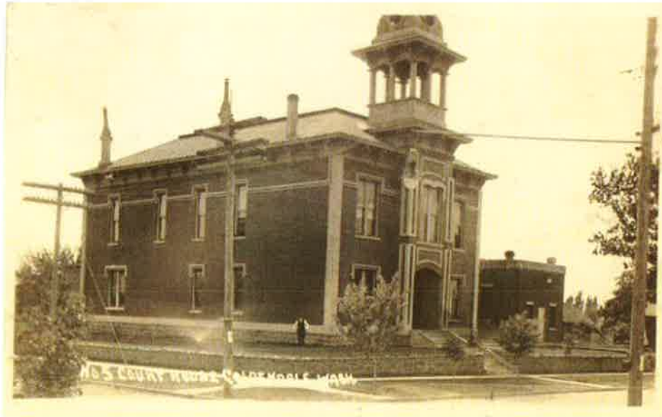
Figure 8: 1889 courthouse building. Jail in foreground (at far right).
