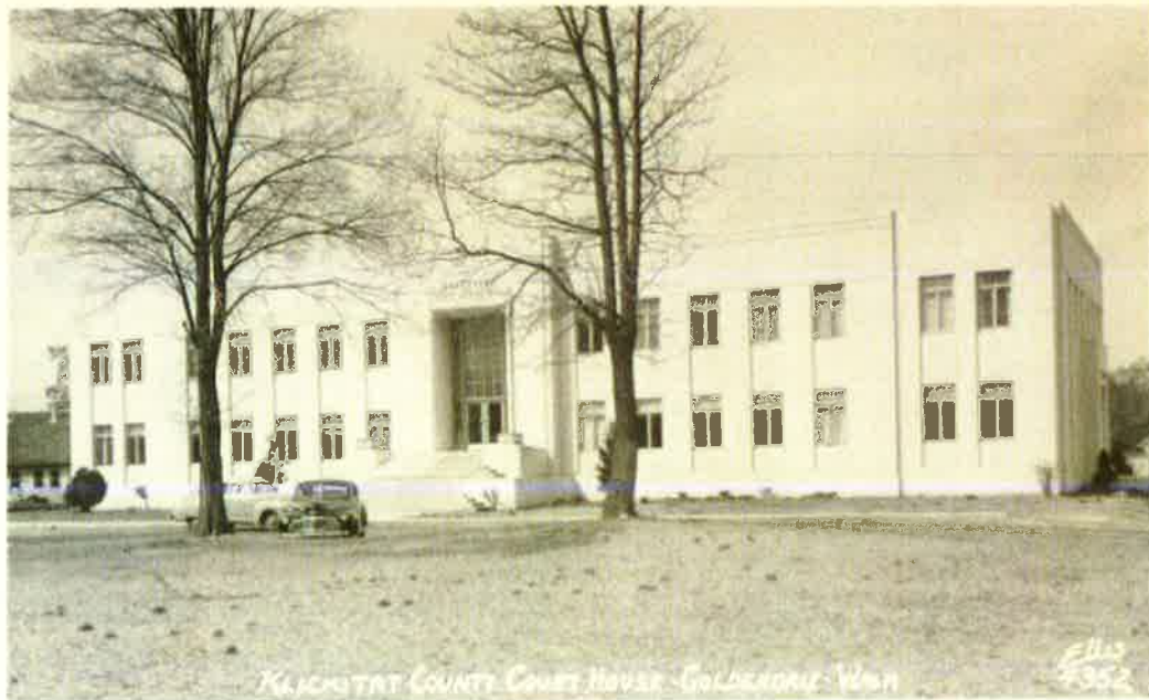
Figure 13: Courthouse, main façade. ca.1945.
