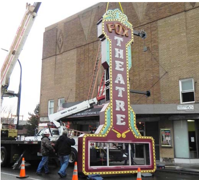
Installation of the Fox Theatre sign in downtown Centralia.
