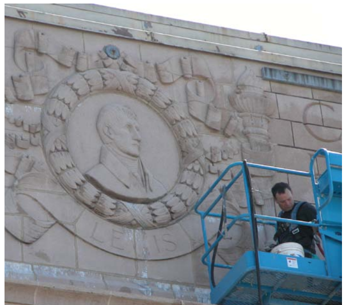
Work on the detail of the Lewis County Courthouse in Chehalis.
