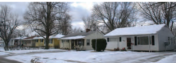
Figure 8. Modified Gunnison houses in the Maenner South Addition in Omaha, Nebraska. This streetscape documents the similar form and massing and setbacks within the addition (Mead & Hunt photograph).
