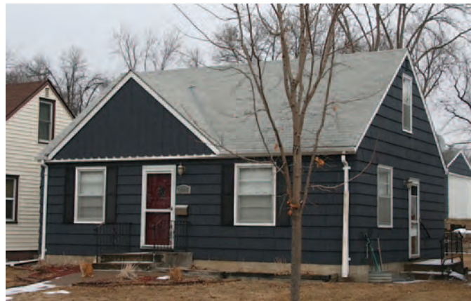
Figure 2. Intact c.1945 house in the postwar St. Louis Park, Minnesota, neighborhood. This residence represents the Minimal Traditional form with a side gable roof and prominent gable above the entrance. The house retains the original footprint, wood shingle siding, and double-hung windows (Mead & Hunt photograph).
