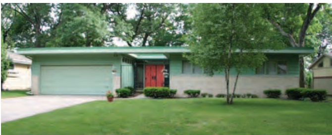
Figure 35. Contemporary house in Madison, Wisconsin, constructed in 1963, retains its original massing and window configuration and displays three architectural elements: combination of wood and brick siding, wrought iron ornamentation at the front entrance, and prominent roof cutout. As a result, it meets the survey criteria (Mead & Hunt photograph).
