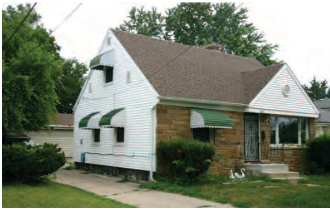
Figure 98. Simulated stone on facade of a c.1945 Minimal Traditional house in Lansing, Michigan (Mead & Hunt photograph).
