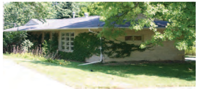
Figure 101. Grouping of 12 Flexivent windows on the rear elevation of a c.1953 Ranch home in Lincoln, Nebraska (Mead & Hunt photograph).
