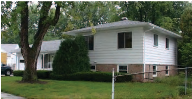
Figure 1. A prefabricated Harnischfeger residence erected c.1960 in the Northbrook Farms Subdivision in Mason, Michigan (Mead & Hunt photograph).
