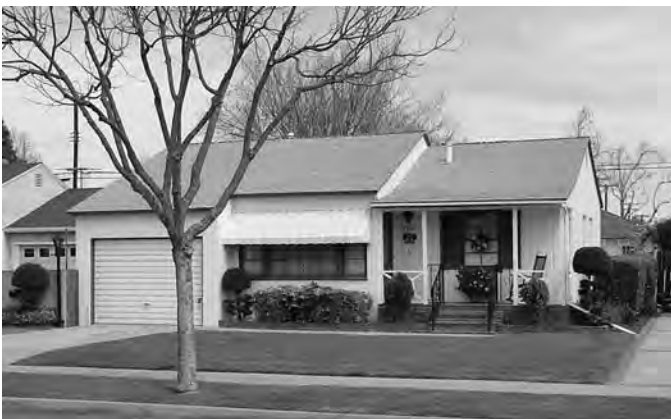
Figure 114. Minimal Traditional house in Lakewood, California, constructed c.1950, with side gable roof, stucco and vertical wood siding, inset entrance, minimal eave overhang, and attached one-car garage (photograph courtesy of Andrew Hope, Caltrans).
