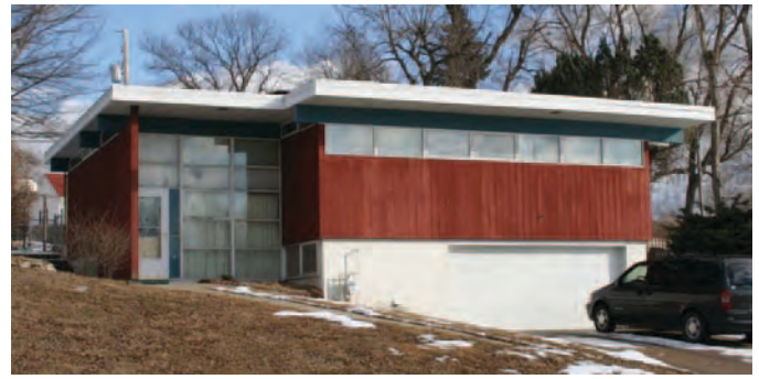
Figure 65. Contemporary house in Omaha, Nebraska, constructed c.1960, with a modern garage door replaced in-kind; it retains enough integrity to be considered individually eligible under Criterion C: Architecture (Mead & Hunt photograph).
