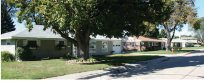
Figure 70. Although these 1950s Ranch houses in Lexington, Nebraska, have modified windows and garage entrances, they are considered contributing in a potential historic district (Mead & Hunt photograph).
