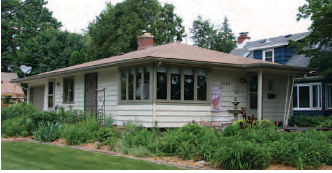
Figure 13. Transitional Ranch house in Madison, Wisconsin, constructed in 1949, retains its original siding, windows, and entrance with a decorative support, and thus meets the survey criteria (Mead & Hunt photograph).
