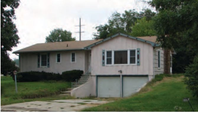
Figure 21. Raised Ranch house in Parkville, Missouri, displays only one original architectural element—the combination of board and batten and clapboard siding—and as a result does not meet the survey criteria (photograph courtesy of Toni Prawl, Missouri Department of Transportation).
