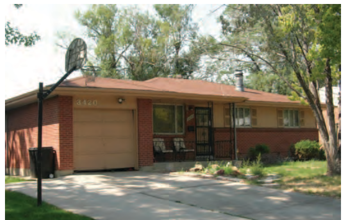
Figure 102. Ranch house in Westminster, Colorado, with a hip roof, partial brick veneer, recessed entrance with decorative wrought iron details, and decorative shutters (photograph courtesy of Dianna Litvak, Colorado Department of Transportation).
