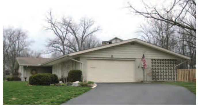
Figure 96. Concrete screen providing increased privacy at the rear patio of this c.1966, Worthington Hills, Ohio, Ranch house (Mead & Hunt photograph).
