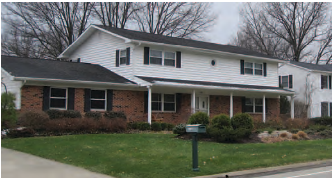
Figure 141. Two-story Massed house in Worthington Hills, Ohio, constructed c.1966, exhibits Colonial Revival style details, including symmetrical fenestration, wide overhanging eaves, faux shutters, compass windows, and simple porch across the facade (Mead & Hunt photograph).
