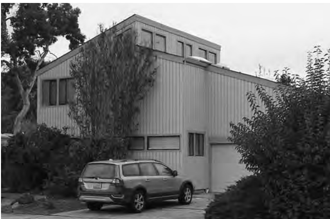
Figure 157. Shed house in Palo Alto, California, constructed c.1972, with intersecting shed roof lines, wood siding, clerestory windows, and an integrated garage (photograph courtesy of Andrew Hope, Caltrans).
