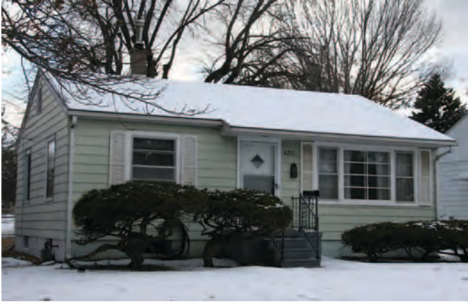
Figure 9. Minimal Traditional house in Omaha, Nebraska, constructed c.1945, retains its original siding, massing, simple entrance, and windows, and thus meets the survey criteria (Mead & Hunt photograph).
