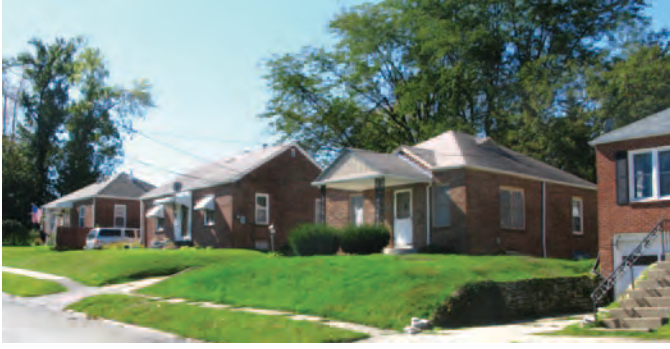
Figure 60. Minimal Traditional houses in the North Fellows Historic District in Ottumwa, Iowa, constructed c. 1945. Although some of the homes display exterior alterations, as a whole the district is able to convey significance (photograph courtesy of Molly Myers Naumann and the State Historic Preservation Office of the Iowa Department of Cultural Affairs).
