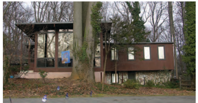
Figure 50. Residence in Greenbelt Knoll Historic District in Philadelphia (photograph courtesy of the Pennsylvania State Historic Preservation Office).
