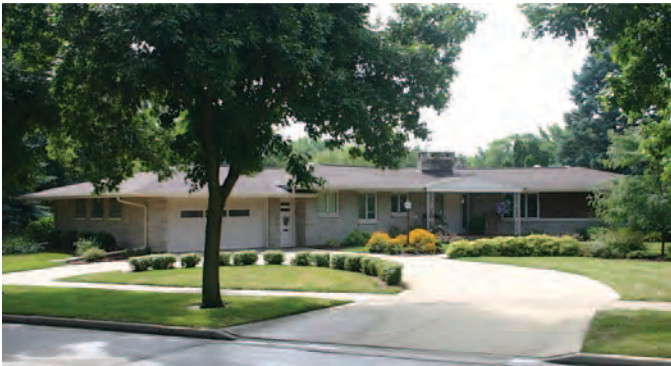
Figure 126. Ranch house in Sparta, Wisconsin, constructed c.1960, with horizontal massing, hip roof, stone veneer, casement windows, wrought iron supports at the entrance, prominent chimney, and attached garage. It is oriented diagonally on a large urban lot (Mead & Hunt photograph).
