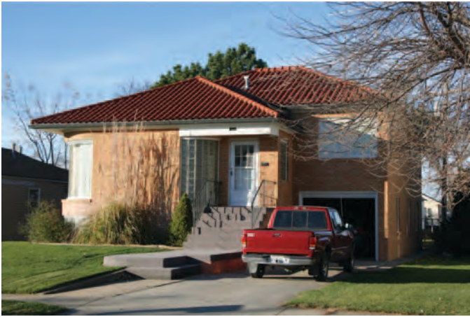
Figure 99. Raised Ranch house in Cozad, Nebraska, constructed c. 1955, with curved glass block windows near the entrance and at the basement level (Mead & Hunt photograph).
