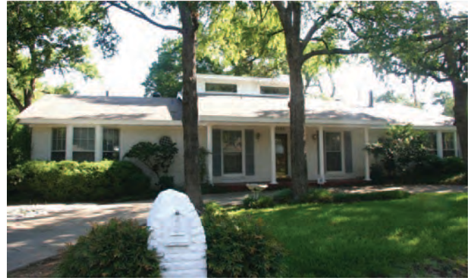
Figure 68. Ranch house in Arlington, Texas, constructed c.1965, with a modern shed dormer that alters the roofline and results in diminished integrity; it is considered not individually eligible (Mead & Hunt photograph).
