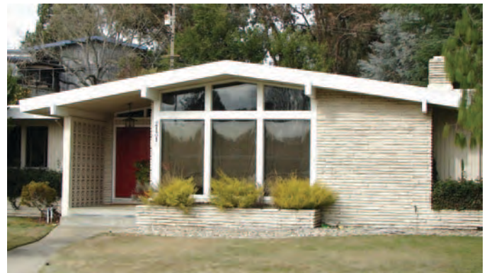
Figure 97. Concrete screen at the front entrance of a c.1964 Ranch house in Sacramento, California (photograph courtesy of Andrew Hope, Caltrans).
