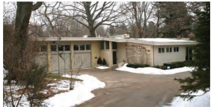
Figure 69. Contemporary residence in Omaha, Nebraska, constructed in 1954, with a modern three-car garage that replaced the historic carport; this alteration compromises the integrity, and the property is considered not individually eligible (Mead & Hunt photograph).
