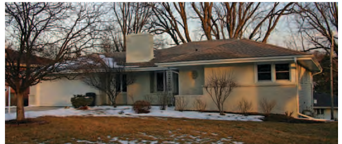
Figure 15. Ranch house in Omaha, Nebraska, constructed c. 1955, retains multiple architectural elements, including accent brick veneer, prominent wide chimney, integrated planter, and wrought iron support, and thus meets the survey criteria (Mead & Hunt photograph).
