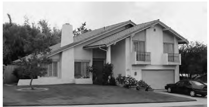
Figure 150. Spanish Colonial Revival style applied to the Split-level form in La Mesa, California, constructed c.1970, with stucco exterior and tile roof (photograph courtesy of Andrew Hope, Caltrans).
