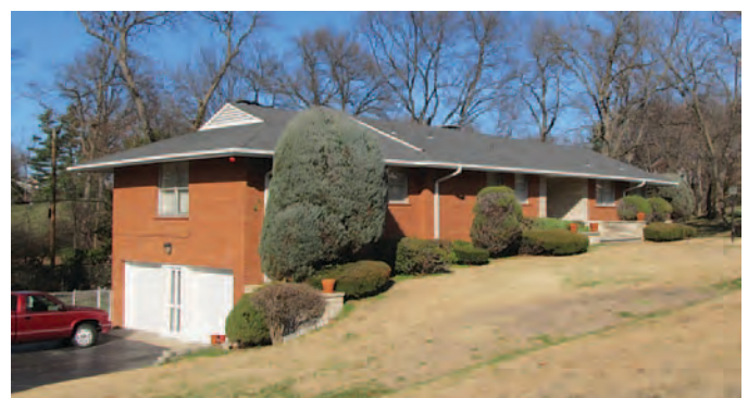
Figure 133. Raised Ranch house in Richmond Heights, Missouri, with the exposed basement at the side elevation, accent stone veneer, and planters (photograph courtesy of Toni Prawl, Missouri Department of Transportation).
