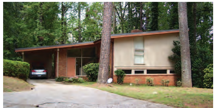
Figure 154. Contemporary style Split-level house in DeKalb County, Georgia, constructed c.1956, with a low-pitched roof, curtain wall at the entrance, minimal decorative details, and an integrated carport (photograph courtesy of Georgia Department of Natural Resources, Historic Preservation Division).
