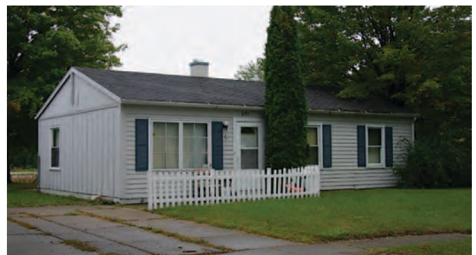
Figure 167. National Homes prefabricated house in the Snyder Subdivision in Mason, Michigan, erected c.1956, with replacement siding and windows (Mead & Hunt photograph).
