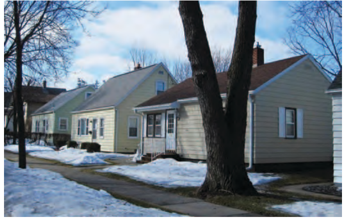
Figure 94. Three c.1945 Minimal Traditional residences in St. Cloud, Minnesota, with aluminum siding (Mead & Hunt photograph).
