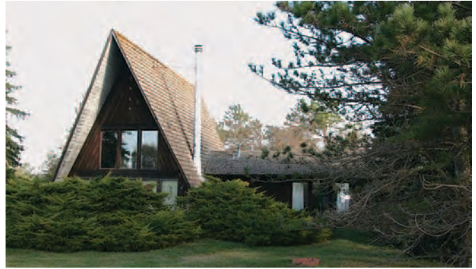
Figure 158. A-frame house in Overton, Nebraska, constructed c.1970, with overhanging eaves and a one-story addition on the side (Mead & Hunt photograph).
