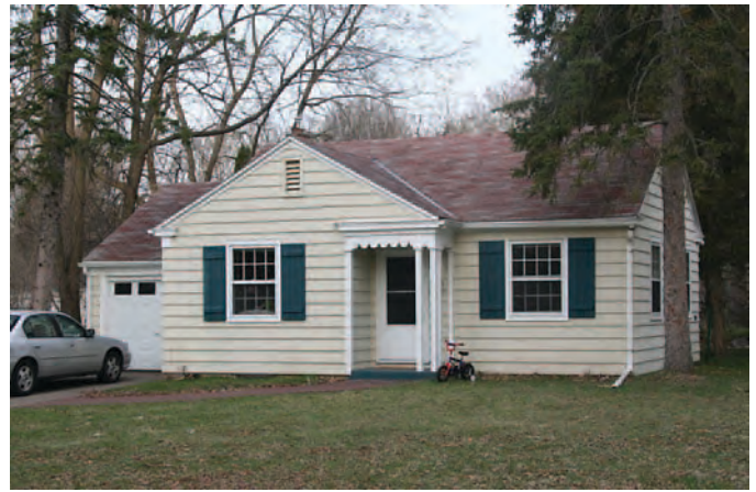
Figure 112. Minimal Traditional house in Madison, Wisconsin, constructed c.1945, with wood siding, compact one-story plan, minimal eave overhang, inset entrance, attached one-car garage, and modest Colonial Revival details, including gable end returns and cornice boards (Mead & Hunt photograph).
