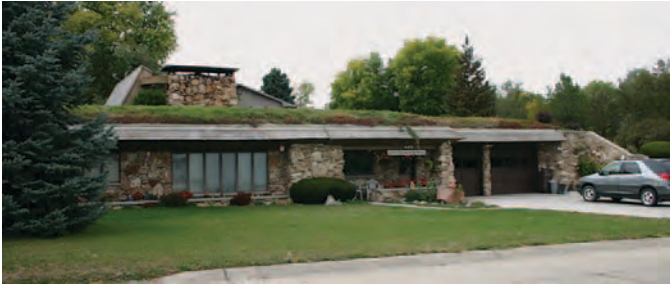
Figure 160. Earthen house in Broken Bow, Nebraska, constructed c.1975 into an embankment with only one exposed elevation (Mead & Hunt photograph).
