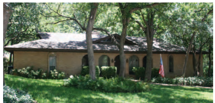
Figure 33. Spanish Colonial Revival house in Arlington, Texas, constructed in 1968, retains its form, massing, original cladding, arched porch and windows, and decorative wrought iron details. As a result, it meets the survey criteria (Mead & Hunt photograph).
