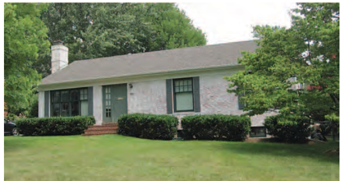
Figure 20. Ranch house in Arlington County, Virginia, constructed in 1959 that does not meet the survey criteria because the multi-light, “cottage-style” replacement windows are non-compatible. In addition, it does not display three architectural elements (Louis Berger photograph).
