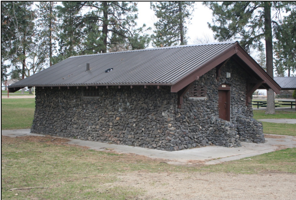
Figure 23: Glass Park Restroom
