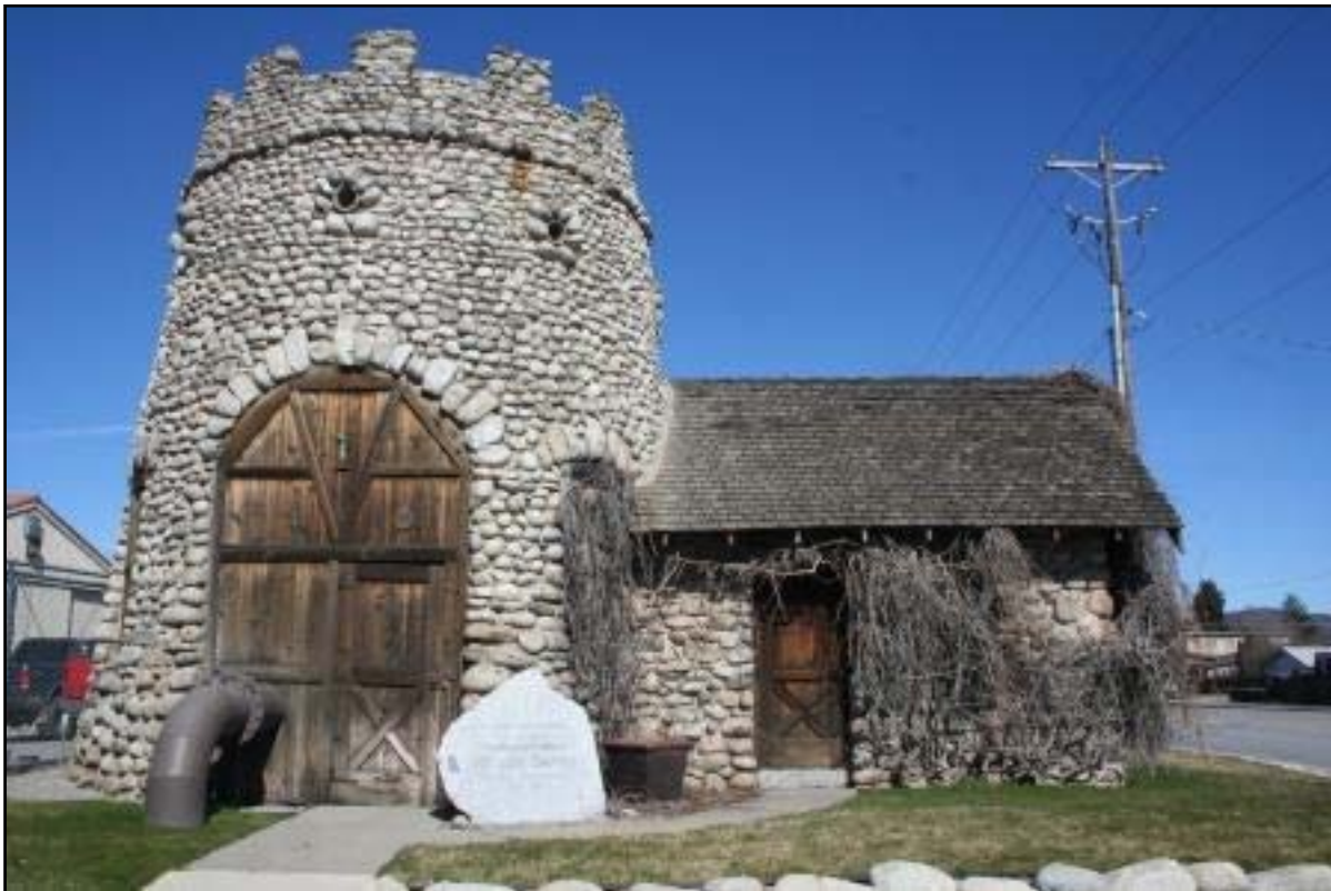
Figure 18: Vera Water and Power well house at 601 N. Evergreen Road
