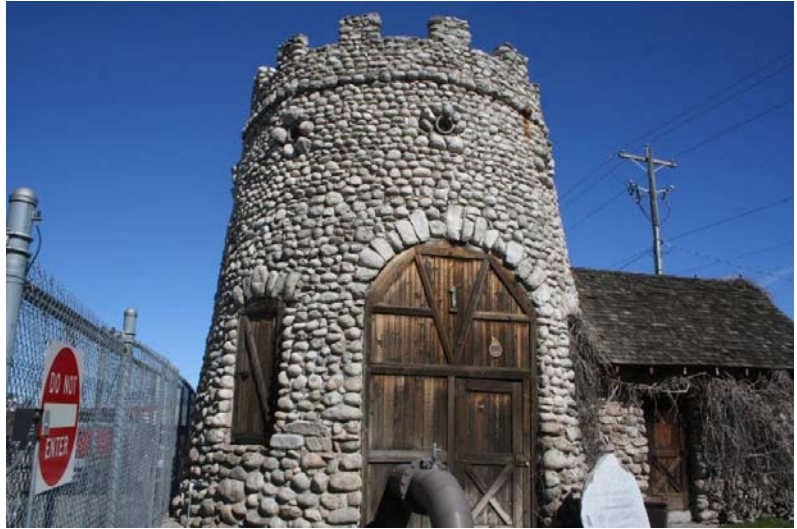
Figure 3: Vera Water and Power Well House
