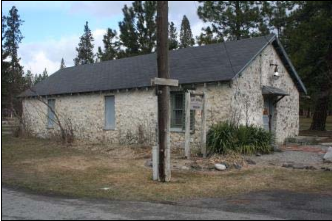
Figure 13: Fort George Wright, paint and oil storehouse
