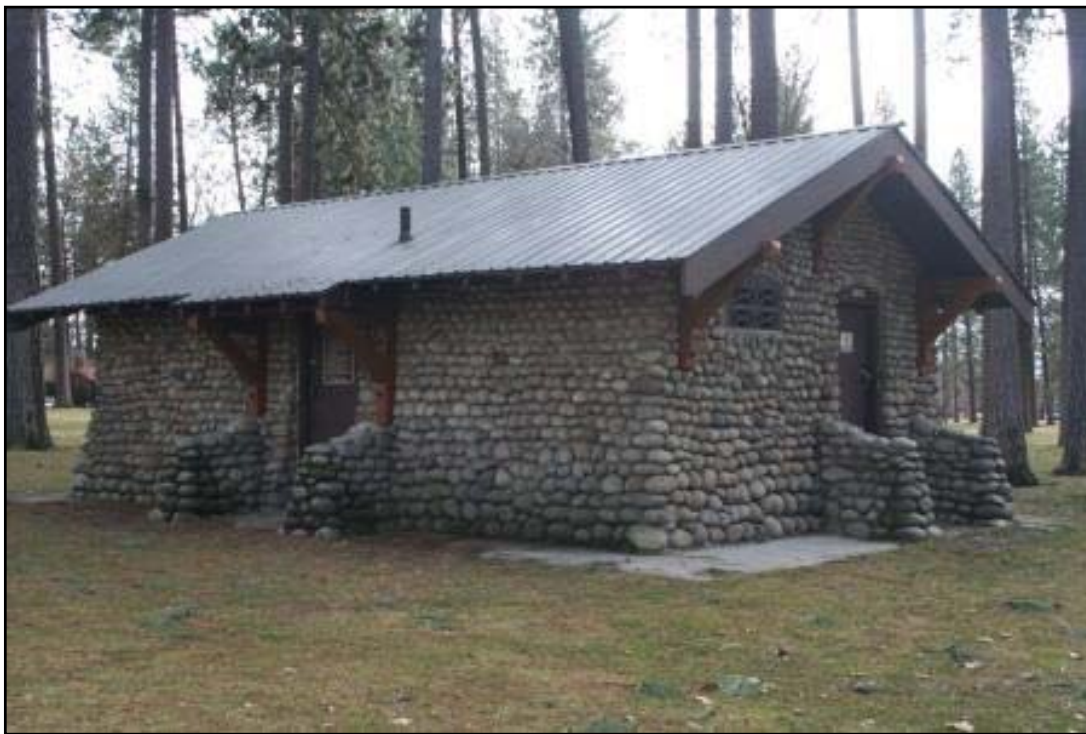
Figure 11: Audubon Park Restroom
