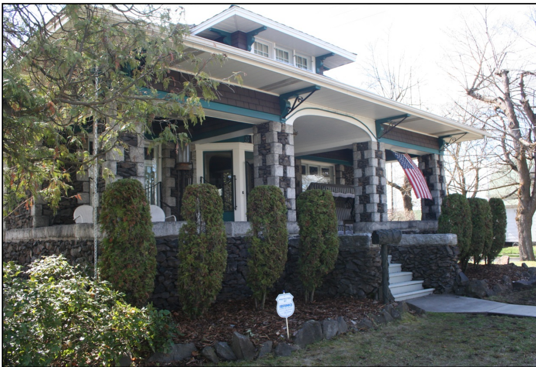
Figure 26: Stone house at 829 W. Mansfield Avenue
