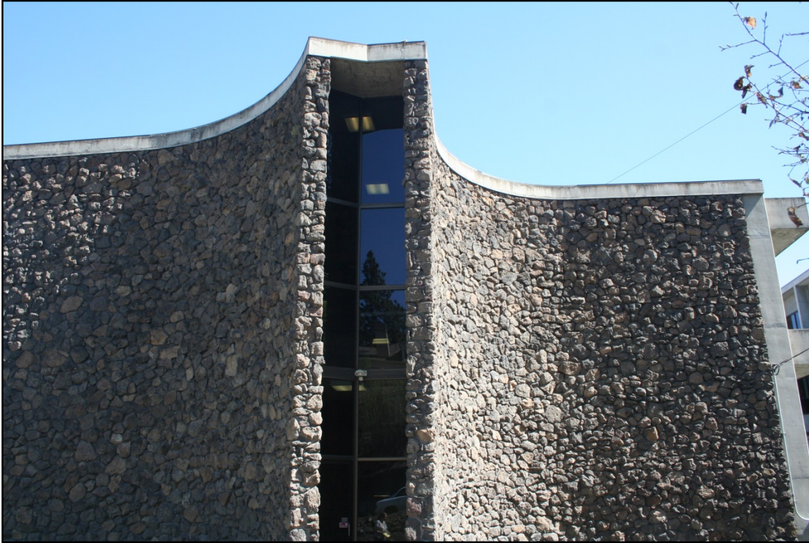
Figure 42: IBM Building, 799 and 801 S. Stevens Street
