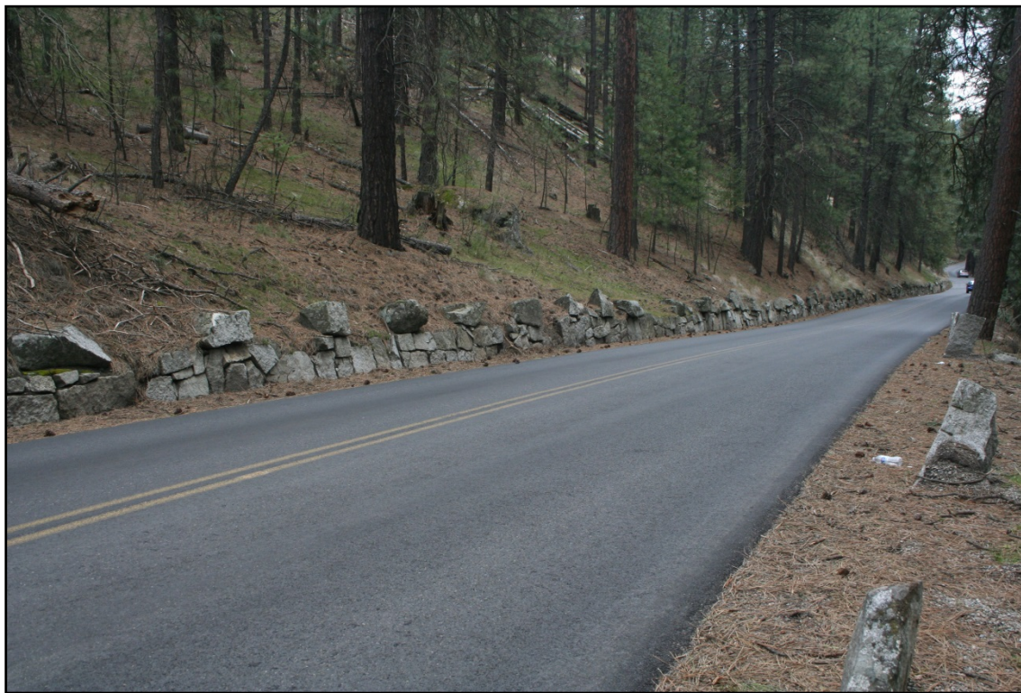
Figure 28: Rutter Parkway Stone Structures
