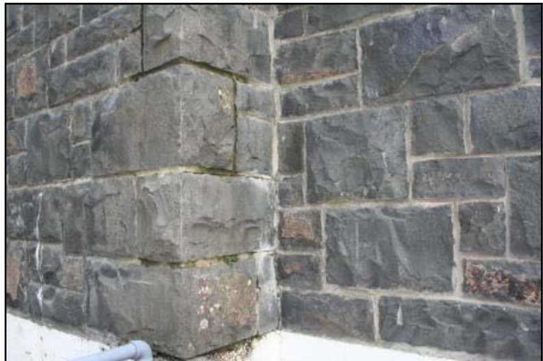
Figure 7: Hammer dressed basalt at Greystones on the Mukogawa Campus
