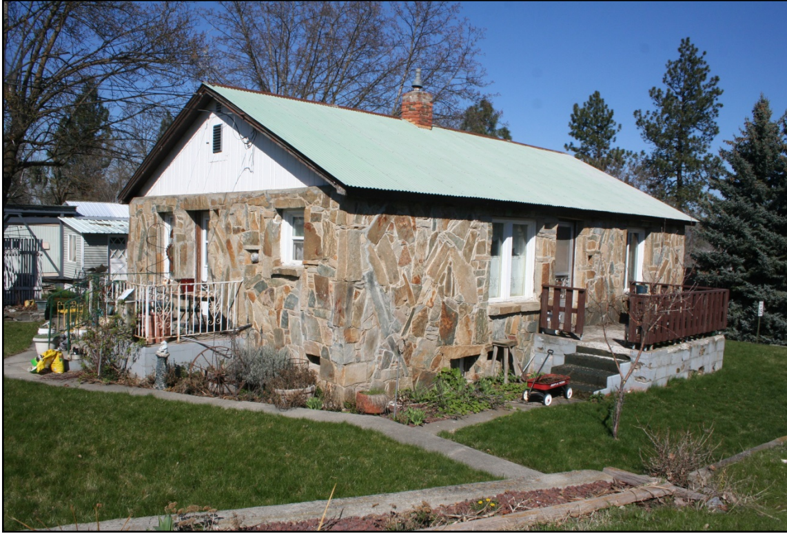
Figure 31: Stone House at 7408 E. 4th Avenue
