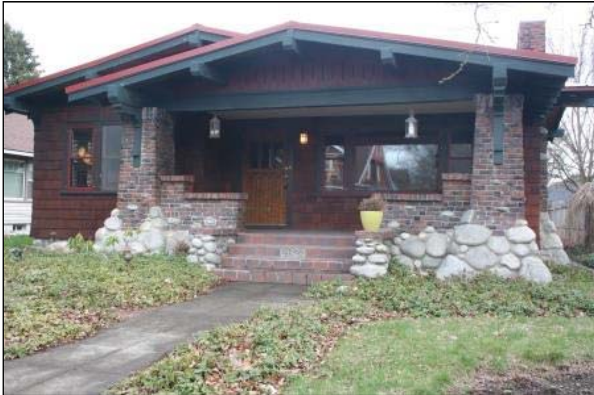
Figure 16: Peanut Brittle House at 2624 N. Wall Street, Spokane
