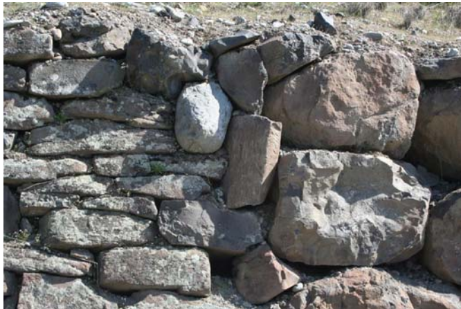
Figure 5: Aubrey White Parkway Rock Walls showing stone retaining wall, juxtaposition of original and poor repair
