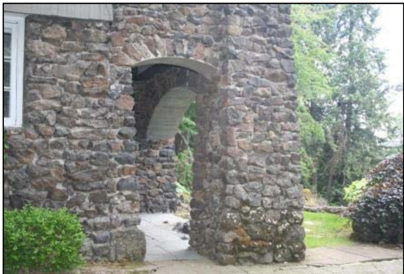
Figure 6: Basalt rubble construction at the Wilbur House, 2525 E. 19th Avenue, Spokane
