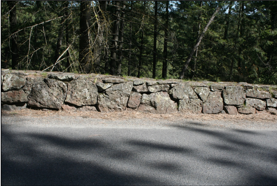
Figure 34: Aubrey White Parkway Rock Walls
