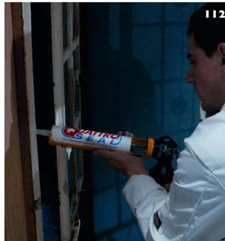
112: Silicone being injected into gaps between the frame and casement to exclude draughts. The casement is first painted with a releasing agent. The silicone is then left to cure with any excess trimmed back.
