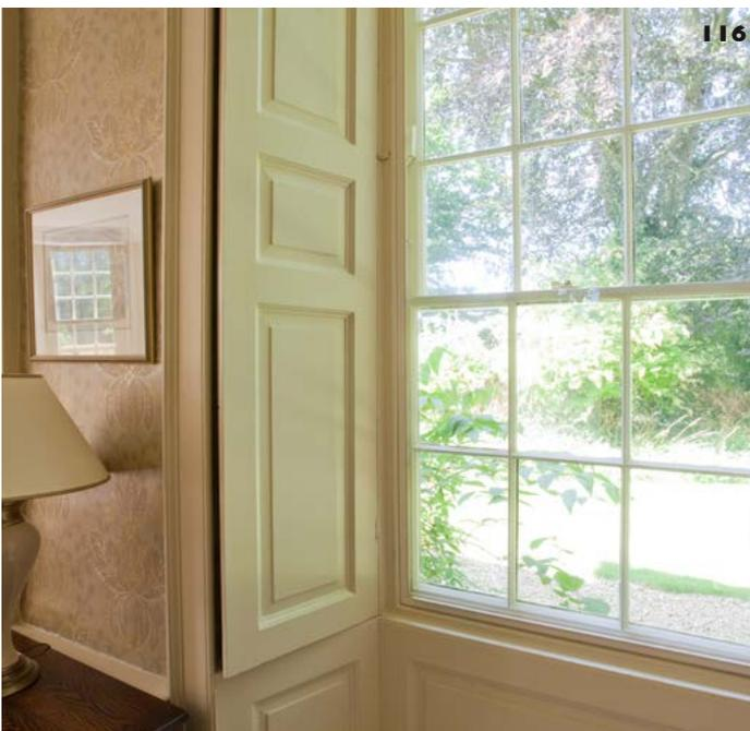
**115:** Failing plastic coated aluminium double glazed windows to this listed terrace house were replaced with single glazed timber casements to the correct historic pattern with secondary glazing incorporating Low E glazing giving a centre pane U-value of 1.6w/m<sup>2</sup>K.
