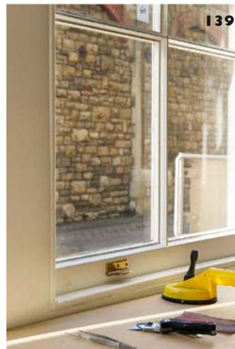
**125–139:** This sequence shows the addition of precision cut acrylic glazing to small paned windows. This allows the existing glazing to remain in place.
