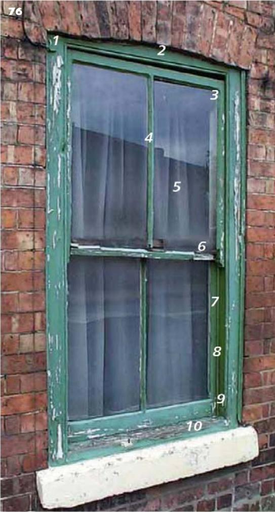
1. Holes drilled in frame for cable entry may admit water and cause decay
