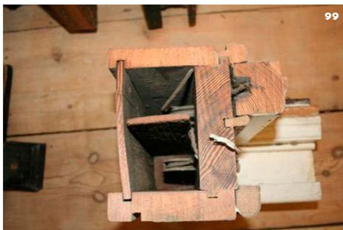
**99:** This section through a sash box shows the high quality of the timber used during the 19th century.
