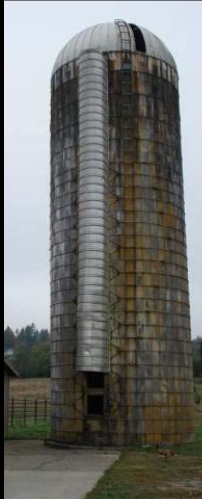
Concrete Stave Silo
