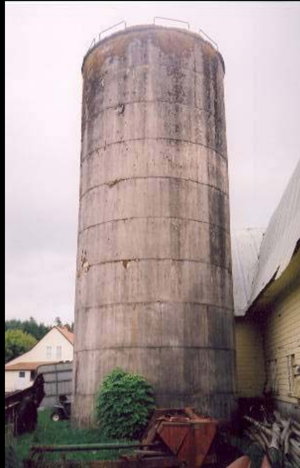
Poured Concrete Silo Grays Harbor Co. – c.1935
