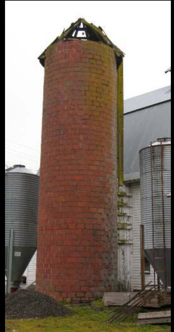
Glazed Tile Silo
