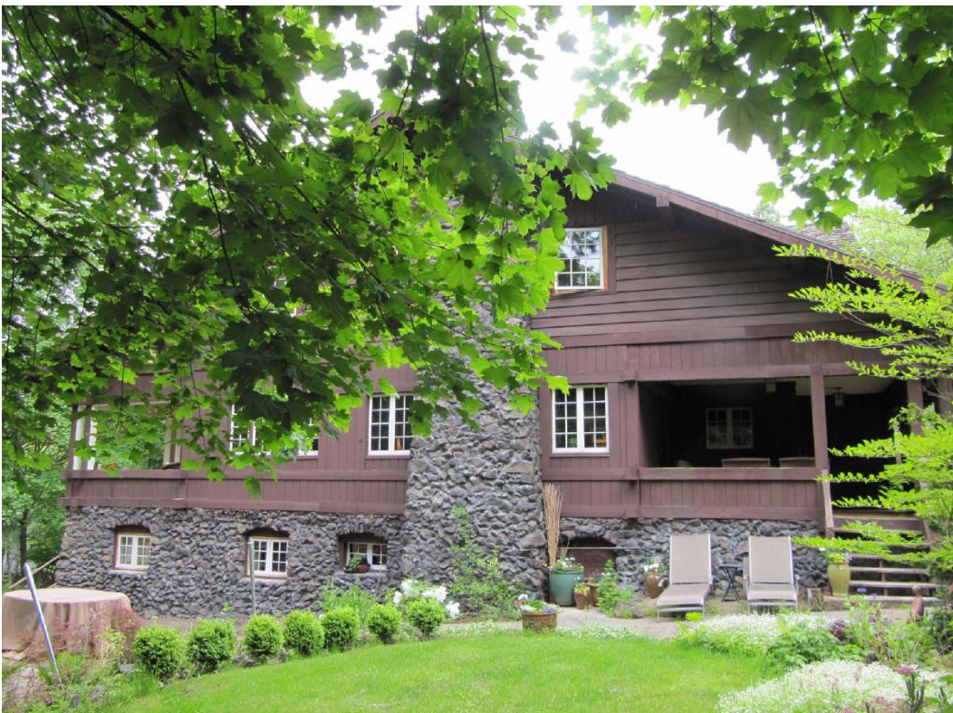
3 of 20: west face of house in 2014
