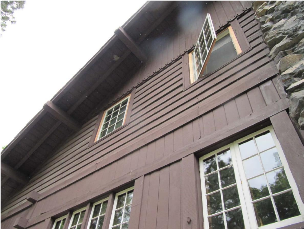
4 of 20: west gable peak detail
