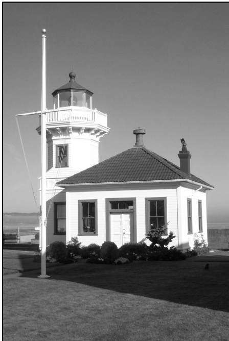
Figure 4: Light Station, Mukilteo.
