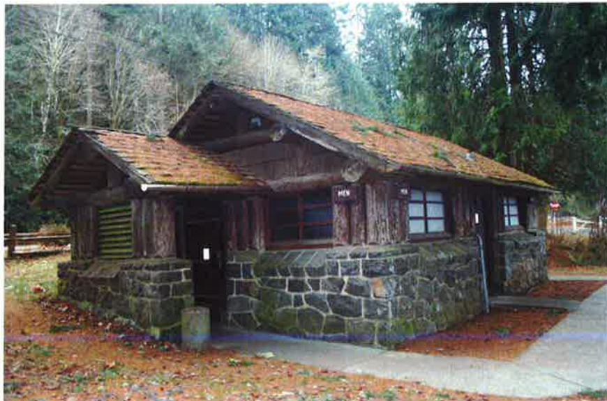
TSP37: Building 7 (comfort station #2), north and east elevations, looking southwest.
