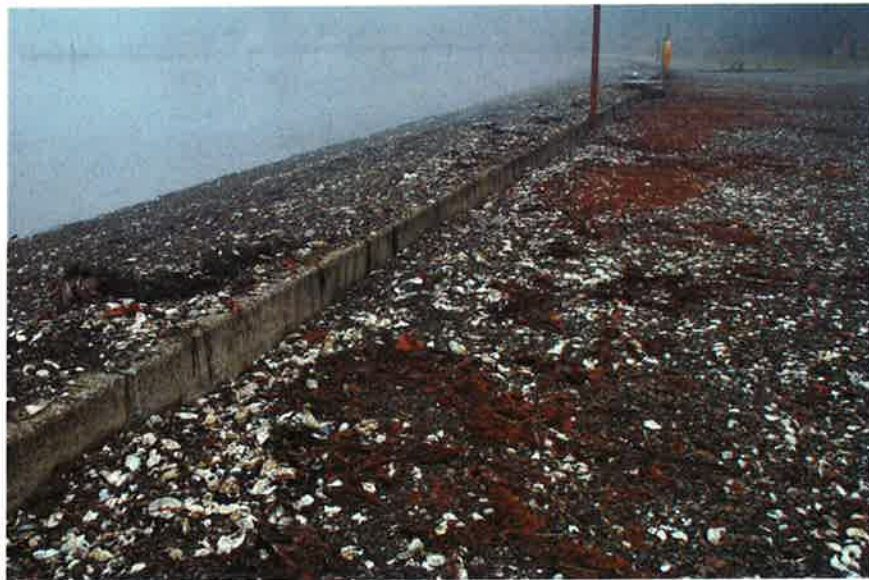
TSP52: Seawall, looking east.
