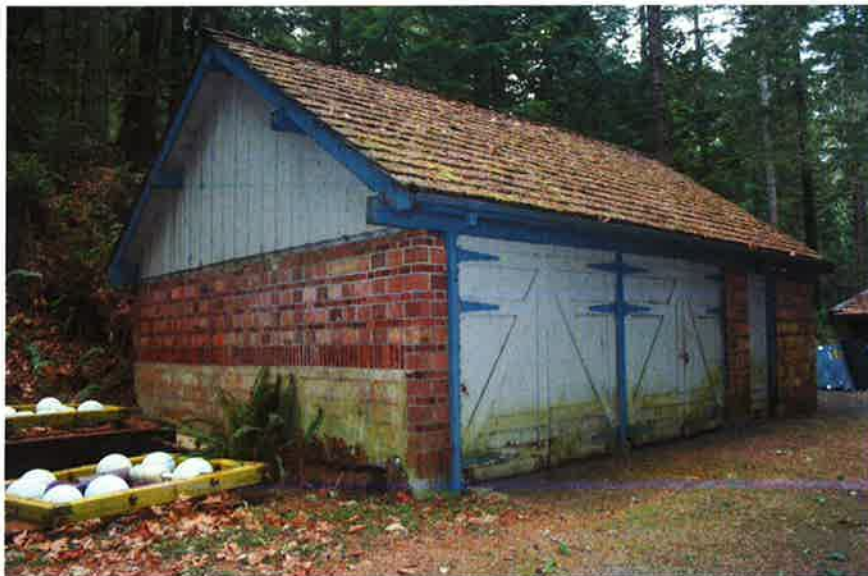
TSP77: Building 3 (garage/shop), north and east elevations, looking southwest.
