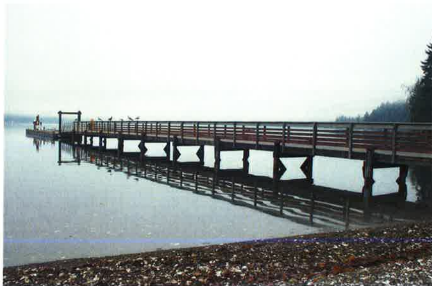
TSP61: Pier and dock, west elevation, looking northeast.
