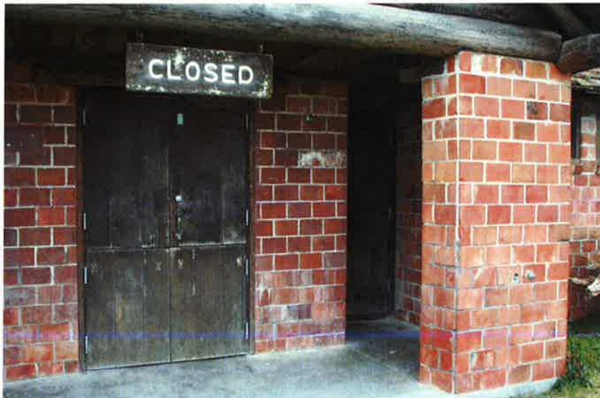
TSP57: Building 5 (bathhouse #2), entry detail, looking southwest.
