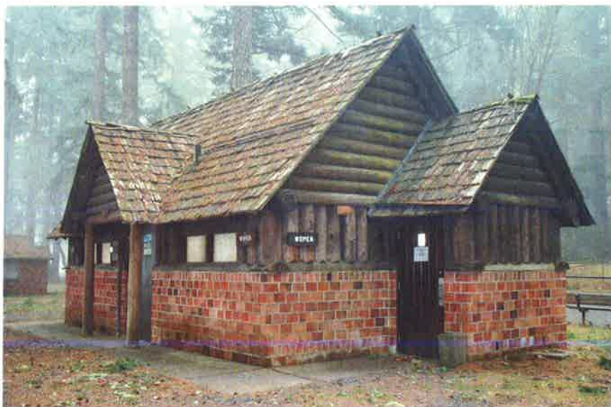
TSP51: Building 6 (comfort station #1), north and west elevations, looking southeast.
