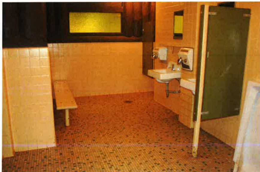
TSP71: Building 8 interior, looking southwest
