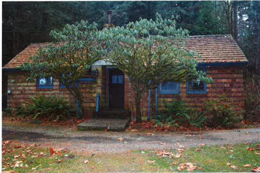
TSP72: Building 1 (superintendent's house), north (front) elevation, looking south.
