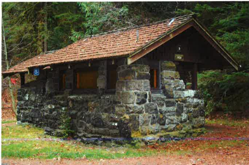
TSP65: Building 9 (comfort station #4), west and south elevations, looking northeast.
