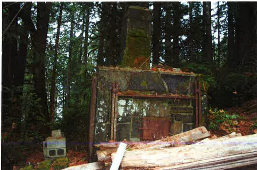
TSP79: Incinerator, west elevation, looking east.
