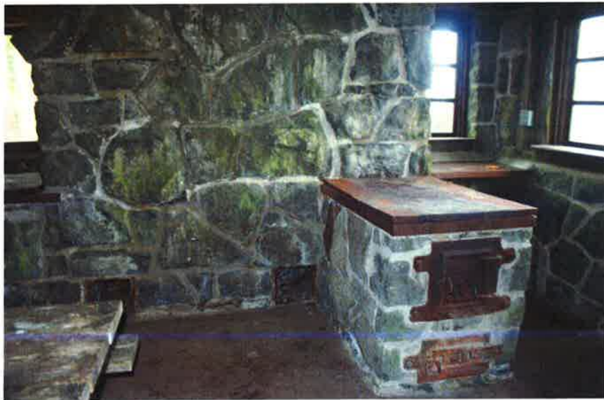
TSP43: Building 11 (shelter kitchen), interior, stove, looking north.
