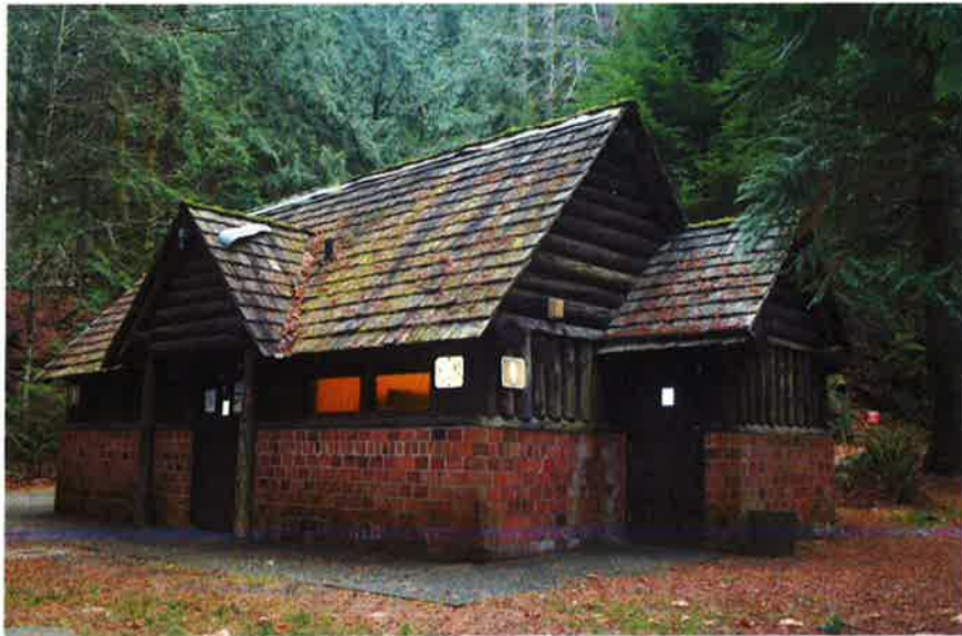
TSP69: Building 8 (comfort station #3), north and west elevations, looking southeast.
