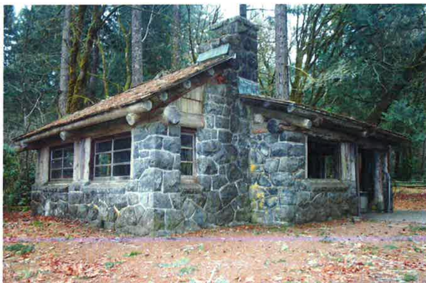
TSP41: Building 11 (shelter kitchen), northwest and northeast elevations, looking south.
