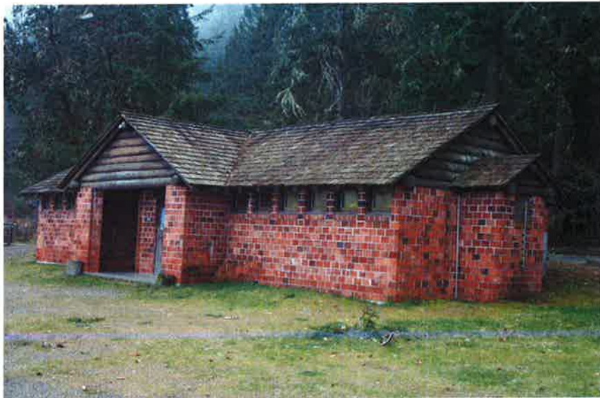
TSP59: Building 4 (bathroom #1), north and west elevations, looking southeast.
