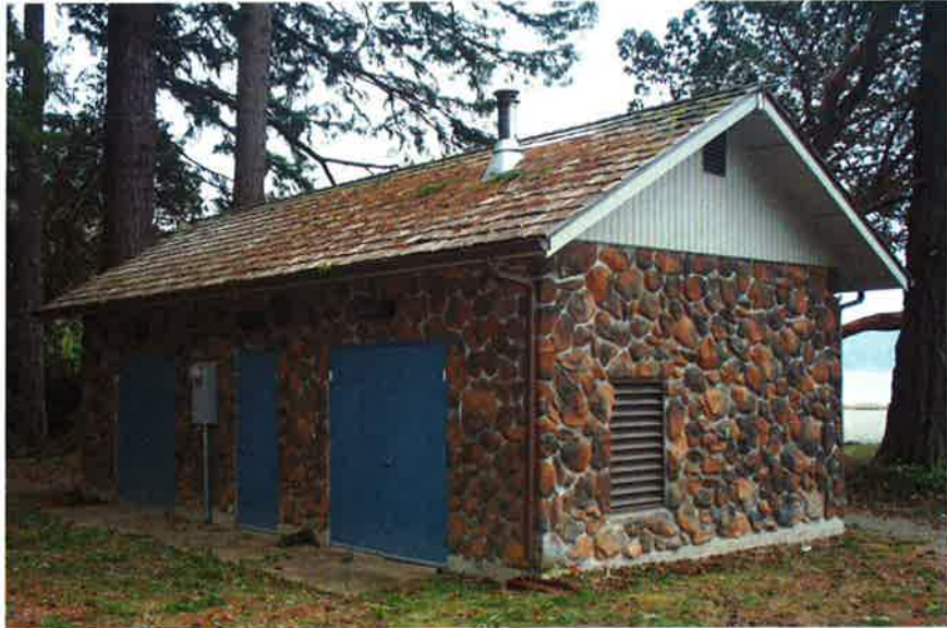
TSP38: Pump house, northeast and southeast elevations, looking west.
