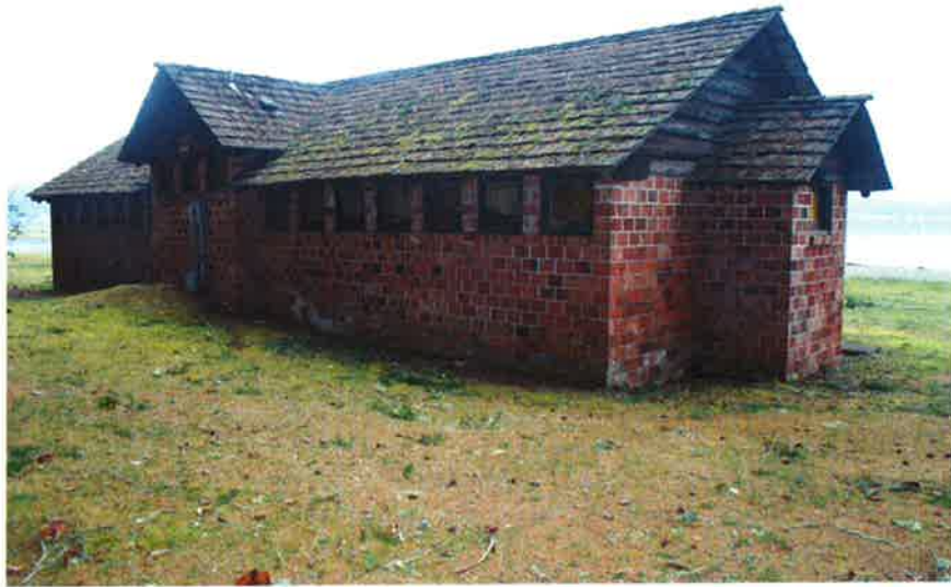
TSP58: Building 5 (bathroom #2), south and east elevations, looking northwest.
