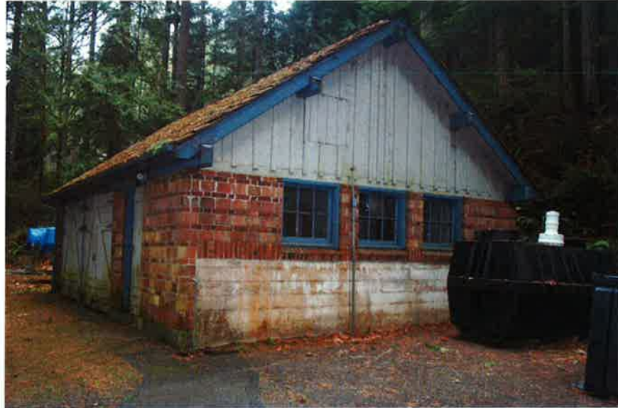
TSP76: Building 3 (garage/shop), west and north elevations, looking southeast.
