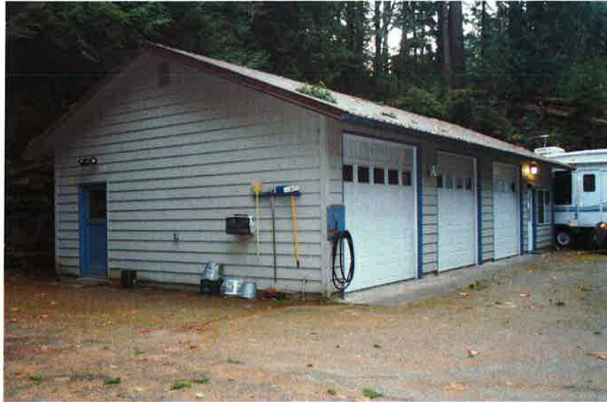
TSP78: Building 25 (modern office/garage), north and east elevations, looking southwest.
