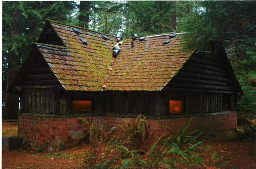
TSP70: Building 8 (comfort station #3), south and east elevations, looking northwest.
