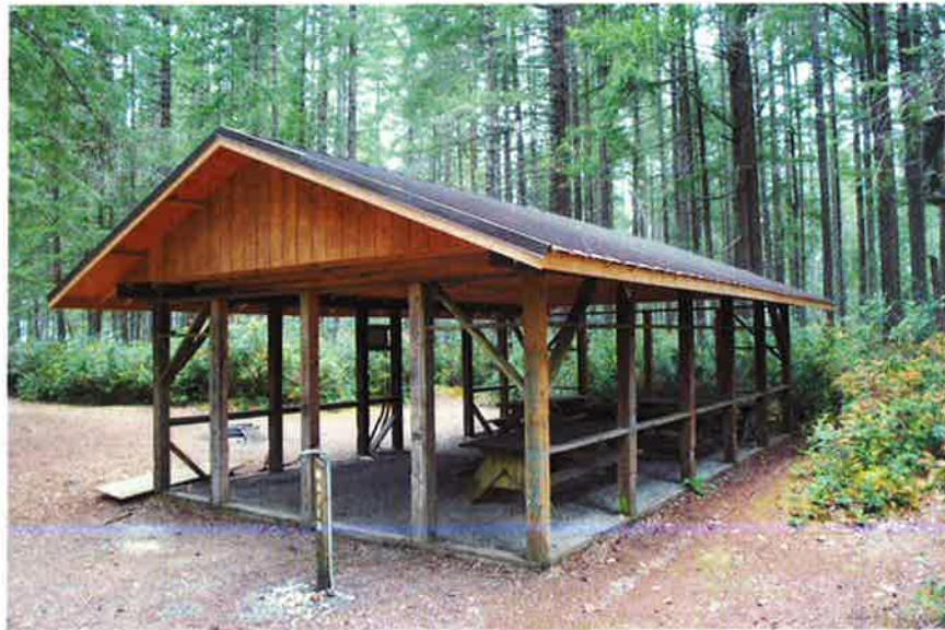
TSP81: Building 20 (group camp shelter), north and west elevations, looking southeast.
