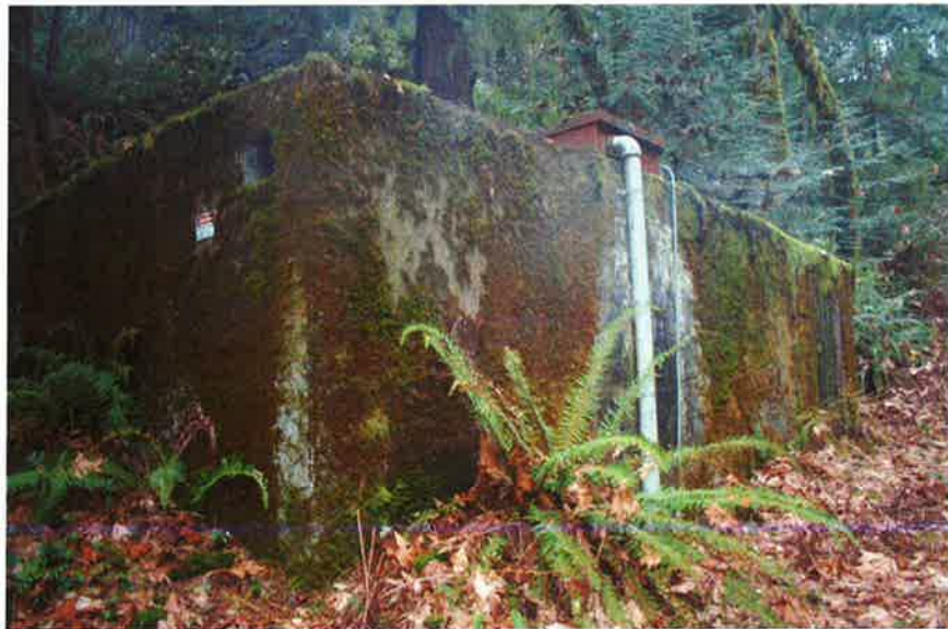
TSP67: Water storage reservoir, north and west elevations, looking southeast.
