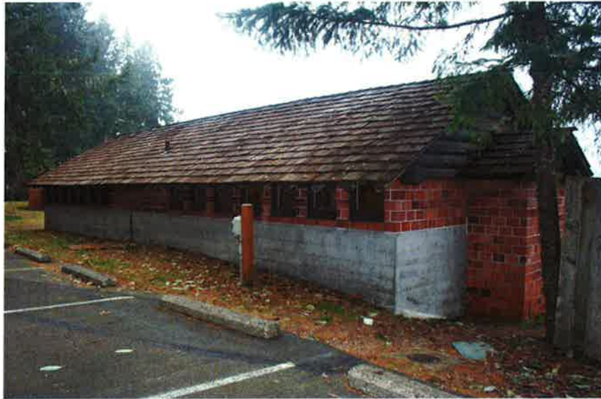
TSP60: Building 4 (bathhouse #1), south and east elevations, looking northwest.
