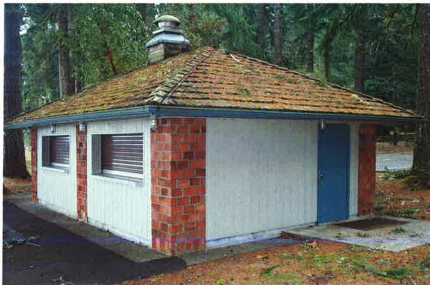
TSP55: Building 16 (concession), north and west elevations, looking southeast.
