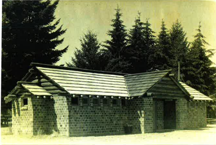
TSP15: Building 5 (bathhouse #2).
