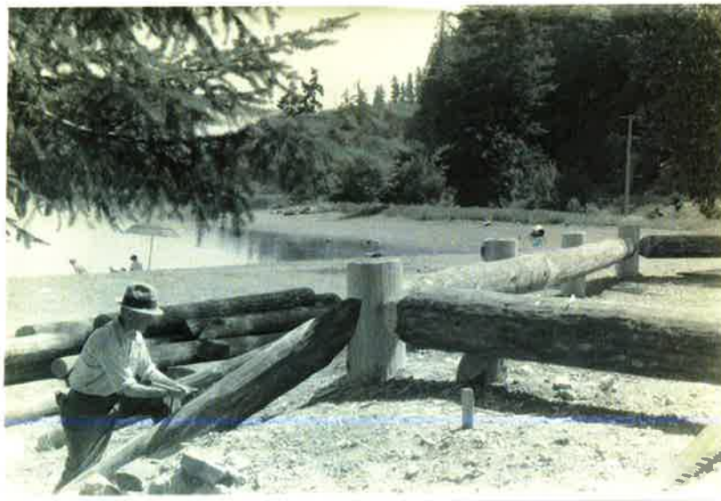
TSP14: Enrollee working on guard rails.
