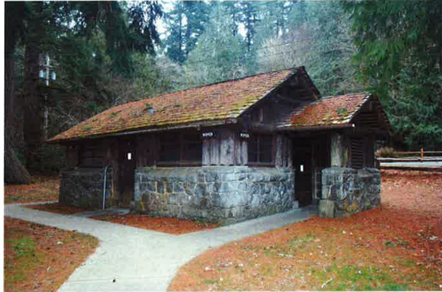
TS36: Building 7 (comfort station #2), north and west elevations, looking southeast.
