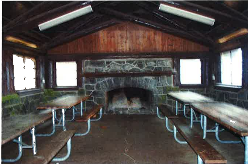
TSP48: Building 10 (community kitchen), interior, west end fireplace, looking west.
