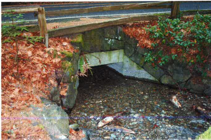
TSP63: Highway culvert, north elevation, looking southwest.
