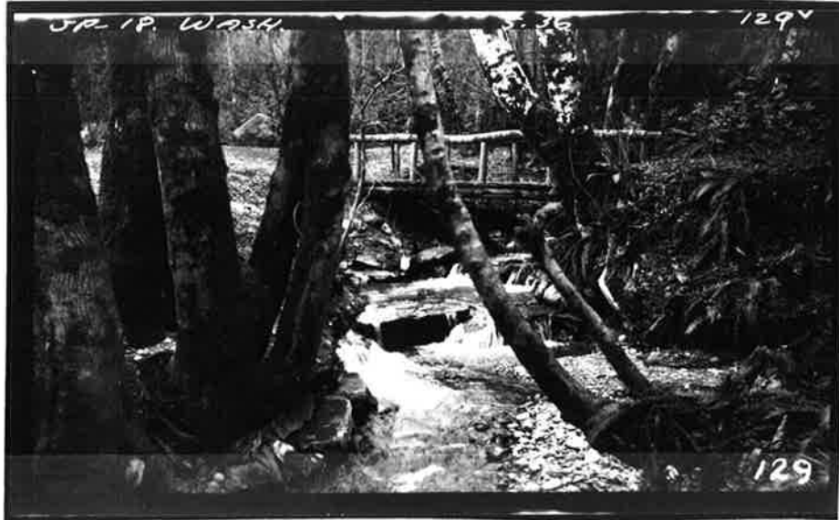
TSP7: Footbridge over Twanoh Creek.
