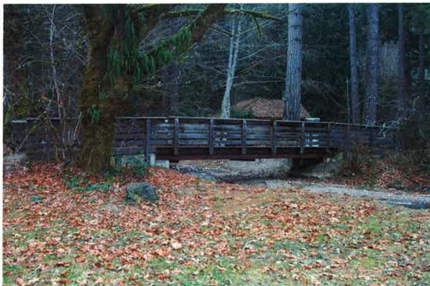
TSP40: Lower footbridge, north elevation, looking southwest.
