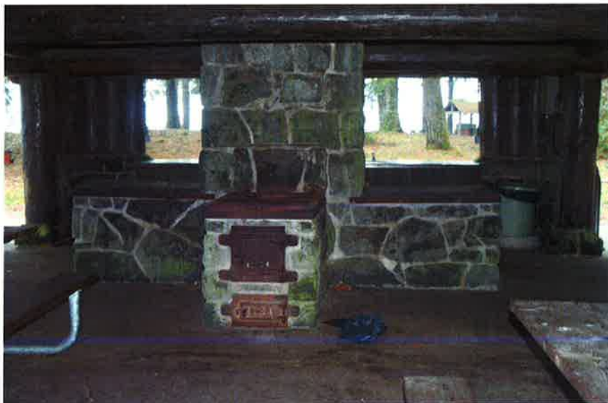
TSP49: Building 10 (community kitchen), interior, stoves, looking east.
