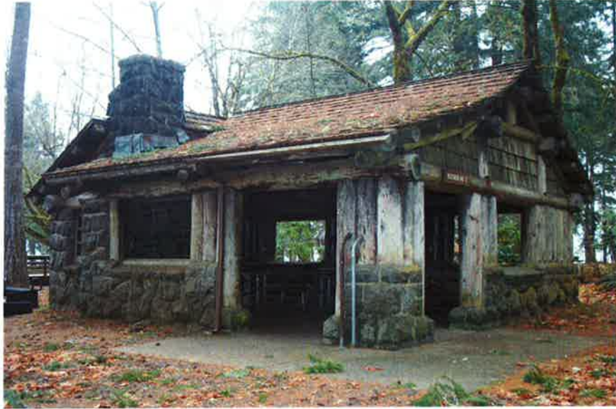
TSP42: Building 11 (shelter kitchen), southwest and southeast elevations, looking north.
