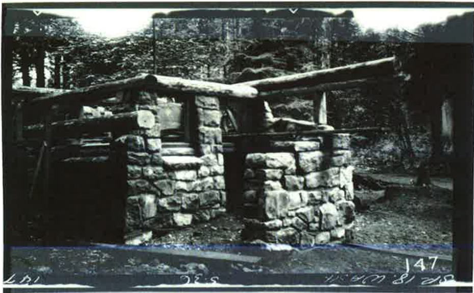
TSP10: Building 9 (comfort station #4) under construction.
