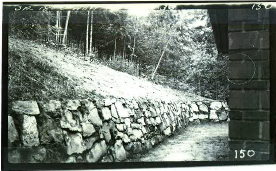
TSP11: Stone retaining wall behind superintendent's house.
