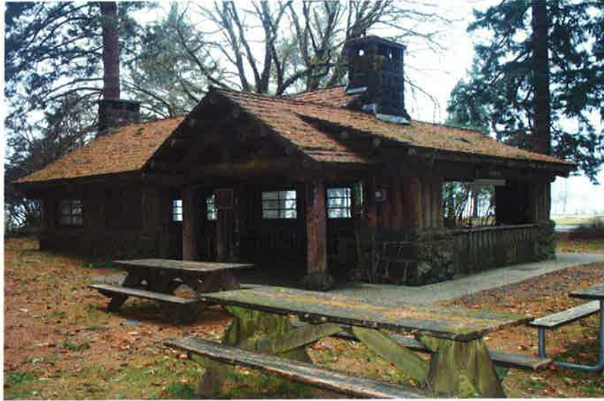
TSP46: Building 10 (community kitchen), south and east elevations, looking northwest.
