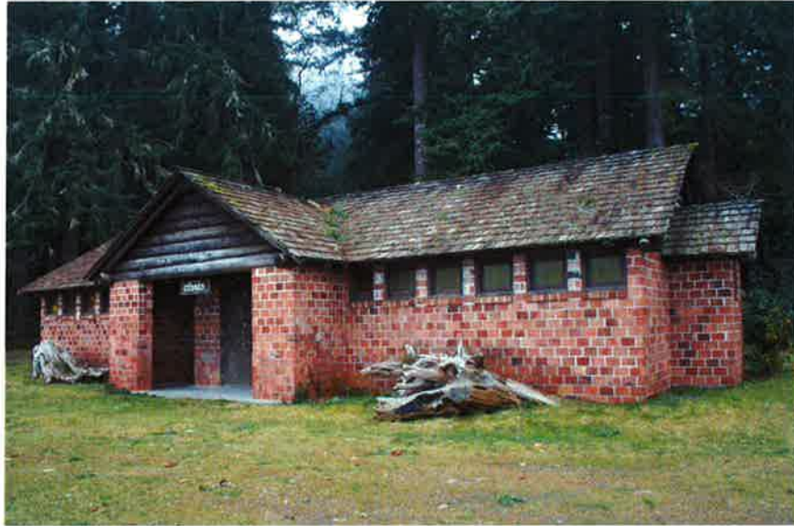
TSP56: Building 5 (bathhouse #2), north and west elevations, looking southeast.
