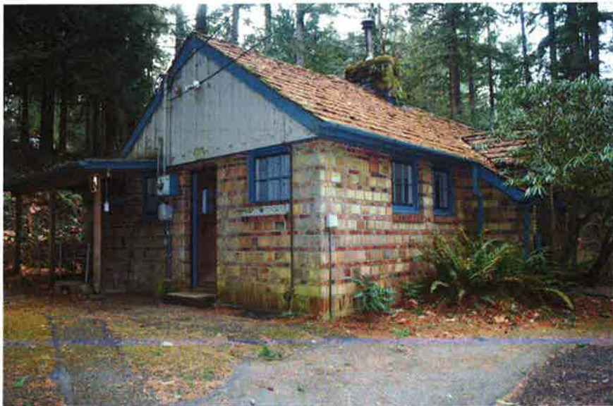
TSP73: Building 1 (superintendent's house), north and east elevations, looking southwest.
