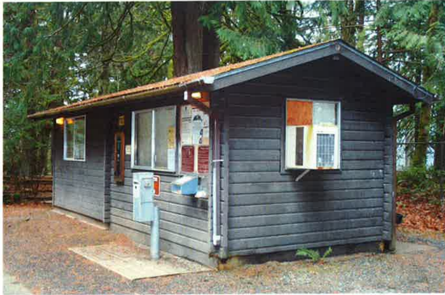
TSP62: Ranger's office, south and east elevations, looking northwest.
