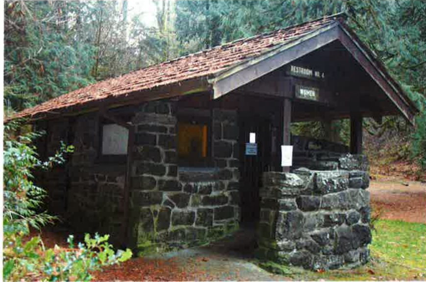
TSP66: Building 9 (comfort station #4), east and north elevations, looking southwest.
