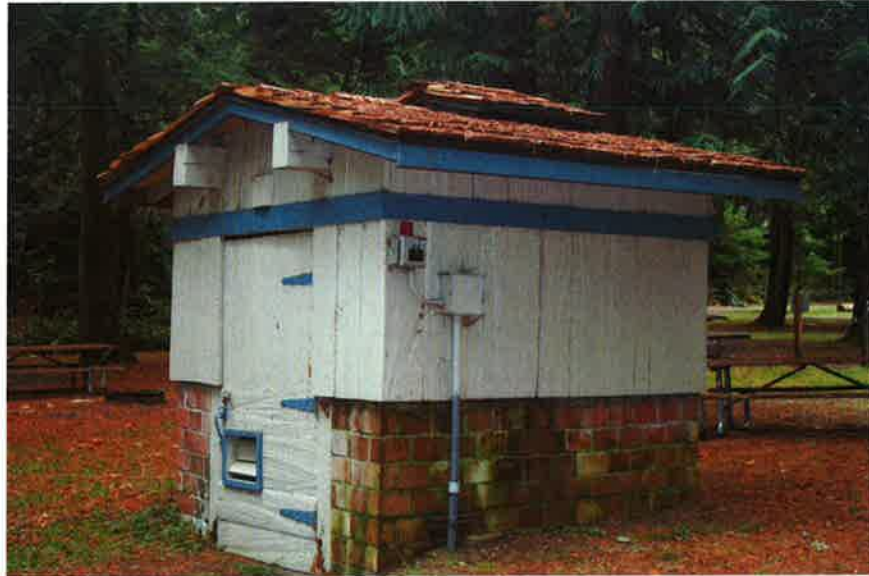
TSP64: Upper campground pump house, north and west elevations, looking southeast.
