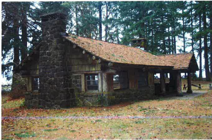
TSP47: Building 10 (community kitchen), south and west elevations, looking northeast.
