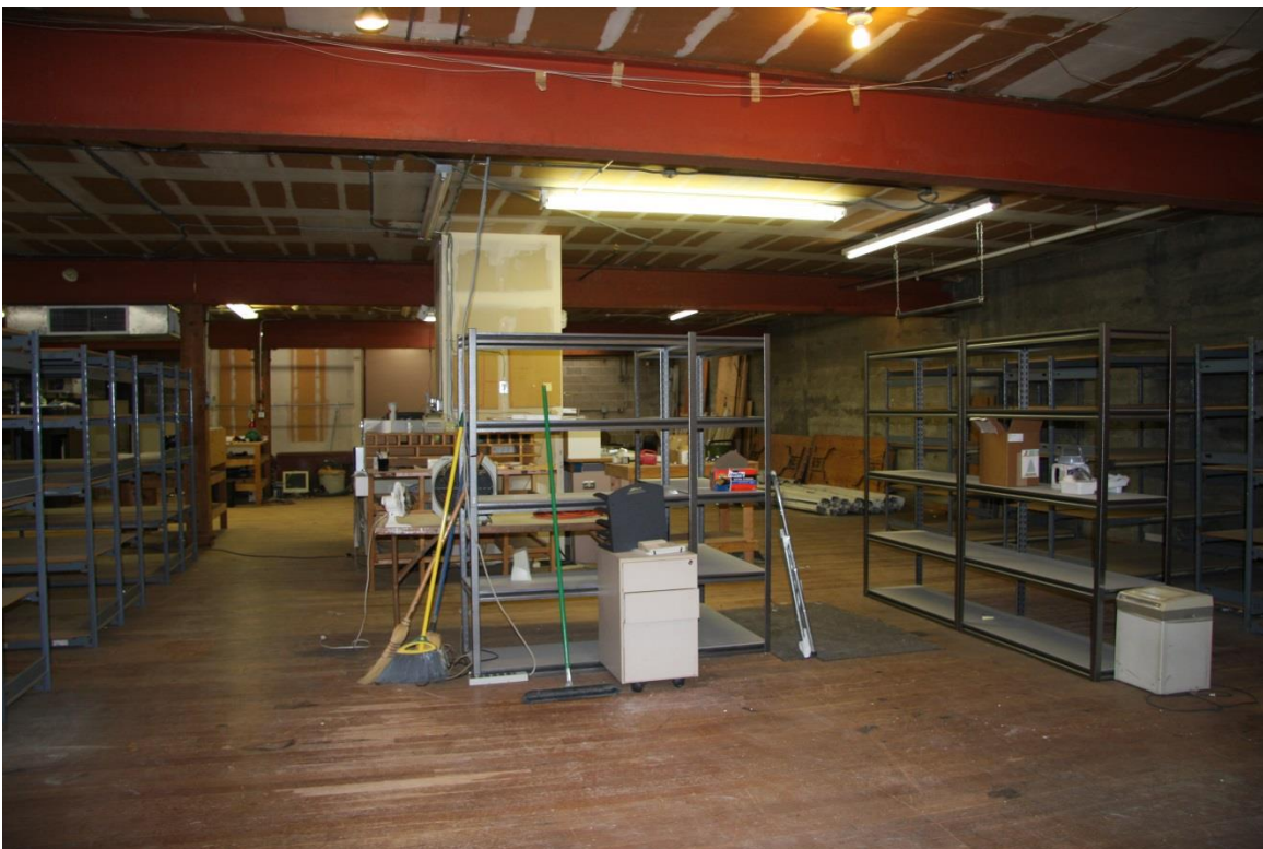
Photo #13 of 15 (WA_PierceCounty_RentonWoolworthBld_0013) Second floor interior, storage room, south (left) and west (right) elevations, camera facing southwest
