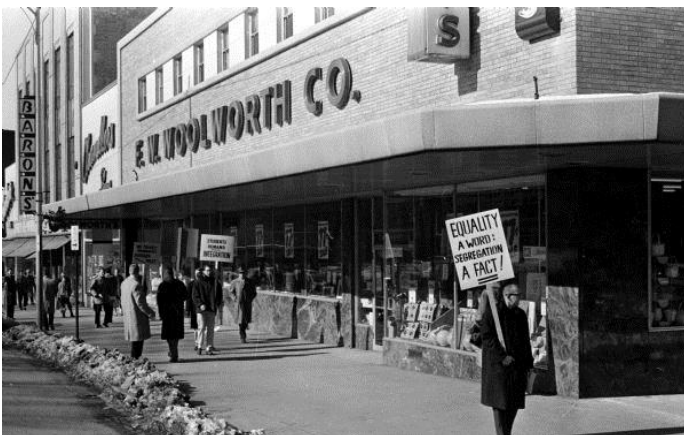
Madison, WI – Woolworth Co. Store (built 1954)
