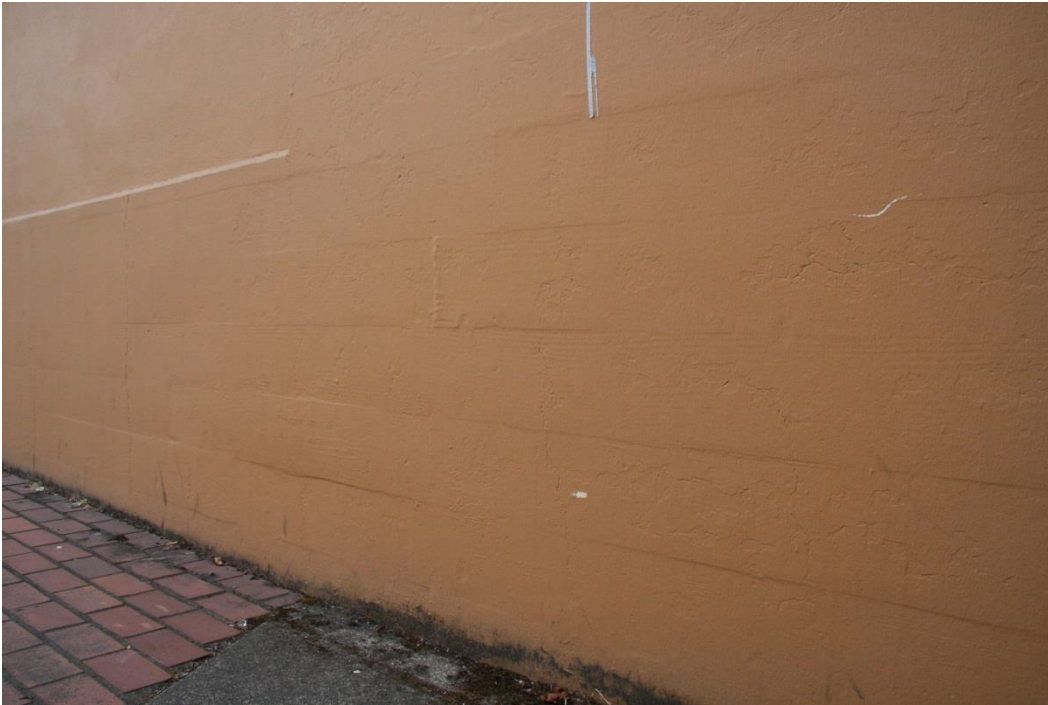
Photo #6 of 15 (WA_PierceCounty_RentonWoolworthBld_0006) East elevation detail, camera facing west
