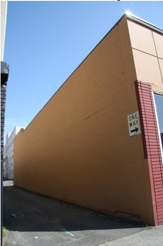
Photo #7 of 15 (WA_PierceCounty_RentonWoolworthBld_0007) West elevation, camera facing northeast
