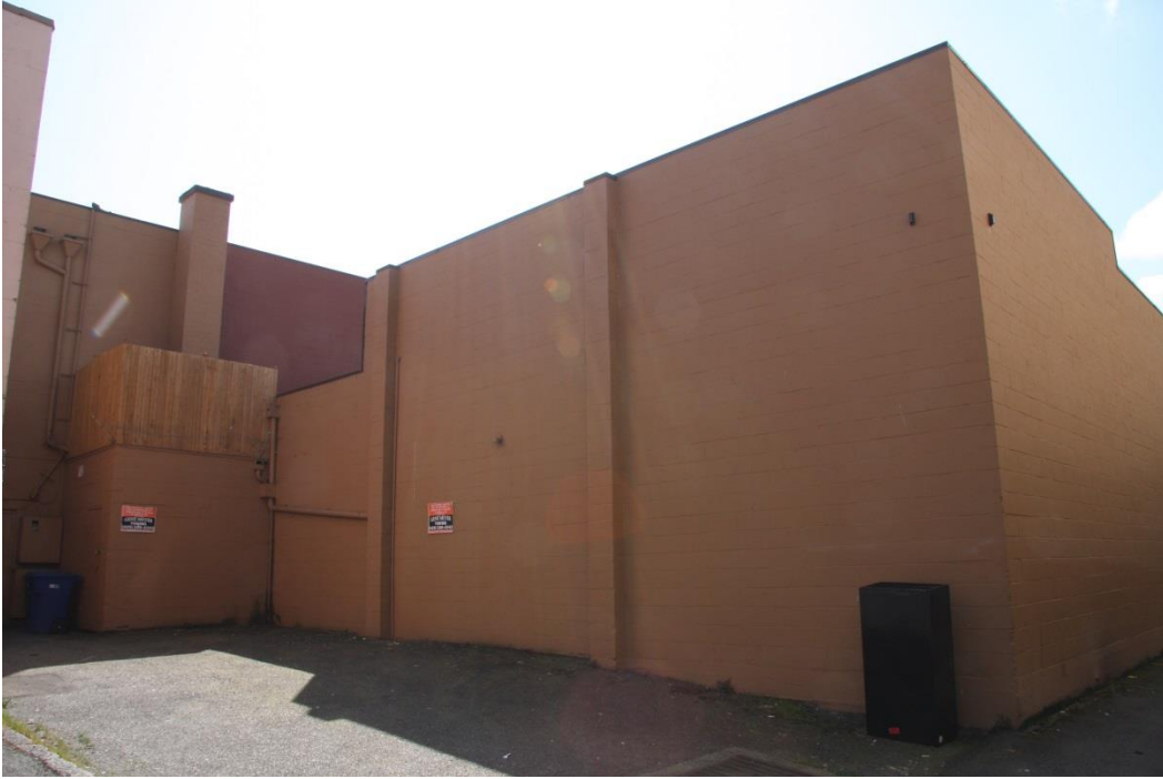
Photo #8 of 15 (WA_PierceCounty_RentonWoolworthBld_0008) North elevation, camera facing southeast
