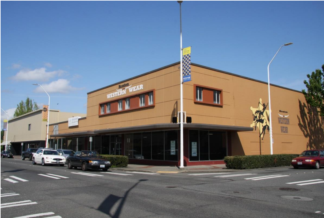
Photo #1 of 15 (WA_PierceCounty_RentonWoolworthBld_0001) South façade (left) and east elevation (right), camera facing northwest
