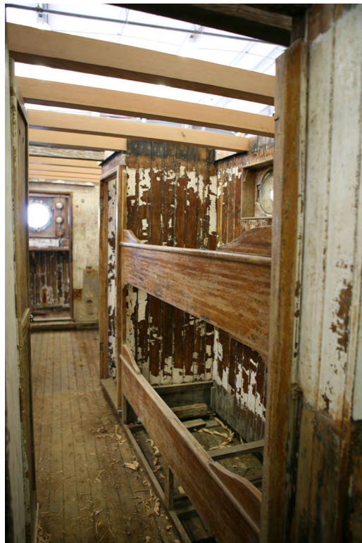
10 of 20. Western Flyer. Deckhouse, looking forward along corridor. Two crew bunks at right (starboard side). Wheelhouse in the distance at left.
