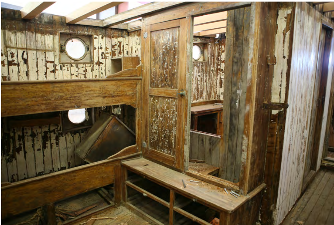
11 of 20. Western Flyer. Deckhouse, looking to port. Crew bunks along port (left) side of corridor. Closet doors, center. captain's cabin visible through (former) closet.
