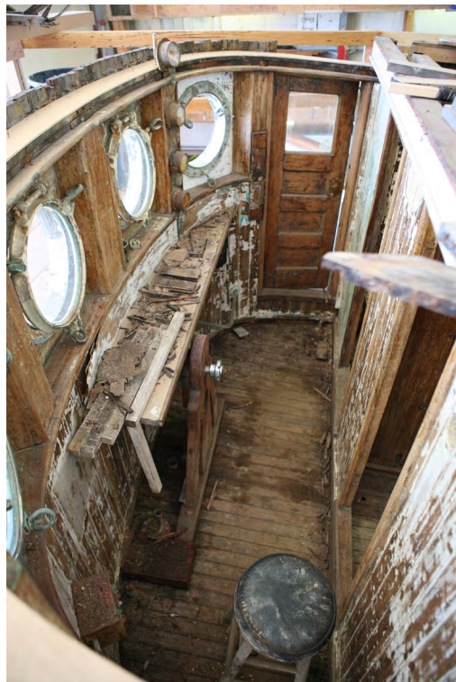
14 of 20. Western Flyer. Deckhouse, looking down into wheelhouse from scaffolding. Looking from port to starboard. Wheel has been temporarily removed during renovation.
