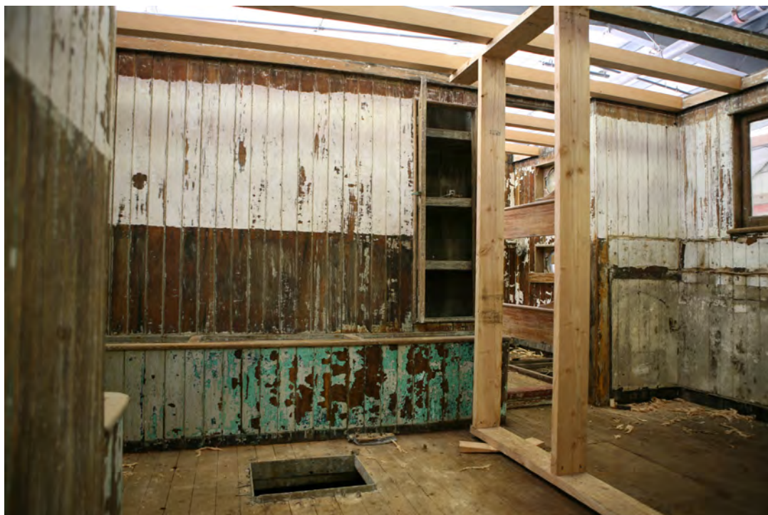
8 of 20. Western Flyer. Looking forward, into galley. Built-in bench seating at left. Former location of sink and stove at right.
