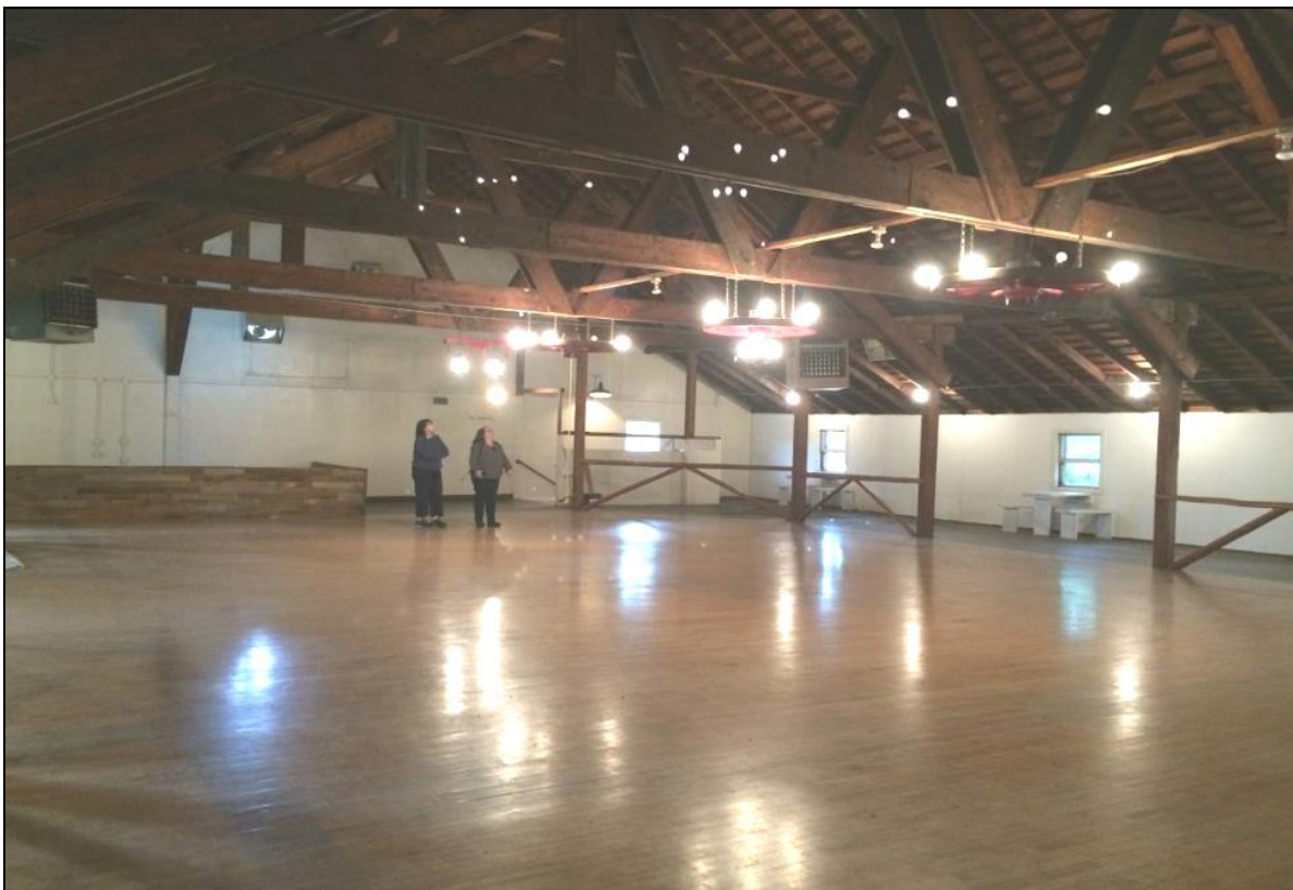
Figure 19. H.L. Wolf Feed & Implement Warehouse, interior upstairs.
