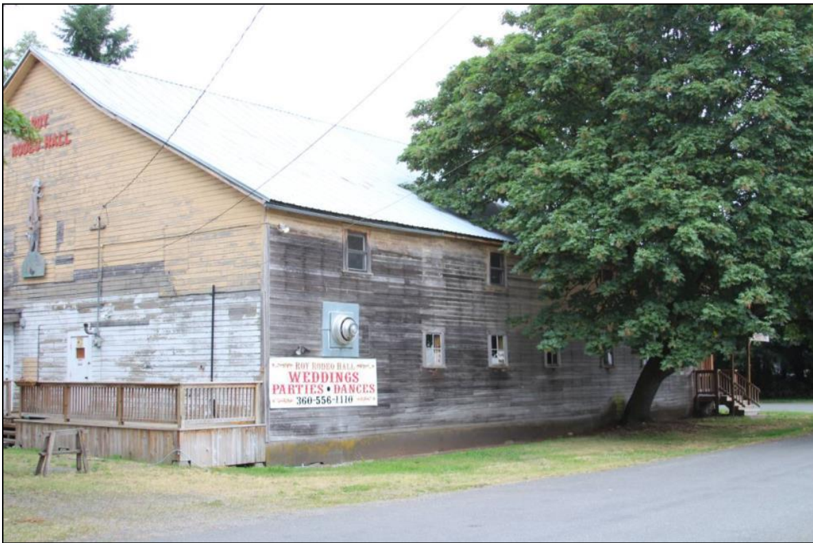
Figure 16. H.L. Wolf Feed & Implement Warehouse, south aspect, looking northwest. Photo from First Street.
