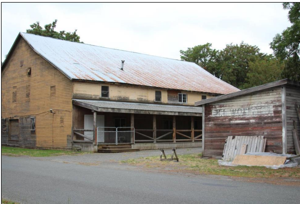
Figure 13. H.L. Wolf Feed & Implement Warehouse, north aspect and east aspect, view to the southwest. Low shed in foreground is the location of the former H.L. Wolf wellhouse. Photo from Peterson Street.
