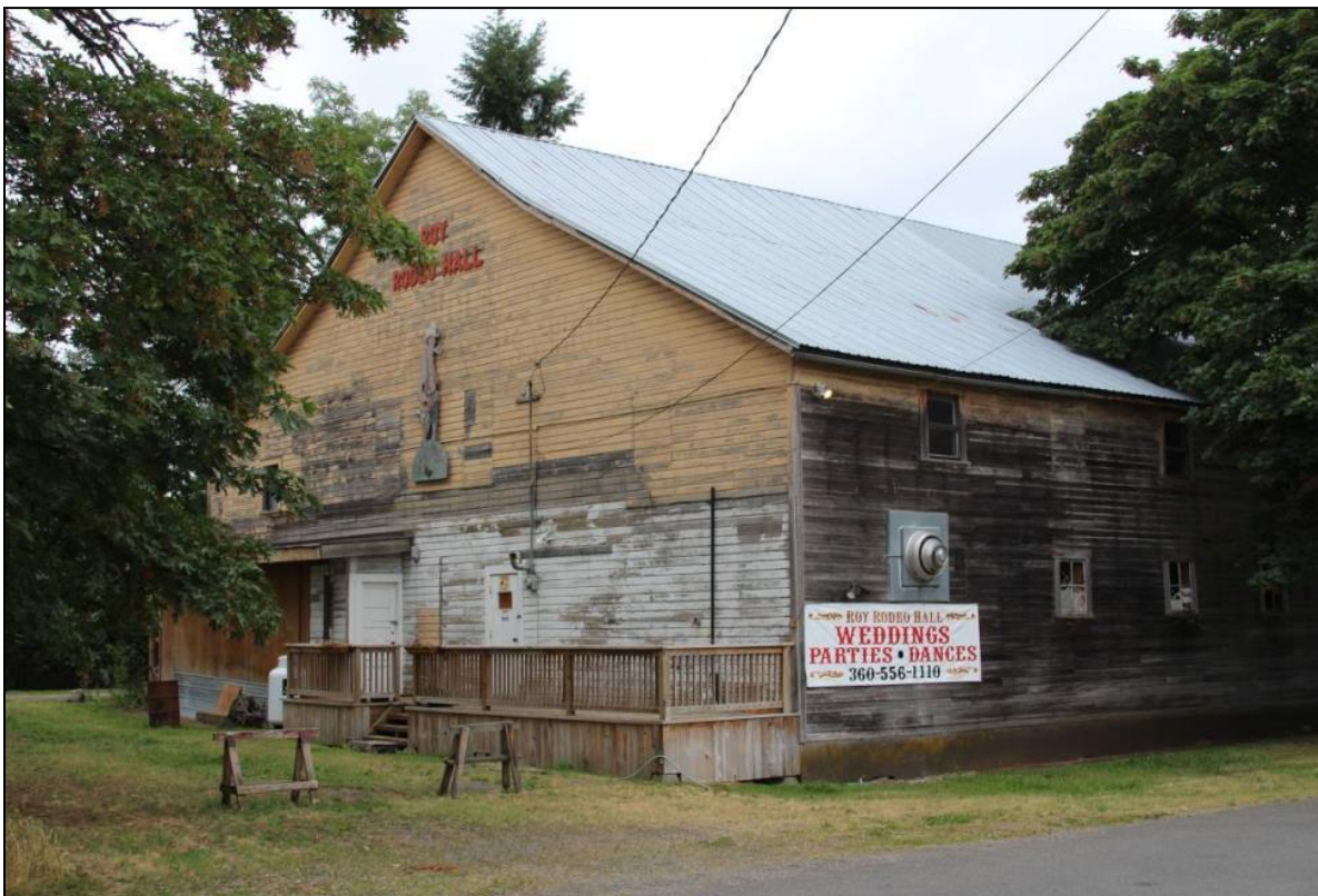
Figure 17. H.L. Wolf Feed & Implement Warehouse, west aspect, showing south aspect. View to the northwest. Photo from First Street.
