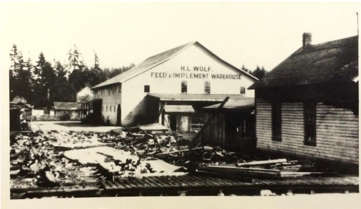
Figure 22. H.L. Wolf Feed & Implement Warehouse (1932). Nominated building.
