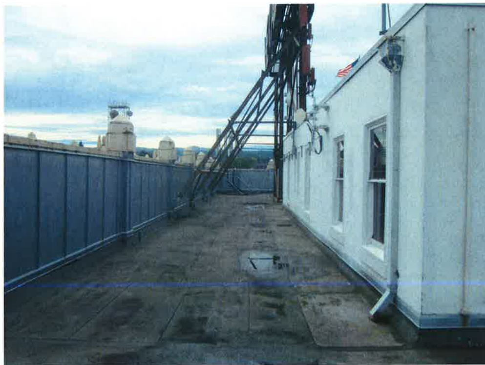
Photograph 18 of 18: View of roof, looking southeast.
