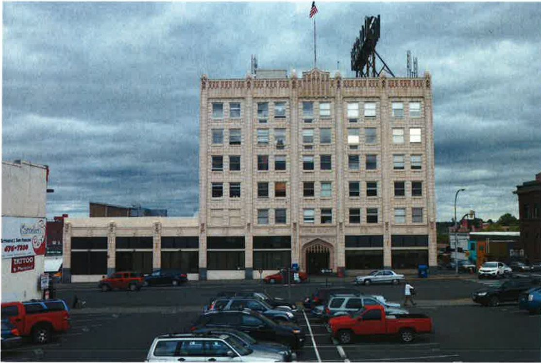
Photograph 1 of 18: View of southeast facade.
