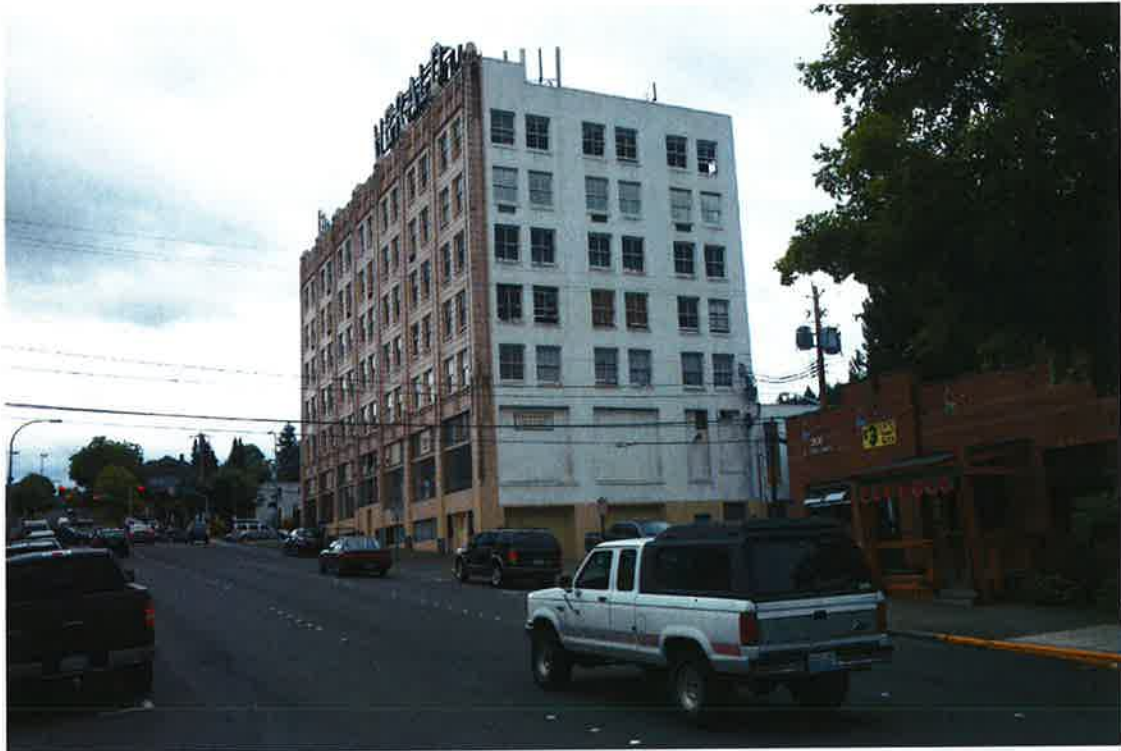
Photograph 3 of 18: View of northeast and northwest facades.
