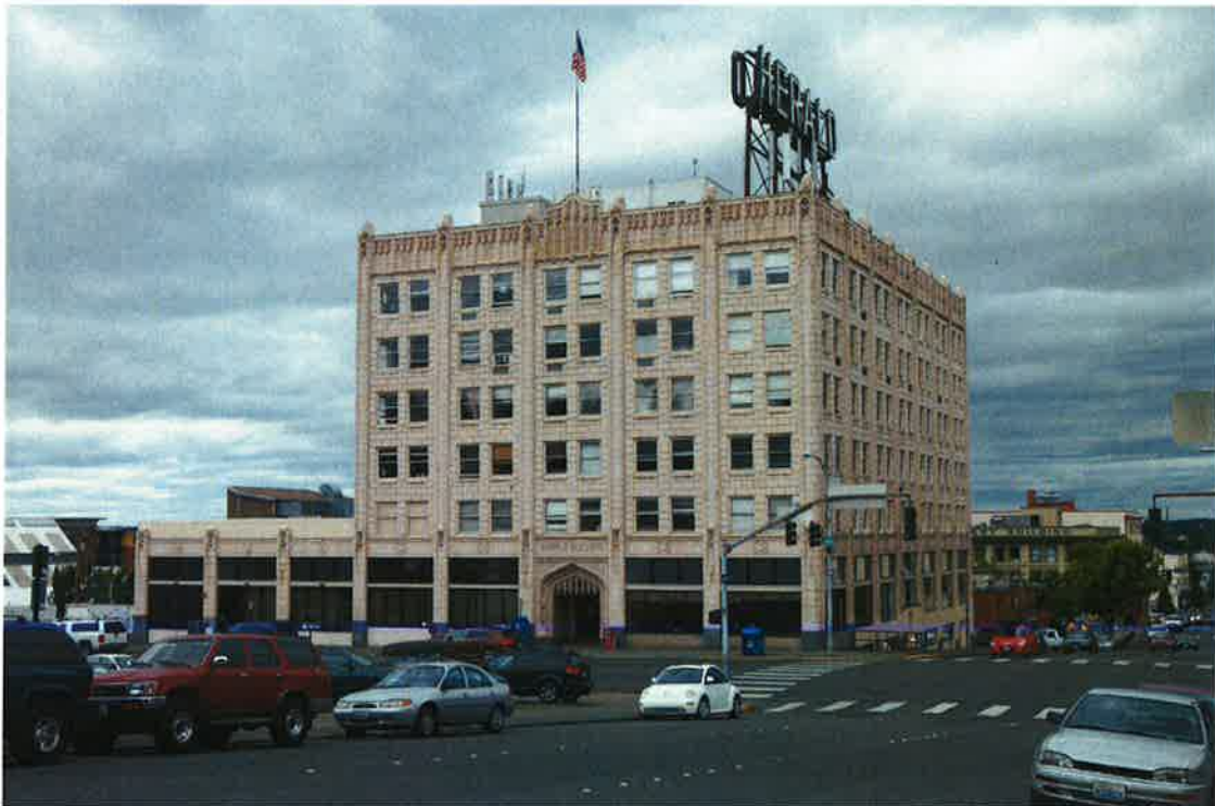
Photograph 2 of 18: View of southeast and northeast facades.
