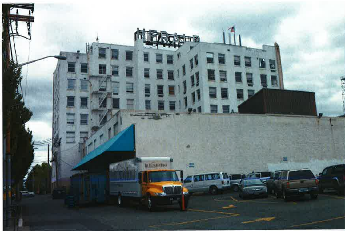
Photograph 4 of 18: View of southwest facade.
