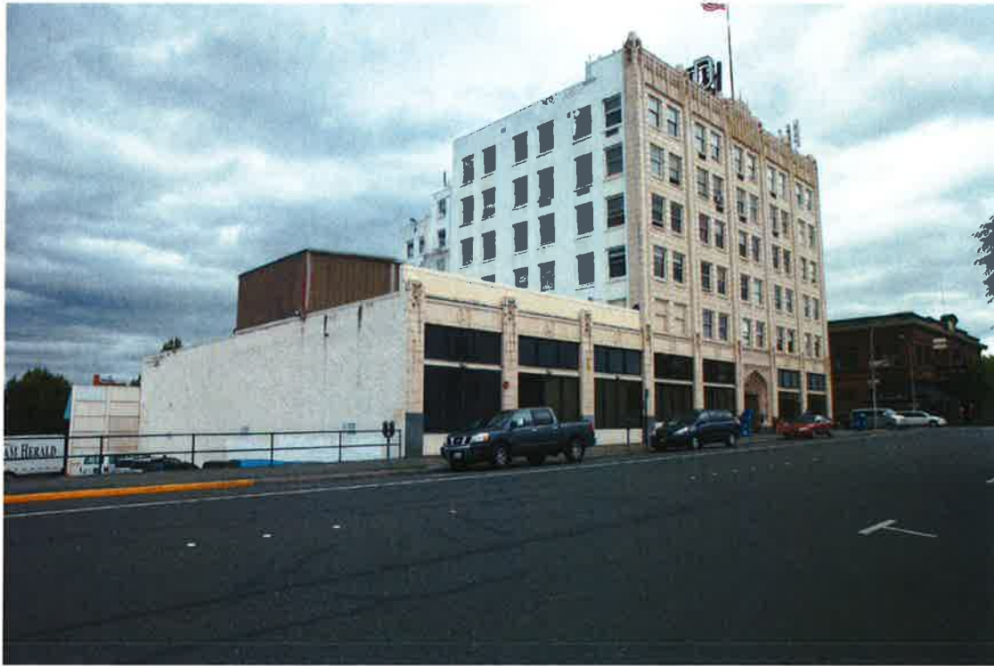
Photograph 5 of 18: View of southwest and southeast facades.
