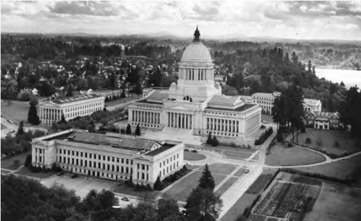
2. 1940s to 1950s view of the capitol group looking southeast. Source: Washington State Archives
