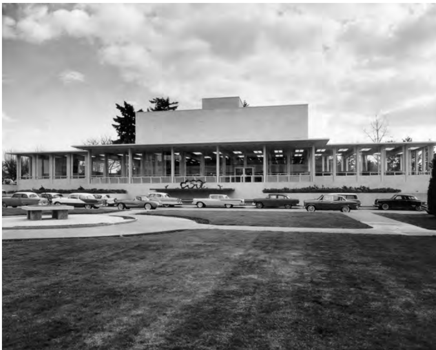
19. Ca 1959 view of the Washington State Library taken from near the O'Brien Building looking southeast. Source: Washington State Library
