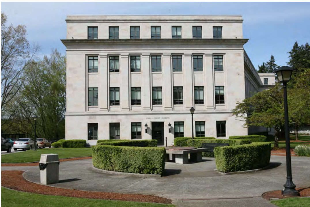
6 of 14. O'Brien Building, east facade fronting the Cherberg Building
